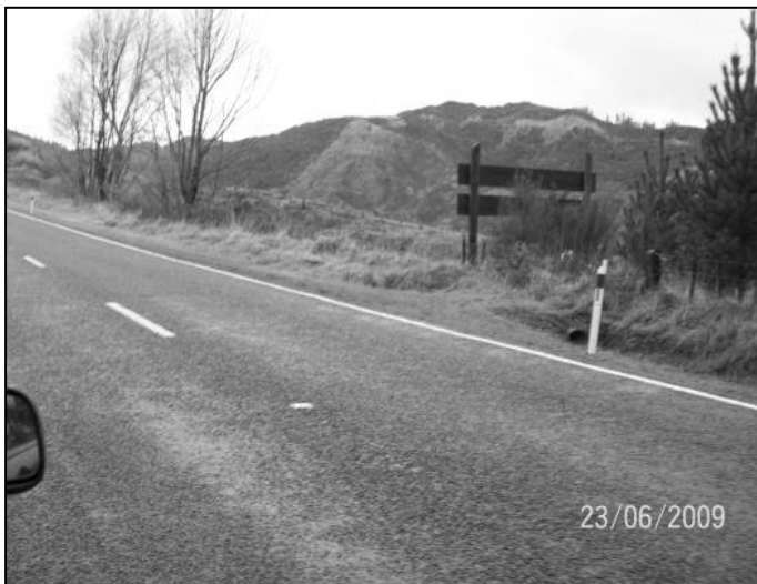
Figure 4.49 View of site C17, showing patchwork repairs
