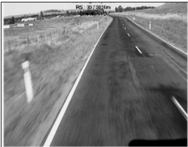
Figure 5.25 Typical view of site C1 (RP 33/3816 decreasing), showing repairs
