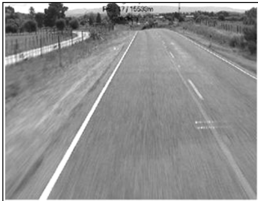
Figure 5.32 Inspection length in site C4: RP 15,533 increasing
