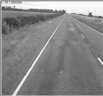
Figure 5.73 Typical view of site E4: RP 16,528 decreasing
