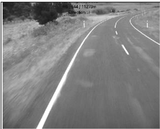
Figure 5.38 Inspection length in site C10: RP 544/11,273 increasing
