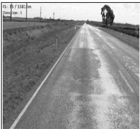
Figure 5.75 Inspection length in site E4: RP 15,817 increasing
