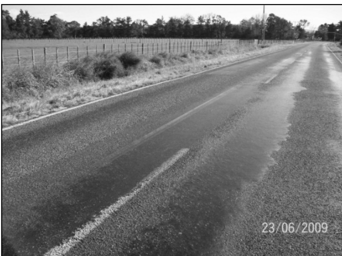
Figure 4.28 View of site C3, showing the high shoulders and an area of extensive flushing
