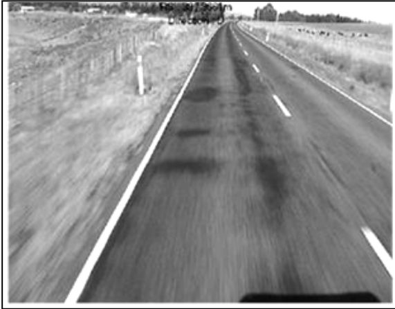
Figure 5.26 Typical view of site C1 (RP 33/3661 decreasing), showing extensive flushing
