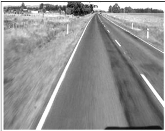
Figure .5.27 Inspection length of site C1: RP 33/3570 decreasing
