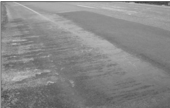
Figure 4.55 View of site D2, showing flushing and patchwork repairs
