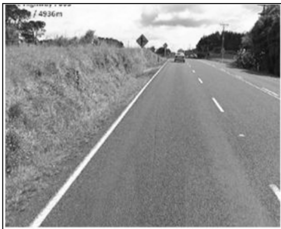
Figure 5.6 Inspection length 1 for site A1: RP 279/4936 decreasing
