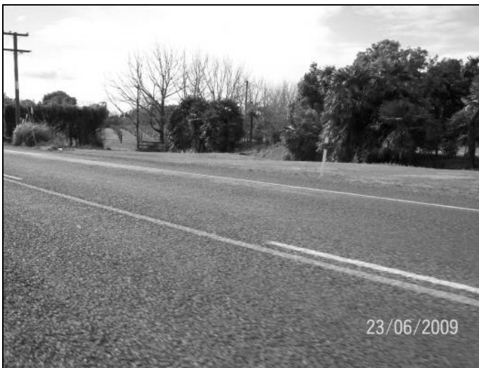
Figure 4.34 View of site C7, showing an area of good pavement condition
