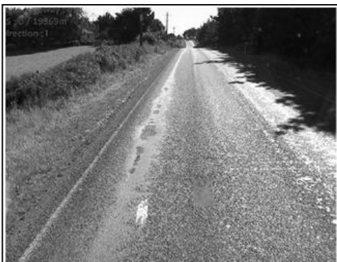
Figure 5.54 Another view of site D10 (RP 0/19,969 increasing), showing generally poor pavement condition
