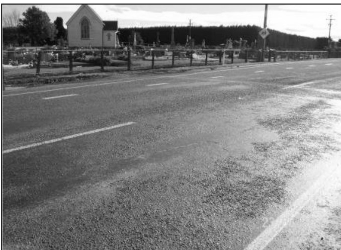
Figure 4.32 View of site C6, showing an area of considerable flushing
