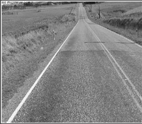
Figure 5.49 Another view of inspection length 1 from site D6: RP 8082
