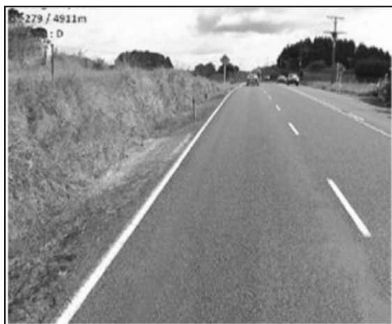
Figure 5.7 Inspection length 1 for site A1: RP 279/4908 increasing
