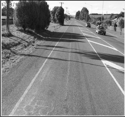
Figure 5.66 Another typical view of site E2 (RP 9452 increasing), showing flushed surface. condition
