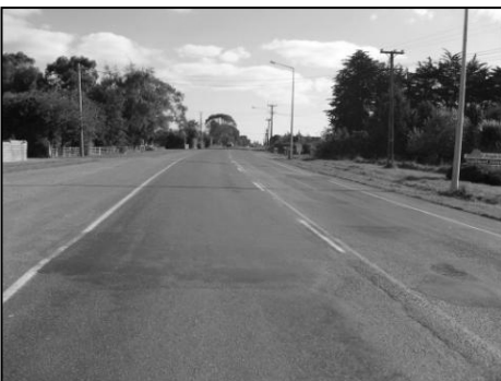
Figure 4.73 Alternative view of site D11, showing the depth of rutting
