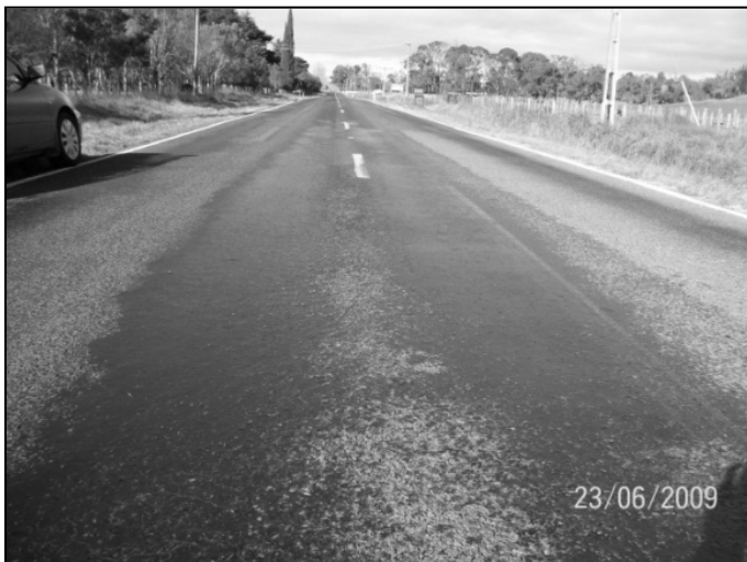
Figure 4.28 View of site C3, showing the high shoulders and an area of extensive flushing
