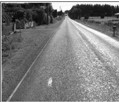
Figure 5.57 View of the inspection in site D10 (RP 0/19,747)
