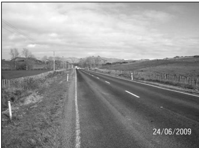
Figure 4.13 View of site B6, showing overall condition.
