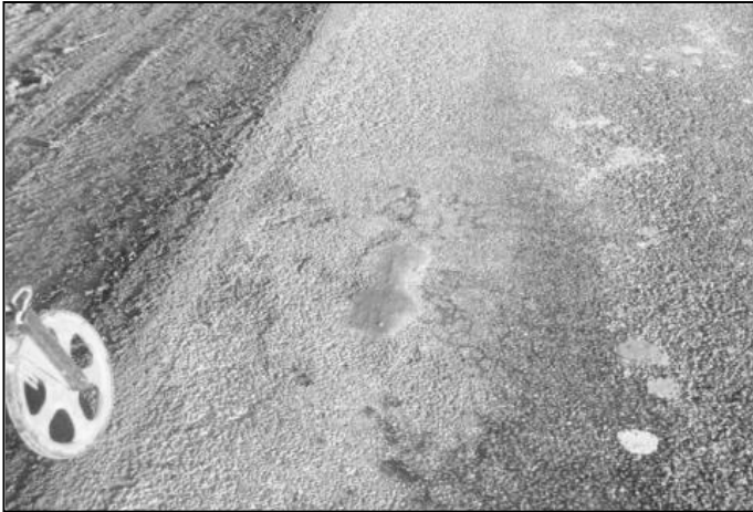
Figure 4.63 Second close-up view of site D6, showing flushing
