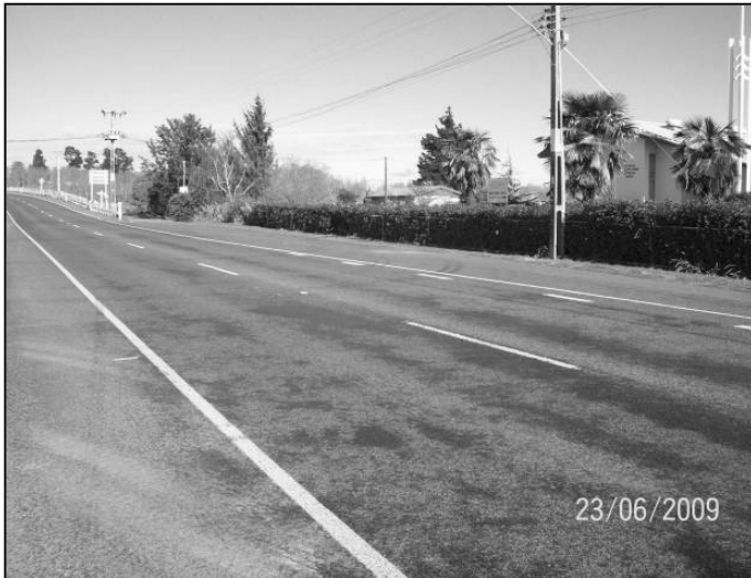
Figure 4.29 View of site C4, showing areas of flushing
