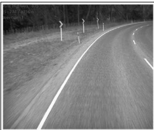
Figure 5.14 Typical inspection length distress in site B2 (RP 8736), showing evidence of corrugation
