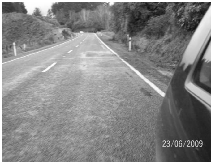
Figure 4.49 View of site C17, showing patchwork repairs
