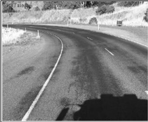
Figure 5.61 The inspection length in site E1: RP 118/15,531 increasing
