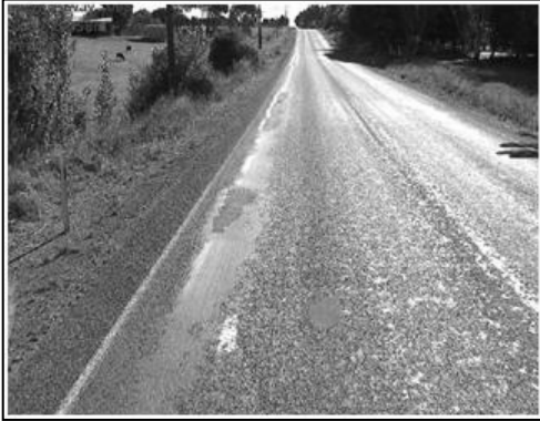
Figure 5.56 Typical section of pavement in site D10 (RP 0/20,234 increasing), showing extensive flushing
