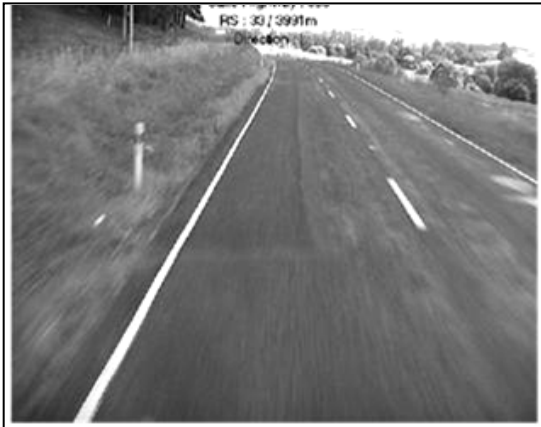
Figure 5.24 Typical view of site C1 (RP 3991 increasing), showing repairs and flushing
