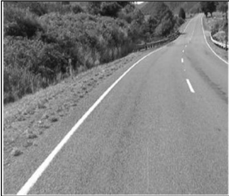
Figure 5.83 Another view of the inspection length in site F1: RP 225/4868 decreasing
