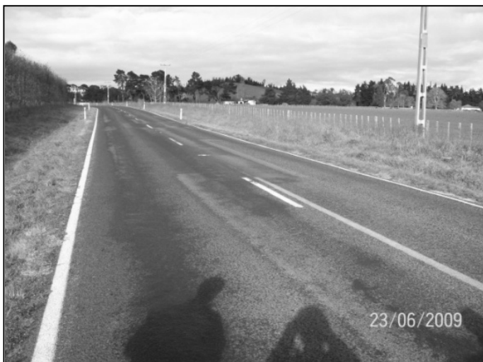
Figure 4.26 View of site C2, showing more patchwork repairs and extensive flushing
