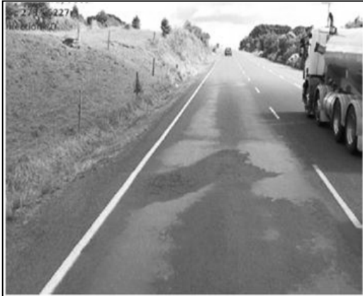
Figure 5.5 Another typical view of site A1: RP 279/5225 decreasing
