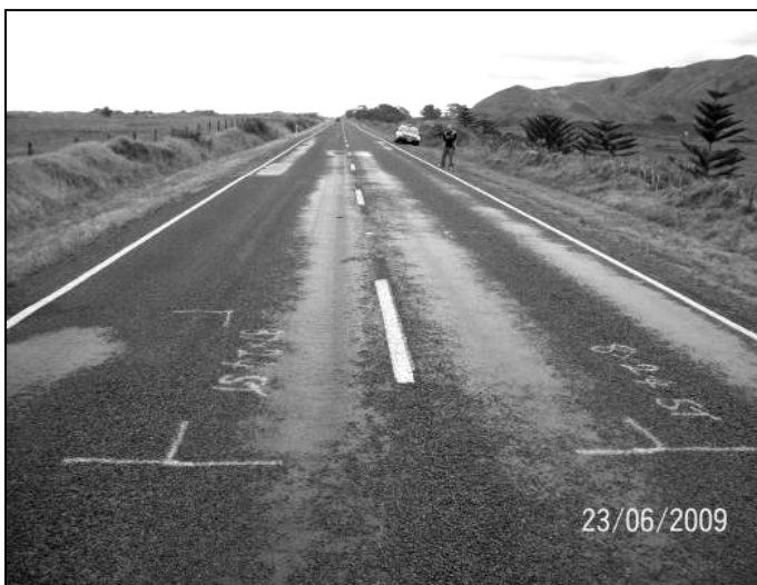
Figure 4.43 View of site C13, showing extensive flushing and potholing
