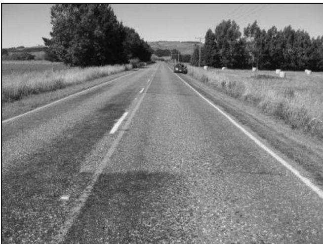
Figure 4.66 View of site D8, showing flushing and pavement repair
