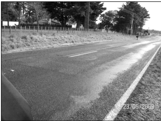
Figure 4.26 View of site C2, showing more patchwork repairs and extensive flushing
