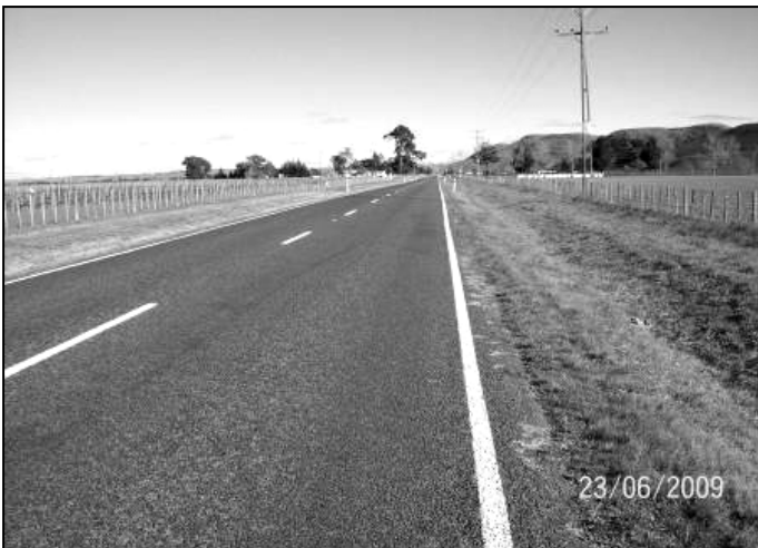
Figure 4.30 View of site C5, showing the reasonable condition of the pavement
