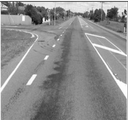
Figure 5.67 Inspection length 1 in site E2: RP 9375 increasing
