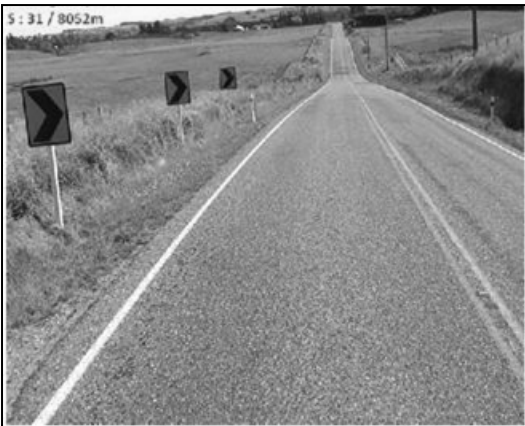
Figure 5.48 Inspection length 1 from site D6: RP 8052
