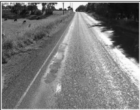
Figure 5.56 Typical section of pavement in site D10 (RP 0/20,234 increasing), showing extensive flushing
