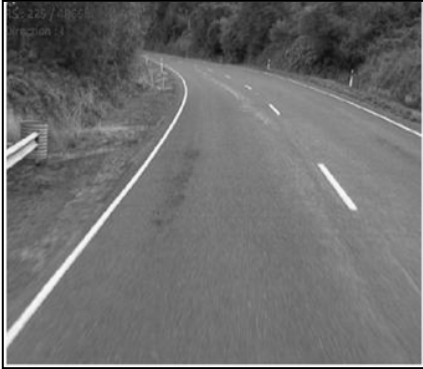
Figure 5.82 The inspection length in site F1: RP 225/4863 increasing
