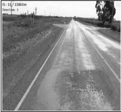
Figure 5.76 Another view of the inspection length in site E4: RP 15,867 increasing
