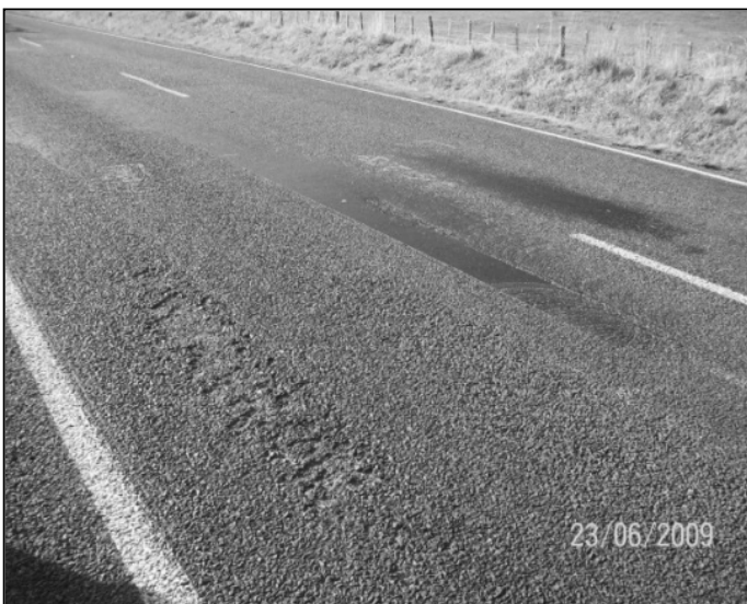
Figure 4.37 View of site C8, showing chip loss and flushing
