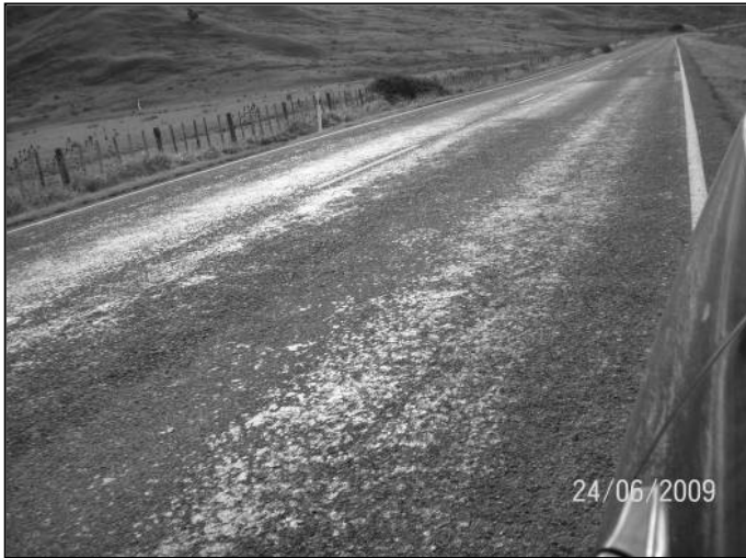
Figure 4.14 Alternative view of site B6, showing flushing
