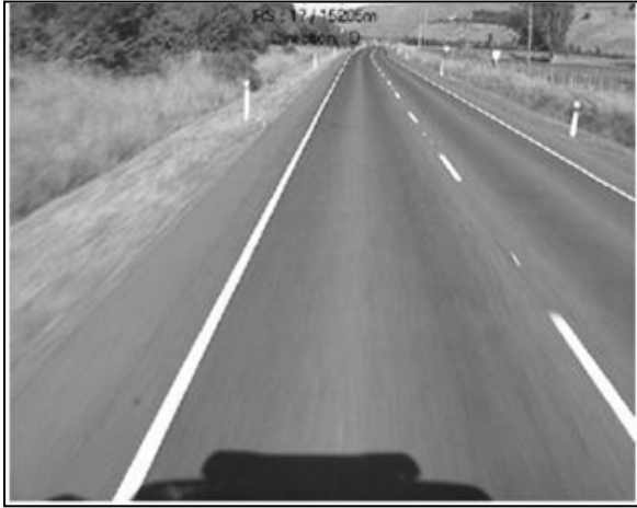
Figure 5.31 A typical section of road in site C4: RP 15,205 decreasing
