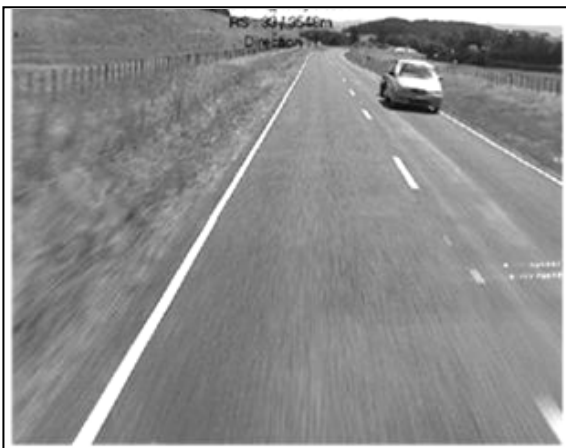
Figure 5.28 Inspection length of site C1: RP 33/3548 increasing
