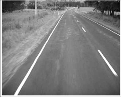
Figure 5.18 Another section of site B6: RP 3943 increasing
