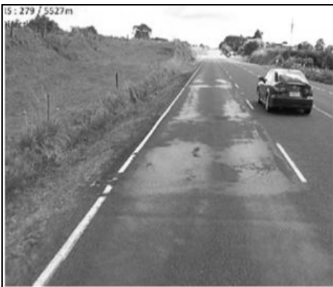
Figure 5.4 Typical view of site A1: RP 279/5525
