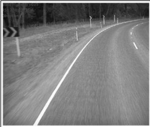
Figure 5.14 Typical inspection length distress in site B2 (RP 8736), showing evidence of corrugation
