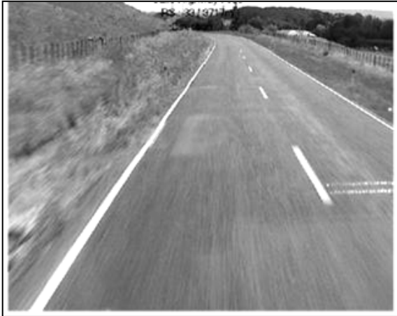
Figure 5.24 Typical view of site C1 (RP 3991 increasing), showing repairs and flushing
