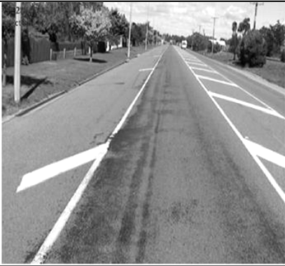
Figure 5.66 Another typical view of site E2 (RP 9452 increasing), showing flushed surface. condition
