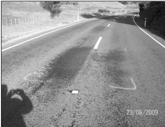
Figure 4.37 View of site C8, showing chip loss and flushing
