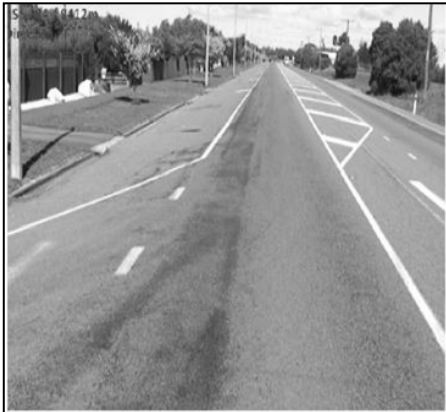
Figure 5.69 Inspection length 2 in site E2: RP 284/9410 increasing
