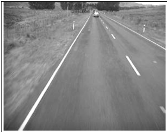
Figure 5.17 Another typical view of site B6 (RP 3763 increasing), showing evidence of pavement repairs
