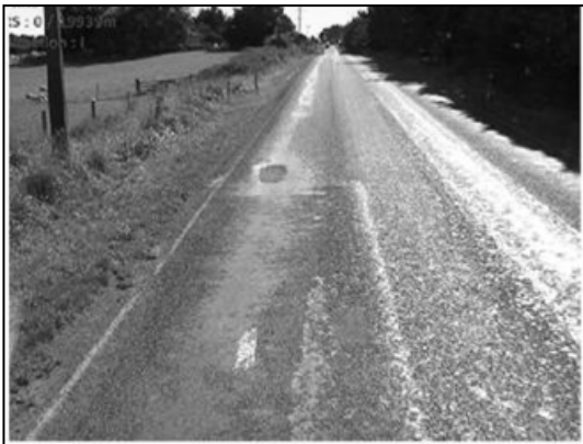
Figure 5.54 Another view of site D10 (RP 0/19,969 increasing), showing generally poor pavement condition
