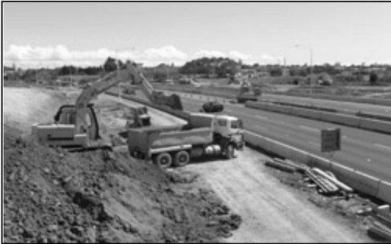
Figure 4.5 A Smith & Davies Ltd truck working at a road construction site
