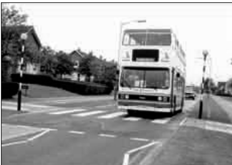
Figure 7.11 An S speed hump installed in the UK (DfT 2007c)
