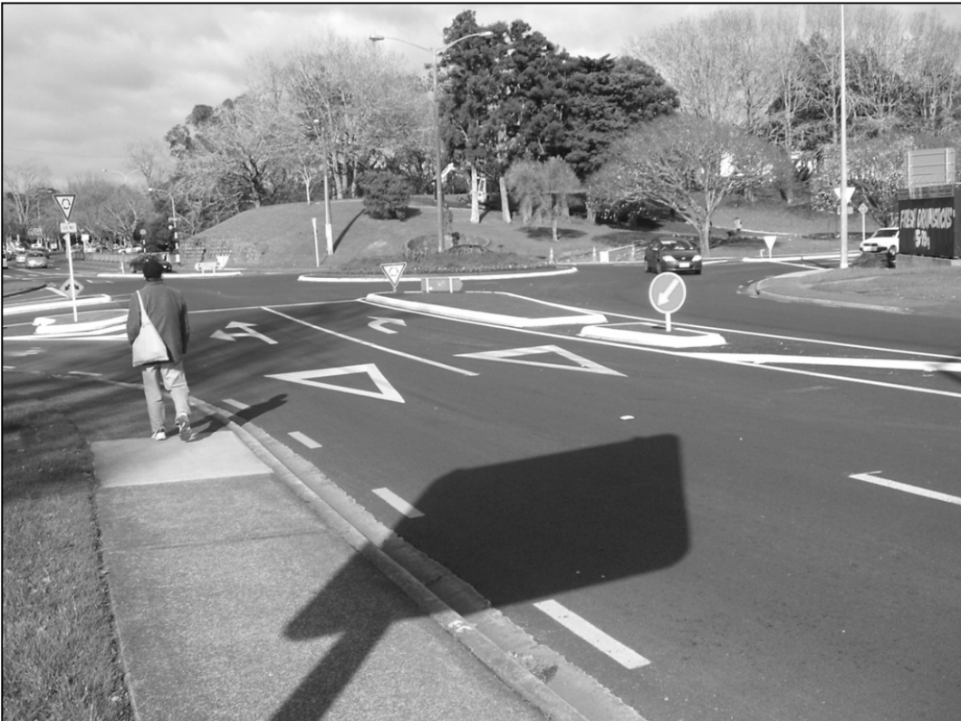
Figure 5.1 A pedestrian refuge island by the Sel Peacock Drive–Alderman Drive roundabout in Waitakere, Auckland
