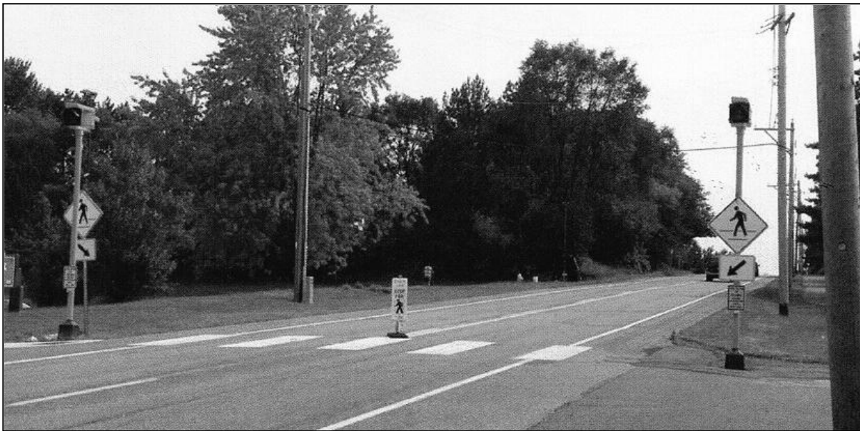
Figure 5.6 An example of an active warning sign with push-button call-up installed at a pedestrian crossing site in the US
