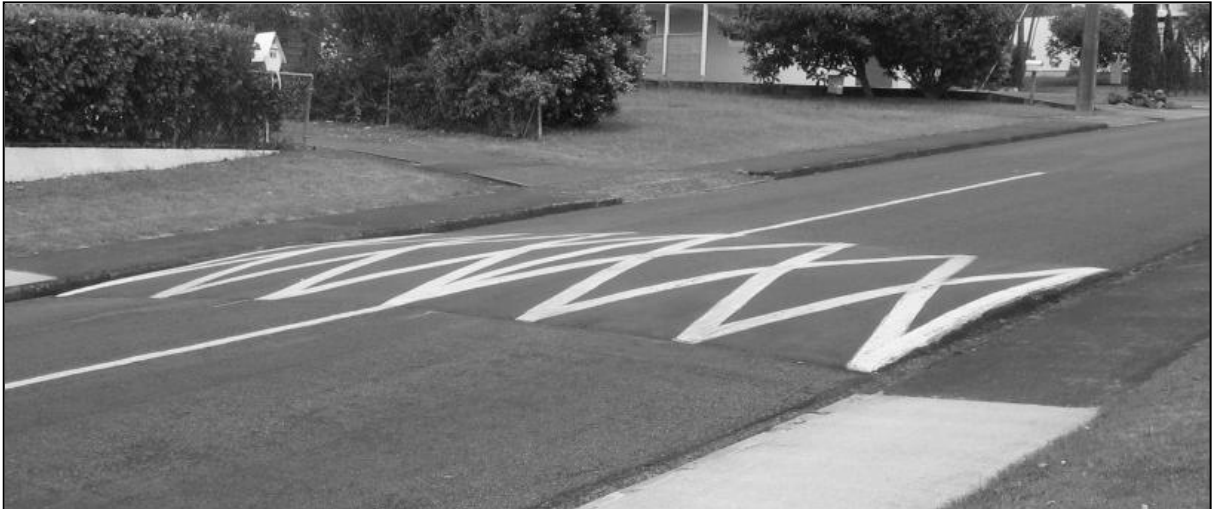
Figure H3 Photo of a MWP speed hump, as commonly installed in some New Zealand jurisdictions
