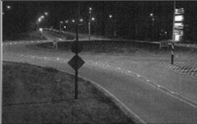
Figure 8.25 Alternative view of the lighting arrangements on the mountable lane dividers at turbo-roundabouts (CROW 2008)
