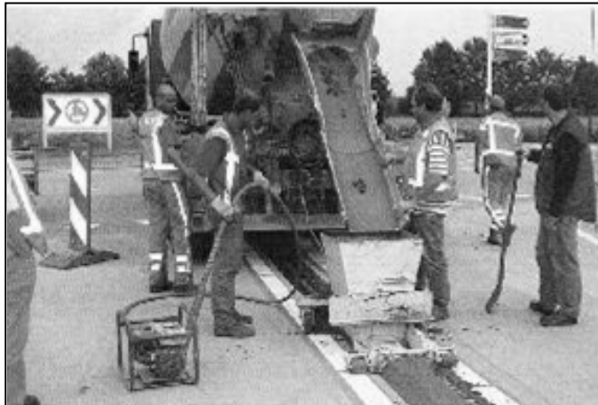
Figure 8.23 In situ construction of the mountable lane dividers: shaping the dividers (CROW 2008)
