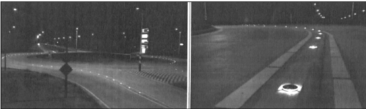
Figure I29 Example of road lighting (LED) to improve visibility of the lane dividers
