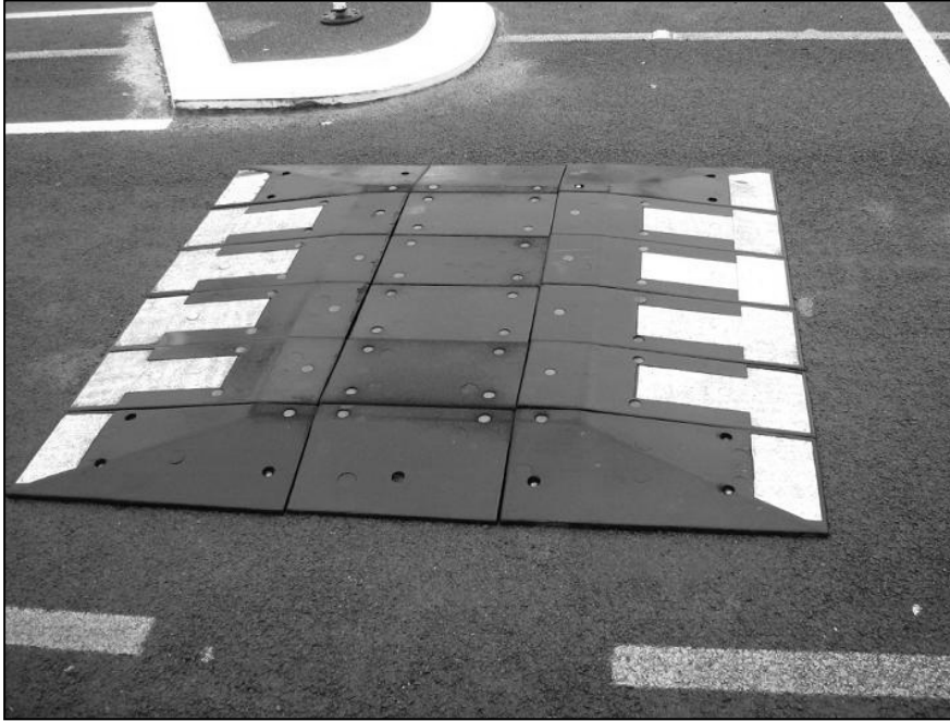
Figure 7.13 Photo of a 1.8m wide speed cushion installed on Pooks Road in Waitakere City (this 75mm high example is made of recycled rubber, which means it can be installed quickly and with minimum traffic management)
