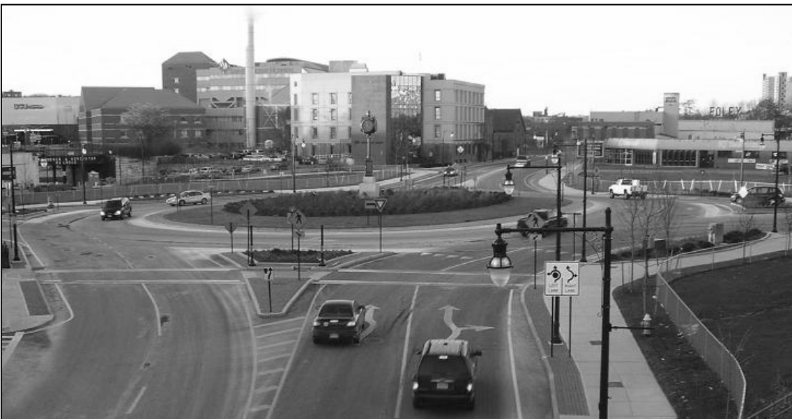
Figure 5.3 Photo of a roundabout in the US with zebra crossing type facilities (where drivers are supposed to yield to pedestrians) with associated signage* and slightly raised red paver treatments
