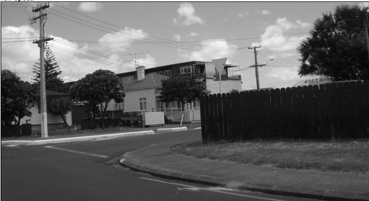
Figure D2 The driver's perspective, taken 10m back from the limit line of the Church Street–Avenue Road roundabout approach, demonstrating how the boundary fence restricts sightlines, encouraging drivers to reduce their speed
