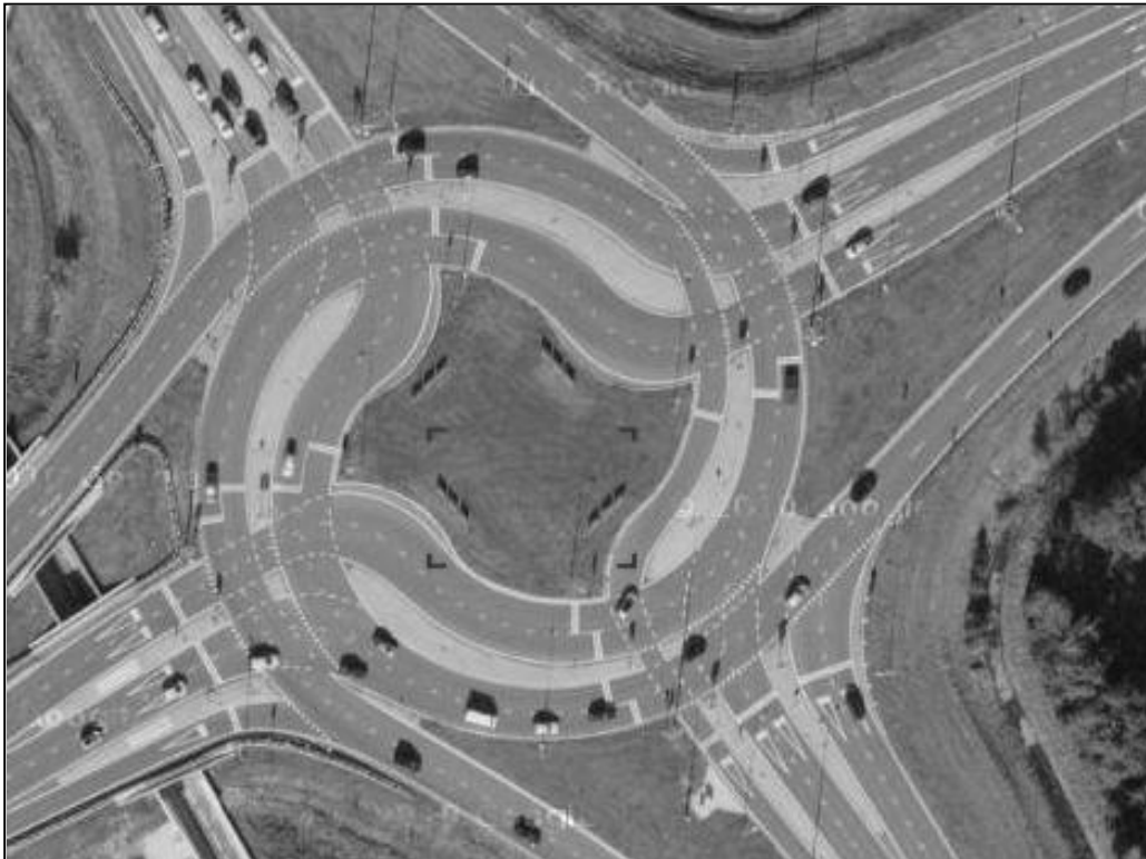
Figure 8.42 Aerial view of the Doenkadeplein signalised turbo-roundabout in The Netherlands at the intersection of roads N209 and N471 (the outside diameter of the roundabout is approximately 110m; photo courtesy of Google Maps)
