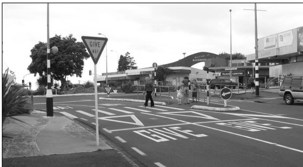
Figure 6.19 Photo of the staggered pedestrian zebra crossing on the Kinross Street approach to the Blockhouse Bay roundabout
