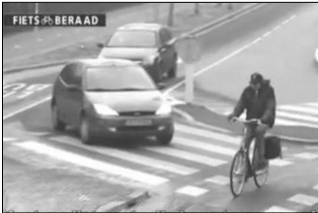
Figure 8.32 Cyclist using the at-grade cyclist priority crossings at a turbo-roundabout, with vehicles yielding (CROW 2008)
