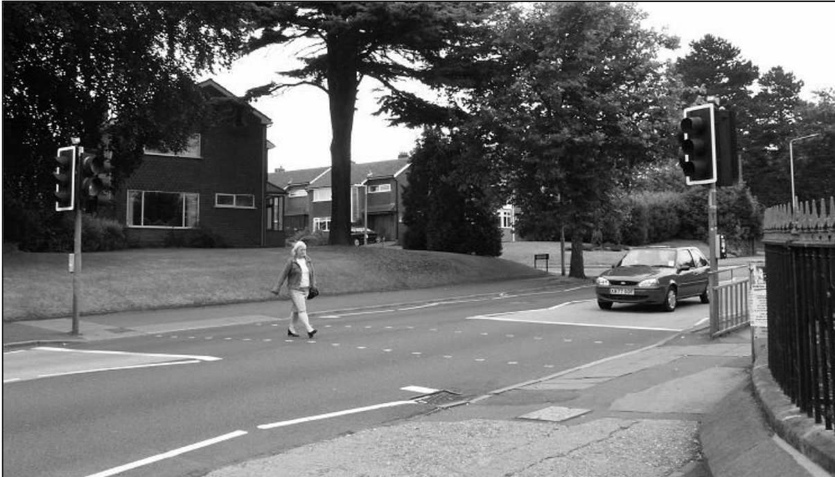
Figure 5.13 A British Pelican crossing, which is a full-time signal arrangement using three-aspect displays facing drivers. This particular example is fitted with nearside displays for pedestrians similar to those used by Puffin crossings (photo from Dudley Metropolitan Borough Council)
