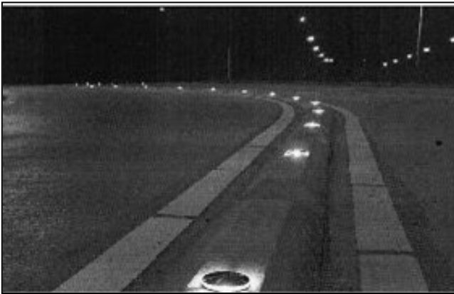
Figure 8.26 Photo of the damage that can occur if lane dividers are glued onto the roadway instead of cast in situ (CROW 2008)
