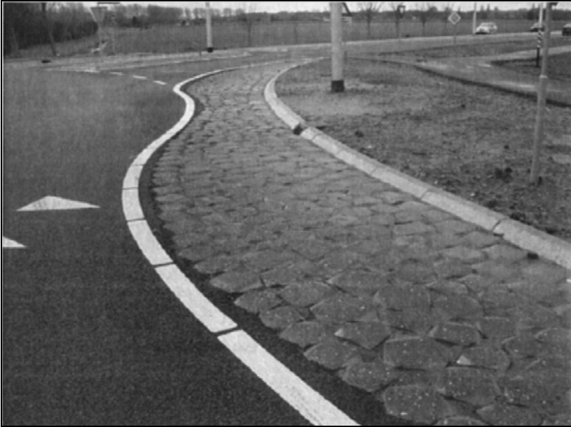
Figure I31 Rumble area for articulated vehicles
