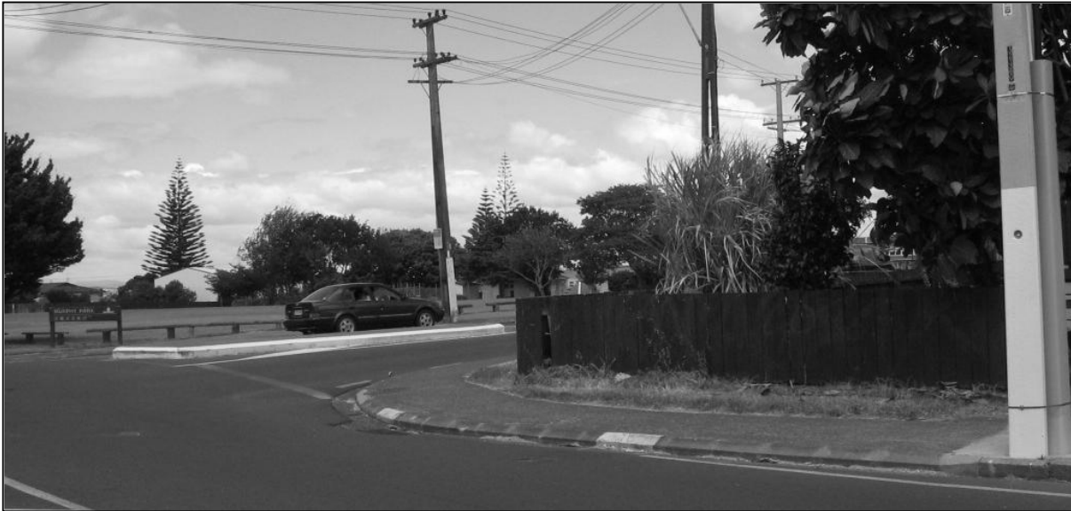
Figure 4.12 View taken on approach B at a point 10 m from the roundabout limit line, showing the corner boundary fence which severely restricts visibility of vehicles coming from approach A to the right
