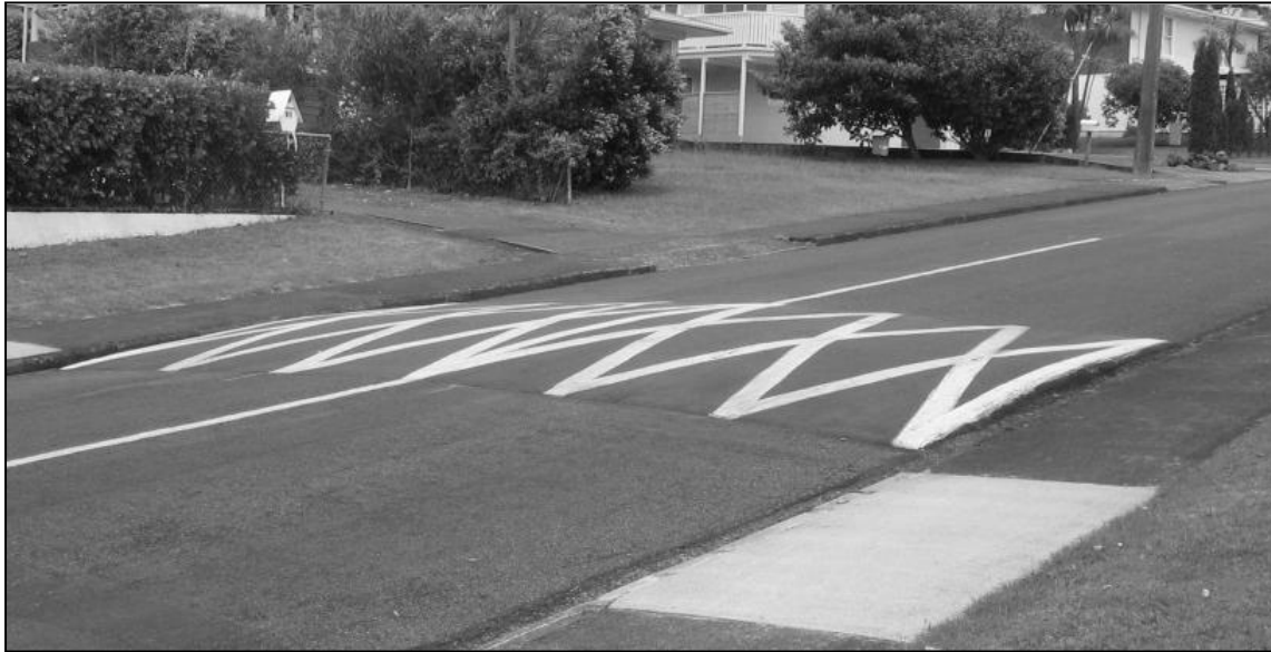
Figure 7.4 A MWP speed hump in a local street, as commonly installed by many New Zealand jurisdictions
