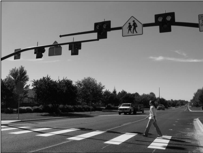
Figure 5.14 Hawk hybrid pedestrian signal in the United States (photo from Ada County Highways Department)
