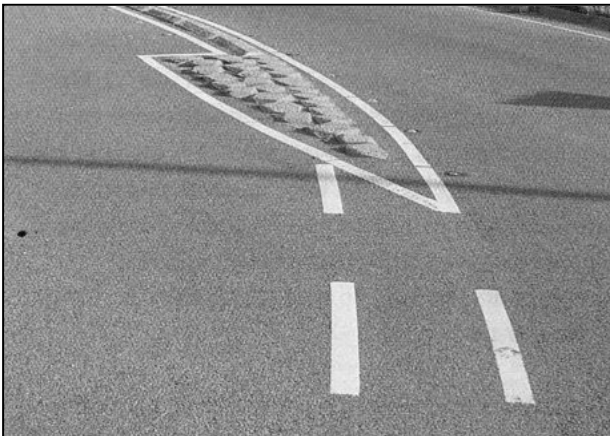
Figure 8.20 Pointed end treatment applied to the lane dividers (CROW 2008)
