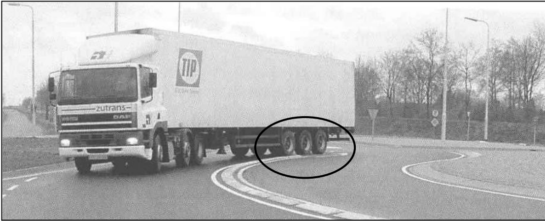
Figure 8.45 Photo showing a semi-trailer in The Netherlands negotiating a turbo-roundabout (CROW 2008). Note the mountable lane dividers between traffic lanes which the rear tyres are driving over (circled)
