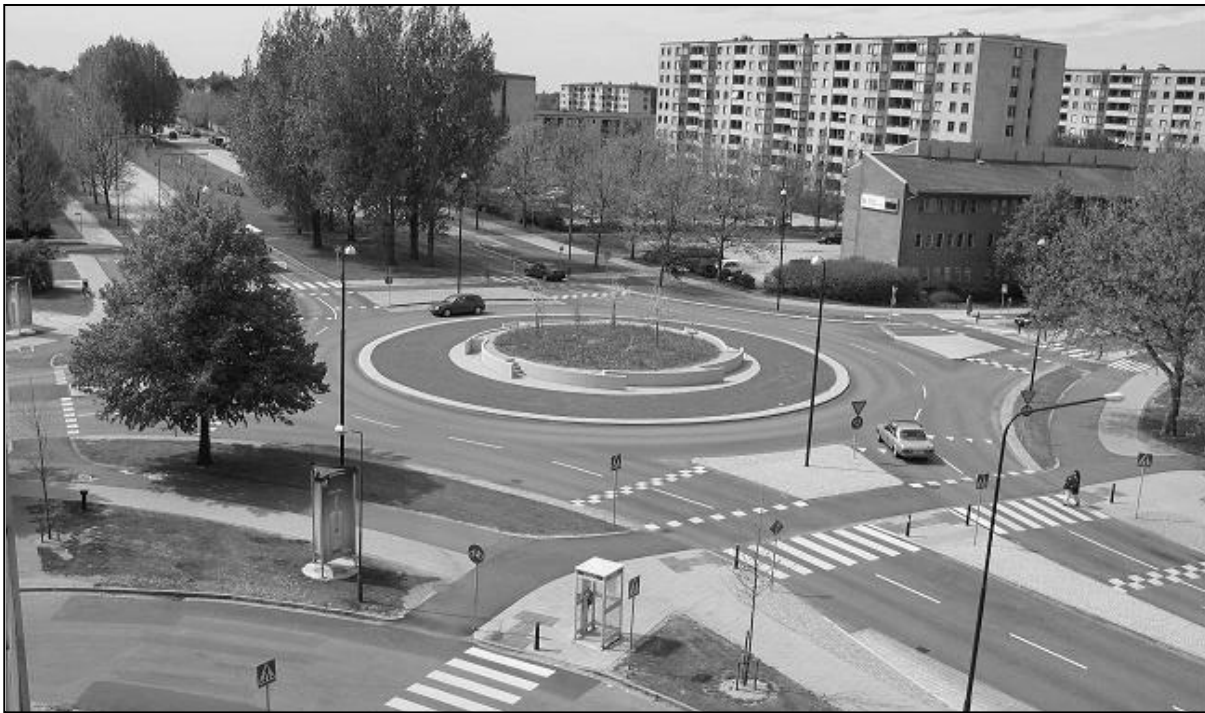
Figure H1 The Lorensborgsgatan–Stadiongatan roundabout in Malmö, Sweden (left-hand drive) which uses 100mm-high raised platforms on each entry and exit arm to facilitate pedestrian and cycle path crossing points around the perimeter of the roundabout (photo provided by Transport Department, City of Malmö)
