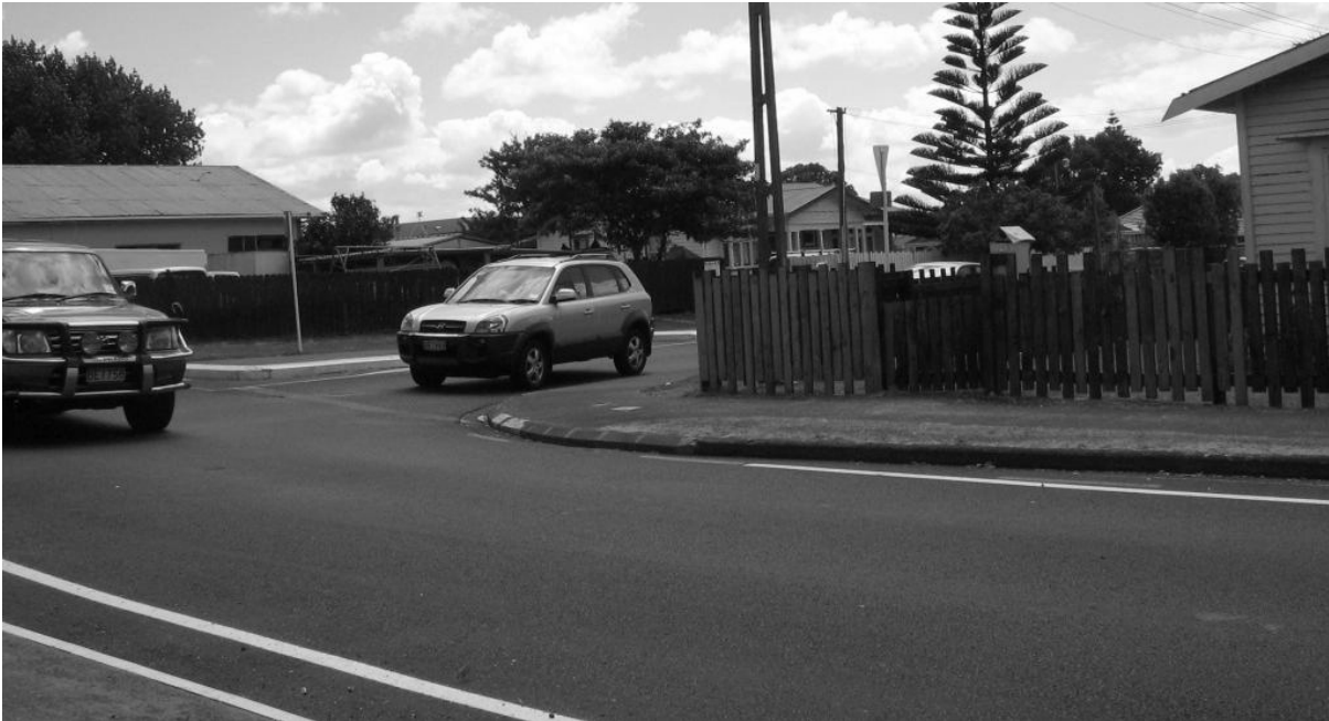
Figure 4.14 View taken on approach D at a point 10m from the roundabout limit line, showing the corner boundary fence which severely restricts visibility of opposing vehicles coming from approach C to the right
