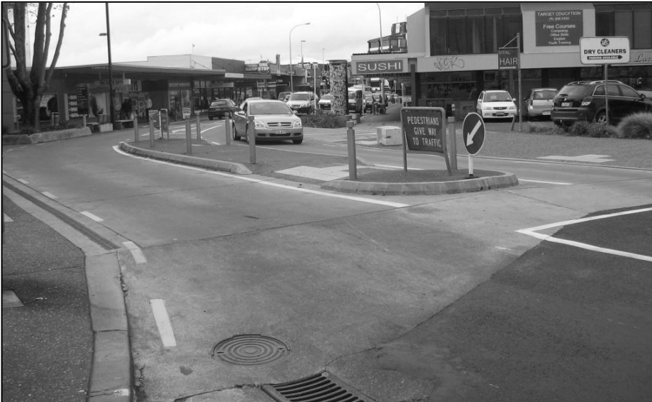
Figure 7.3 A platform arrangement at an informal crossing point in Henderson town centre, Waitakere
