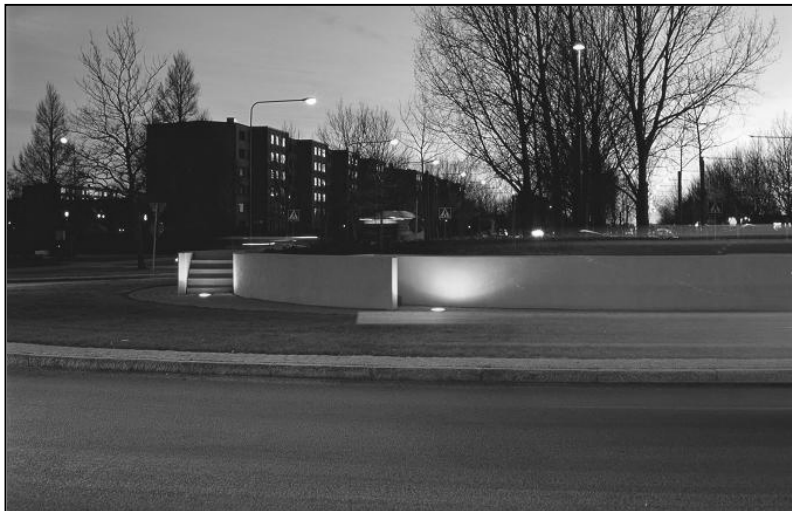
Figure 7.33 Lighting arrangements on the central island of the Lorensborgsgatan–Stadiongatan roundabout, demonstrating how aesthetics and amenity can be combined
