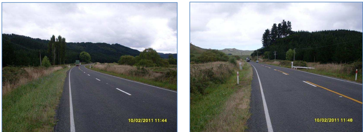
Figure 4.8 The Awaho Culvert project
