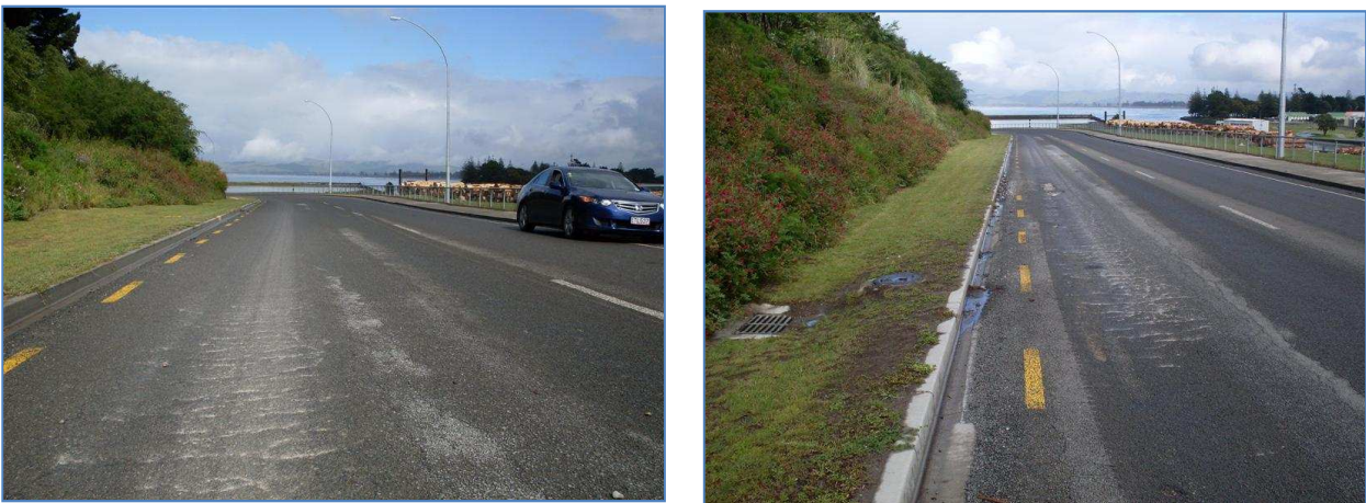
Figure 4.9 The Hirini Street project
