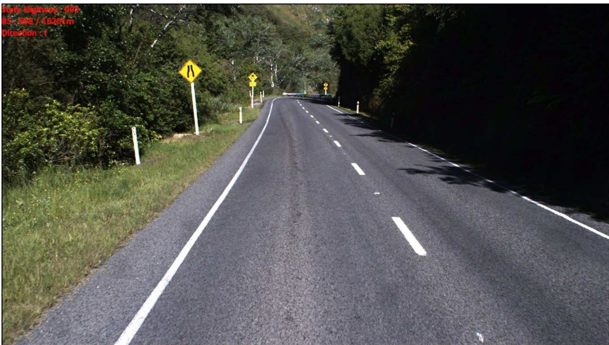
Figure 5.22 Site 11: SH 2 RS 608 15.703 – 17.130 – constructed in 1997
