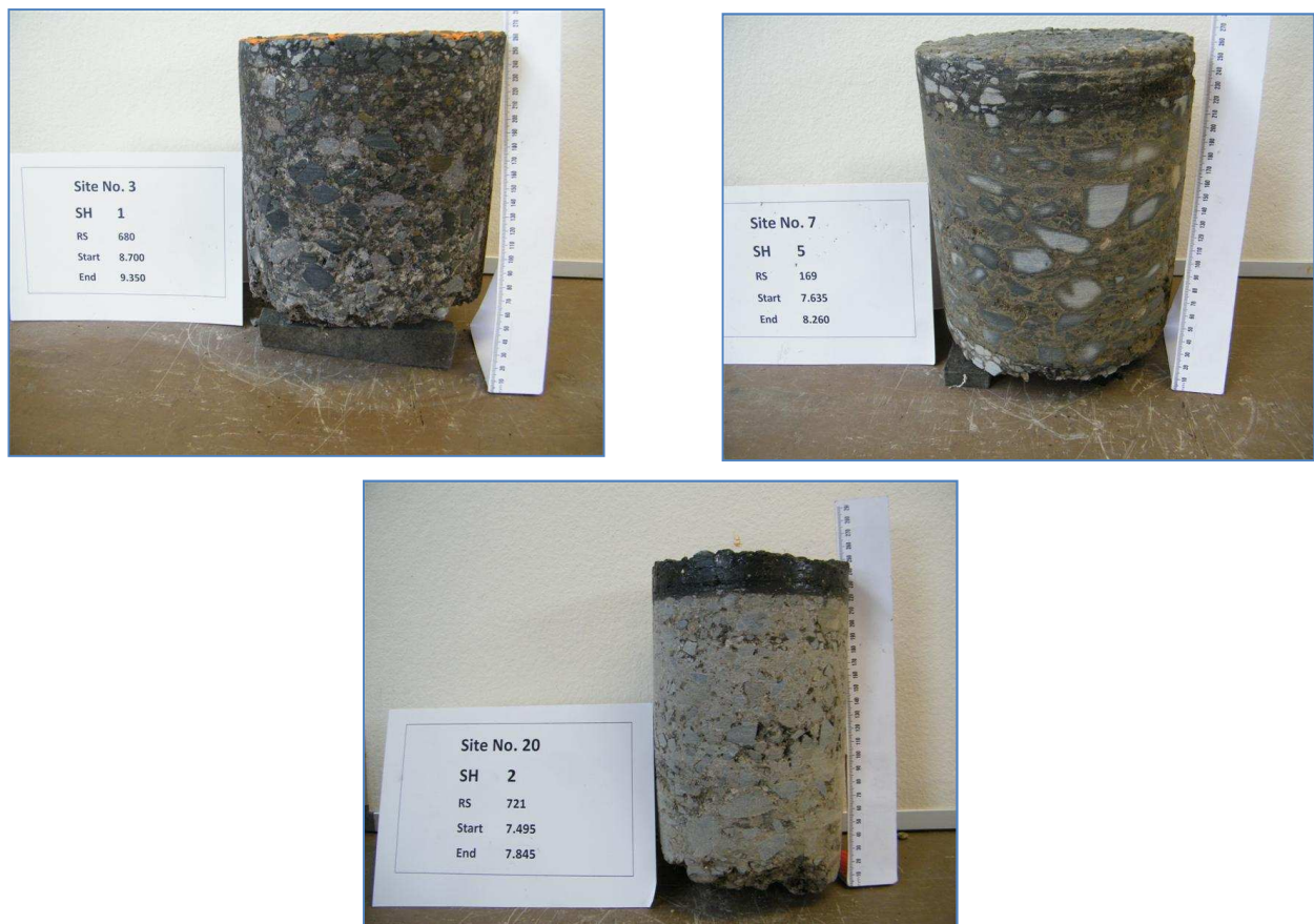
Figure 4.3 Photographs of representative pavement cores retrieved from the field
