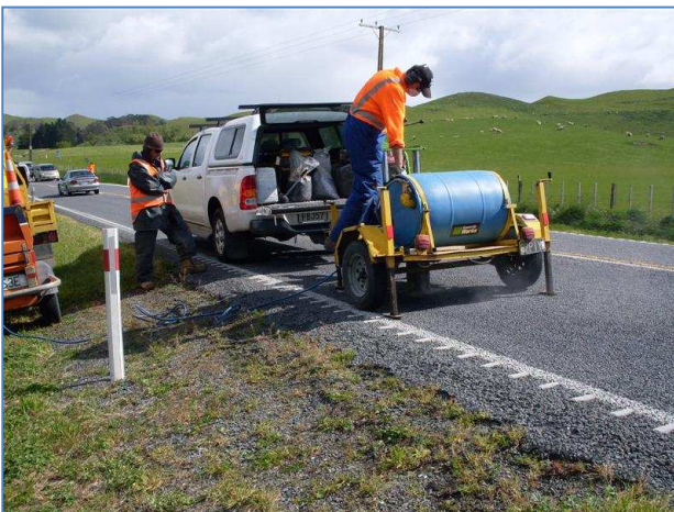
Figure 4.1 Photographs showing pavement core recovery technique
