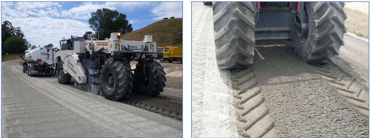
Figure 1.1 Stabilisation of near-surface granular layers
