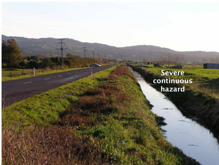
Figure A6.2 Shoulder environment without unsealed shoulder traversable slope limited by severe continuous hazard
