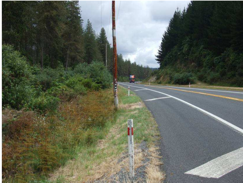
Figure 2.7 Example of roadside shoulder environment with point hazards
