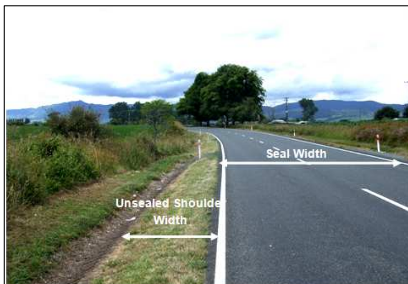
Figure 2.5 Seal width and unsealed shoulder width
