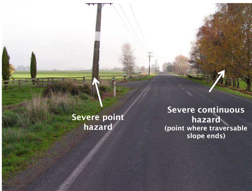
Figure A6.4 Example of severe point hazard data collection
