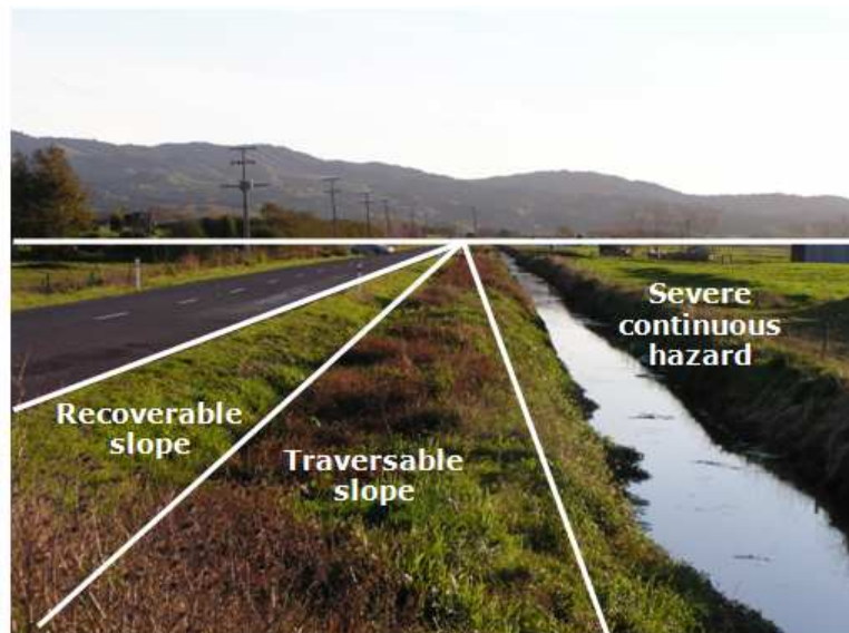
Figure 2.6 Example of roadside shoulder environment showing recoverable slope and traversable slope
