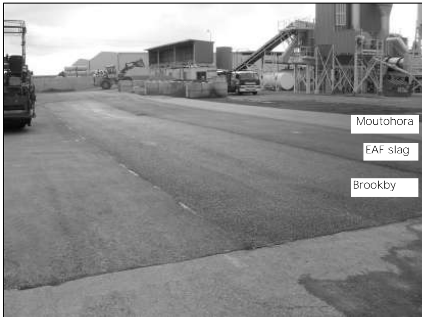
Figure 5.12 Comparative texture of the three sections laid in Auckland
