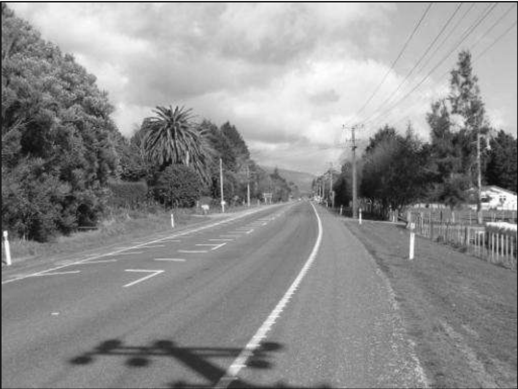
Figure A2 Arapaepae Road (SH57), 410m from the intersection after installation of the transverse markings
