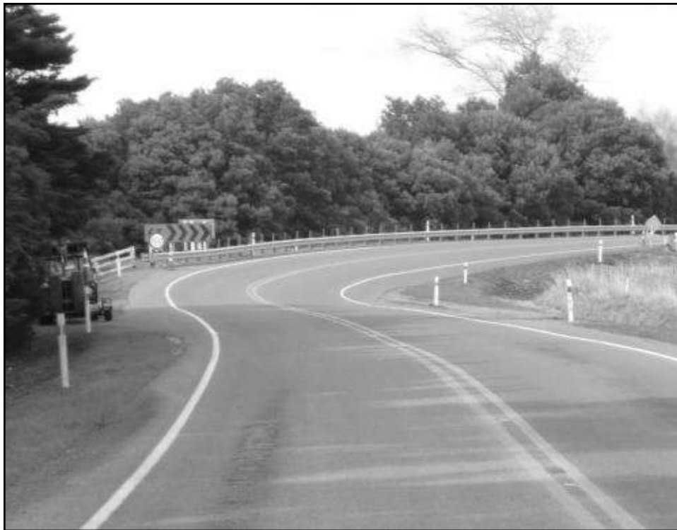
Figure B5 Eastbound Waihenga Bridge approach (SH53), 50m from the horizontal curve
