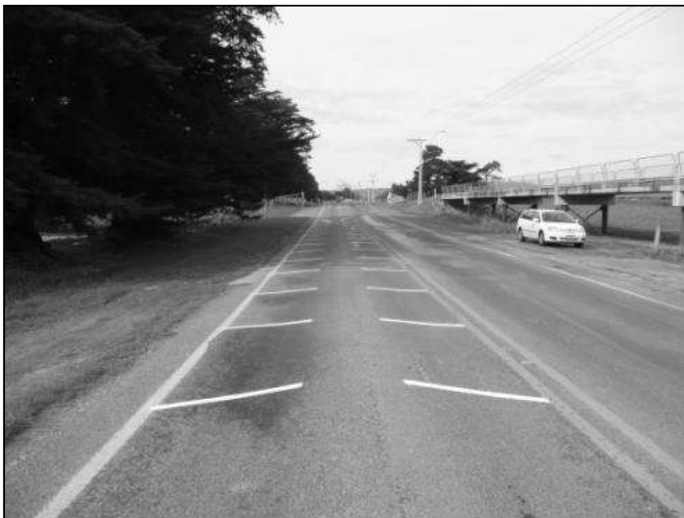
Figure B2 Eastbound Waihenga Bridge approach (SH53), 410m from the horizontal curve after installation of the transverse markings
