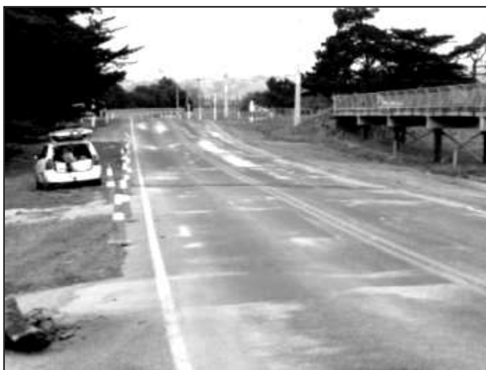
Figure 3.9 Cones observed at the start of the SH53 trial site
