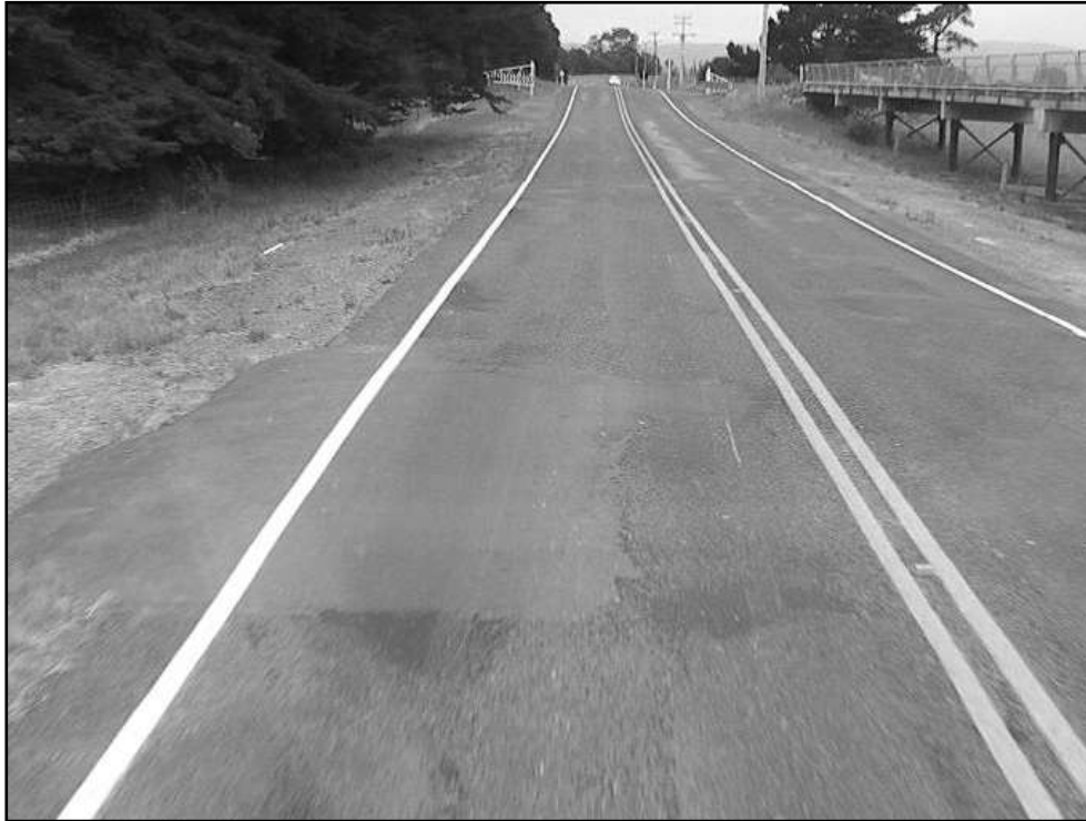
Figure B2 Eastbound Waihenga Bridge approach (SH53), 410m from the horizontal curve after installation of the transverse markings
