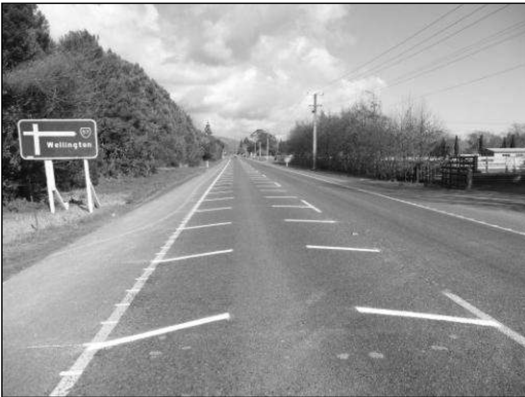
Figure A4 Arapaepae Road (SH57), 260m from intersection after installation of the transverse markings
