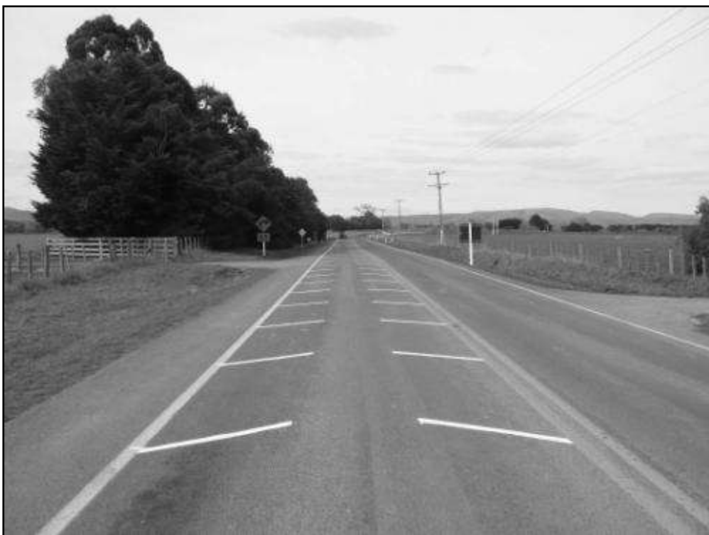
Figure B4 Eastbound Waihenga Bridge approach (SH53), 260m from the horizontal curve after installation of the transverse markings
