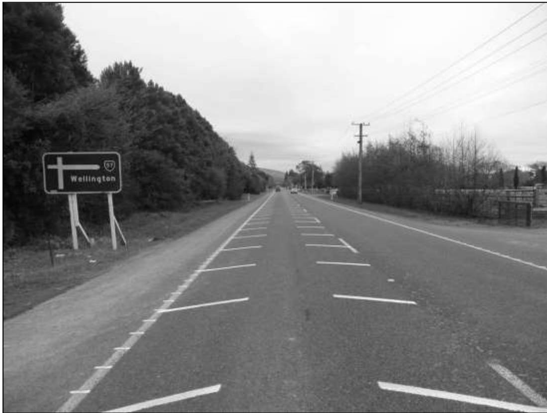
Figure 1.1 An example of transverse road markings
