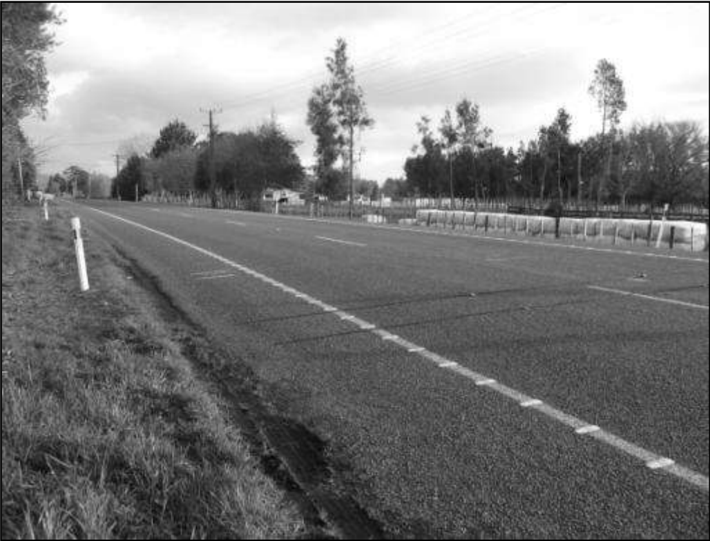
Figure A1 Arapaepae Road (SH57), 410m from the intersection prior to transverse marking installation
