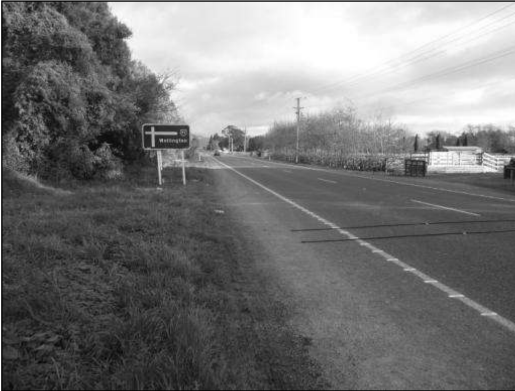
Figure A3 Arapaepae Road (SH57), 260m from the intersection prior to transverse marking installation
