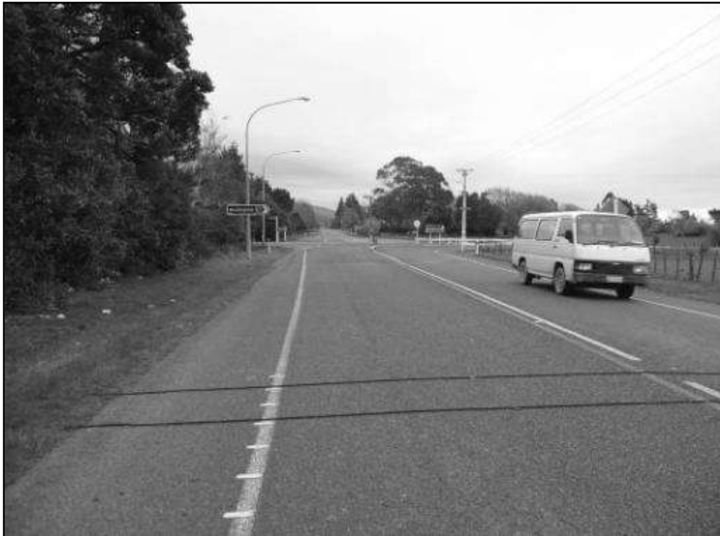
Figure A5 Arapaepae Road (SH57), 50m from the intersection
