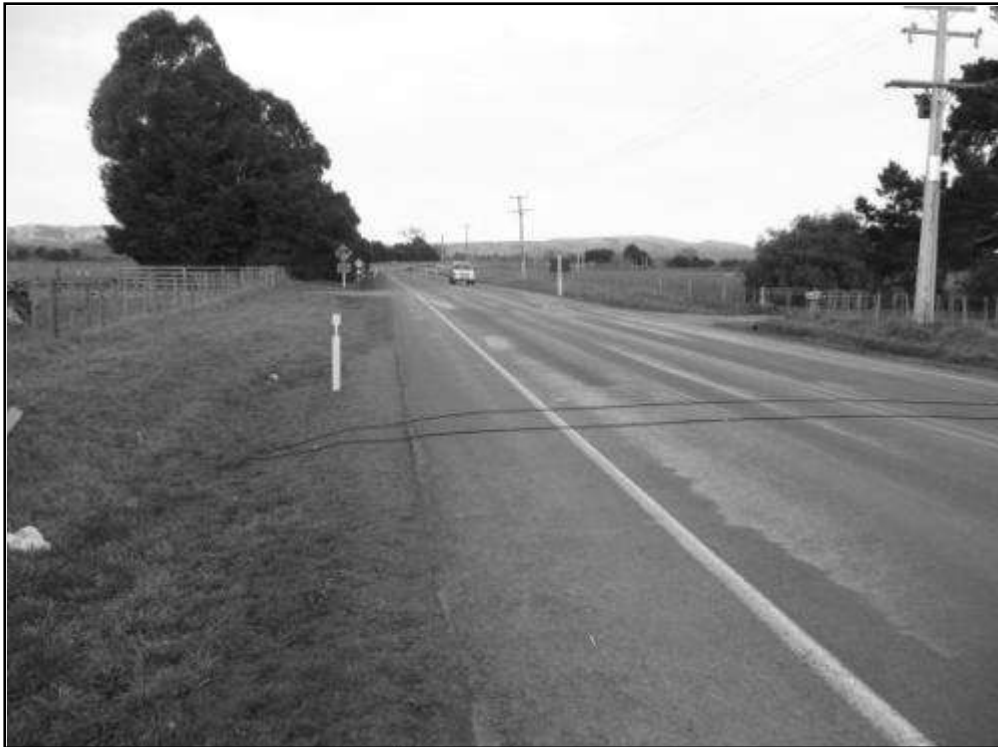
Figure B4 Eastbound Waihenga Bridge approach (SH53), 260m from the horizontal curve after installation of the transverse markings
