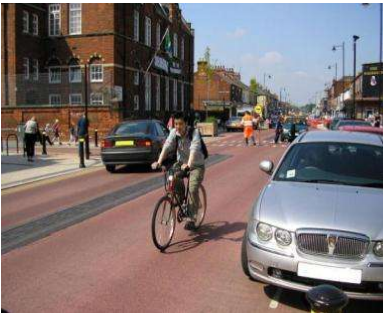
Figure 4.17 The consideration that is increasingly being given to a wide range of road users when designing arterial roads through town centres could be extended to those parts of arterial roads that pass by schools (Photo: Phil Jones)
