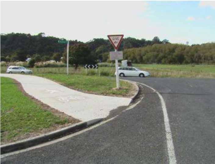
Figure 4.2 A shared pathway in a rural environment (Waitoki, Rodney District) has created walking and cycling opportunities for primary school students
