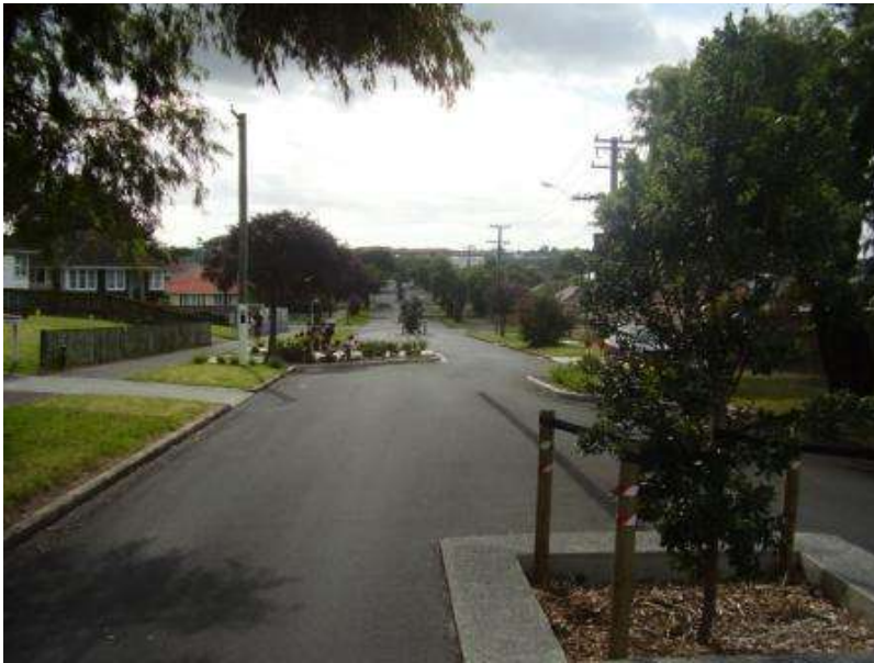
Figure 4.20 Road layout changes resulted in a mean speed of approximately 30km/hr on local streets in the Point England SER study, highlighting the importance of engineering in creating safe speeds
