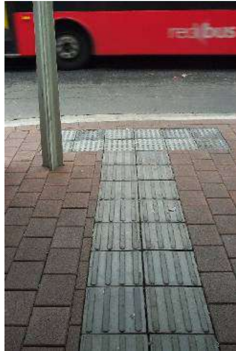
Directional and warning indicators installed at a bus stop
