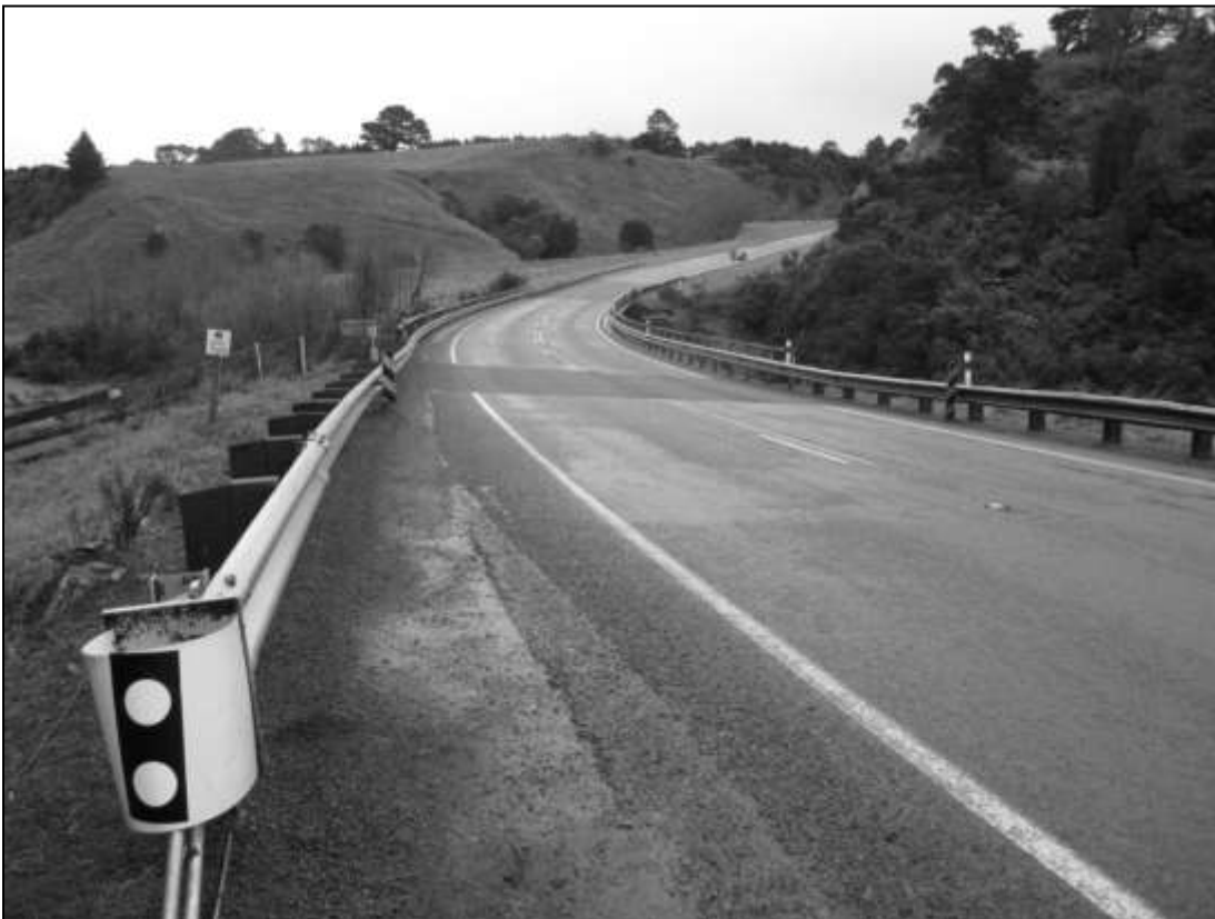
Figure 3.4 Mangatewai-iti bridge looking north (decreasing direction)
