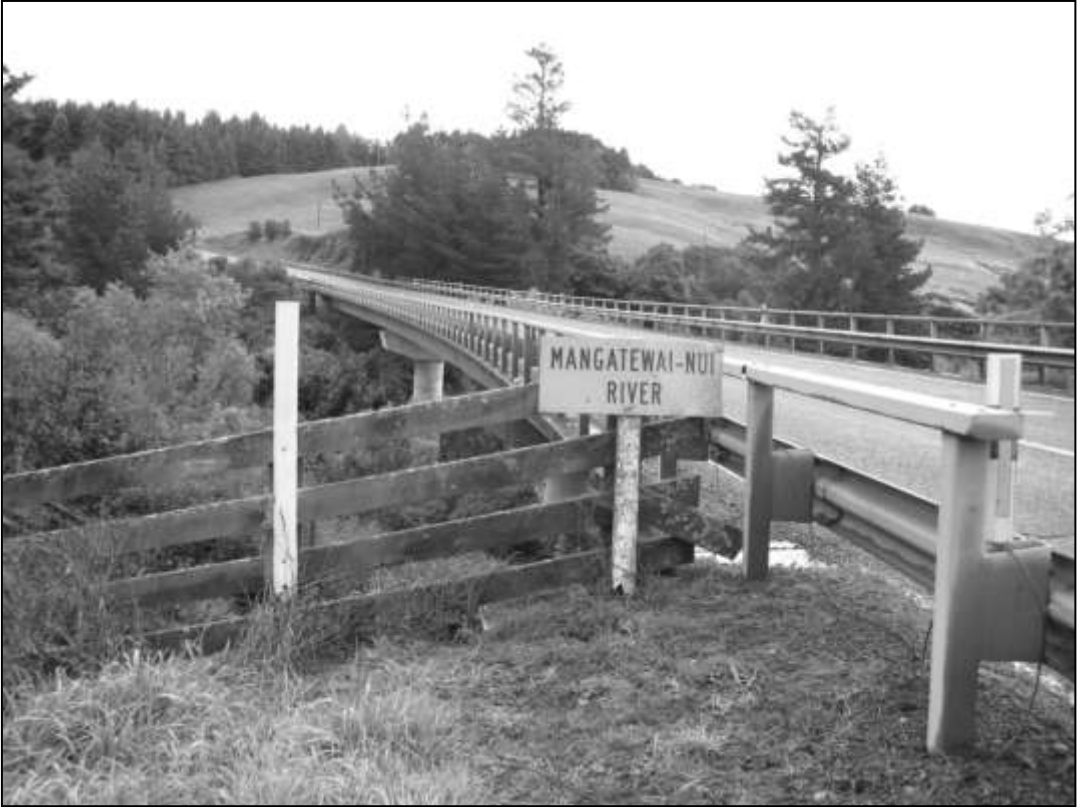
Figure 3.5 Mangatewai-nui bridge looking north (decreasing direction)
