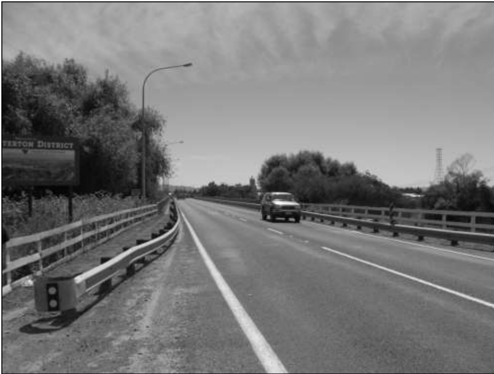
Figure 3.3 Waingawa bridge looking north (decreasing direction)
