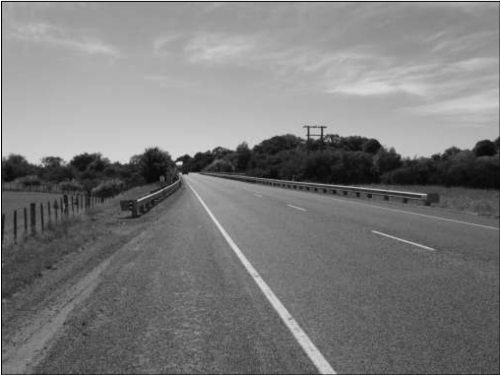
Figure 3.1 Tauherenikau bridge looking north (decreasing direction)
