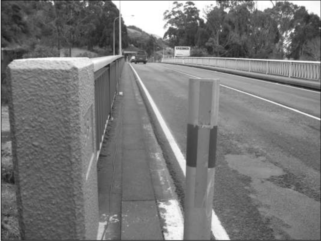
Figure 3.6 Waikanae bridge looking south (increasing direction)
