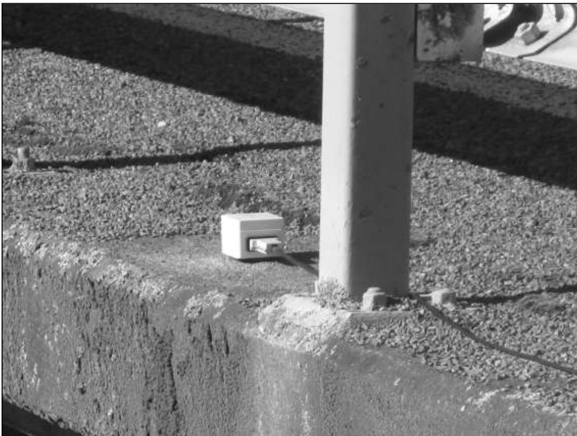
Figure 5.1 Syflex™ triaxial accelerometer on bridge edge (centre of first span)
