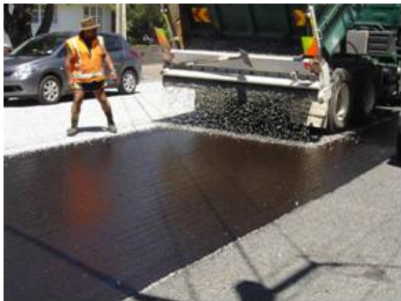
Figure 5.2 Application of the grade 3 chip
