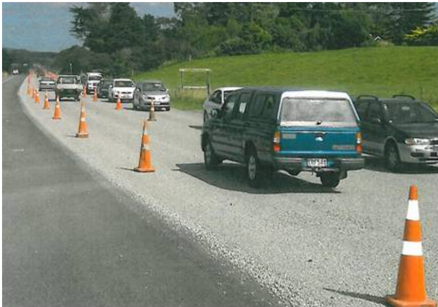
Figure 6.11 Photo of the active traffic control during the resealing
