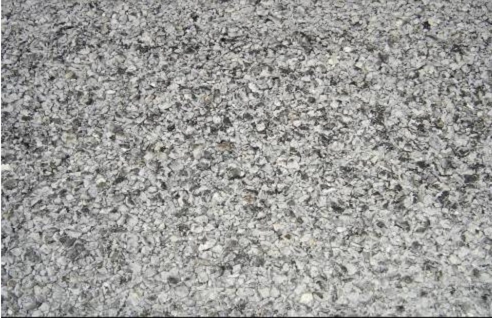
Figure 5.6 Photo showing the polymer modified emulsion being tracked over the seal surface
