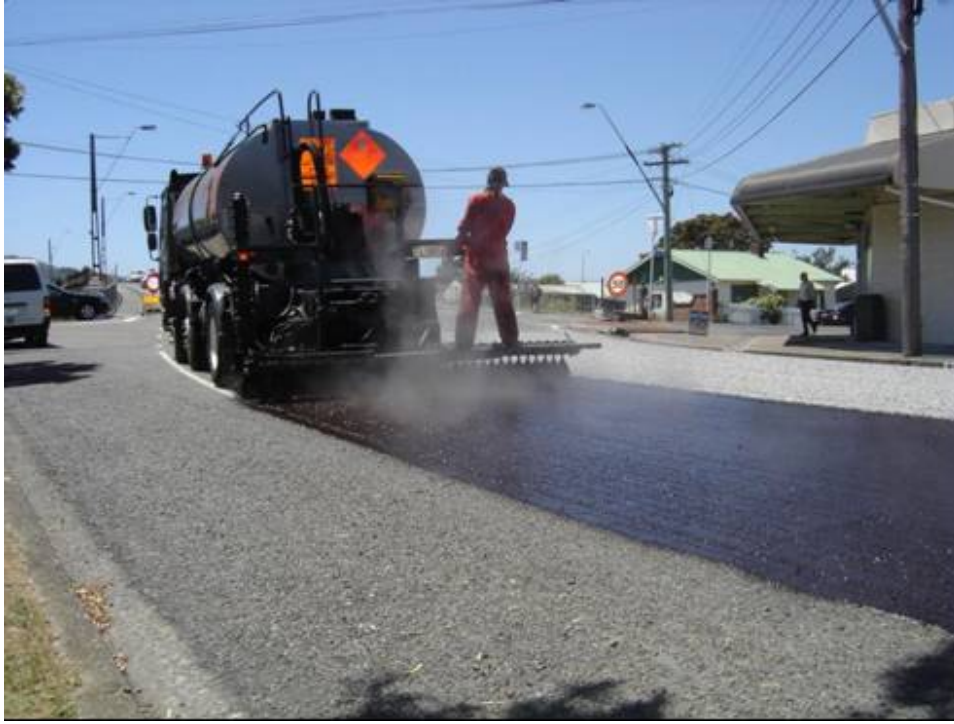
Figure 5.1 Spraying of the polymer modified emulsion in Cuba Street
