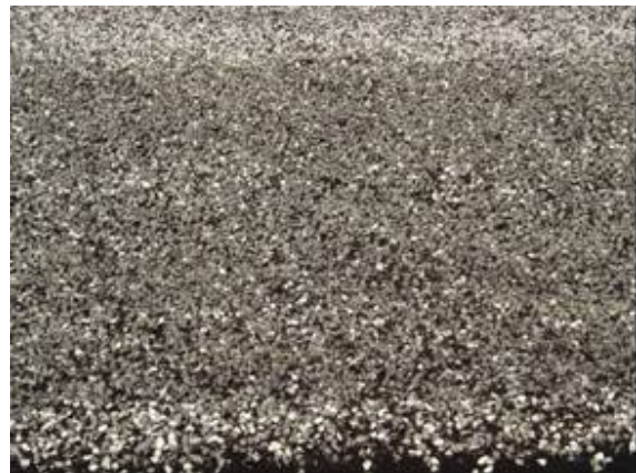
Figure 5.3 Open 'windows' ready for the small grade 5 chip
