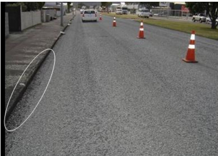
Figure 5.7 Photo illustrating the excess chip flicked to the outer of the wheel tracks
