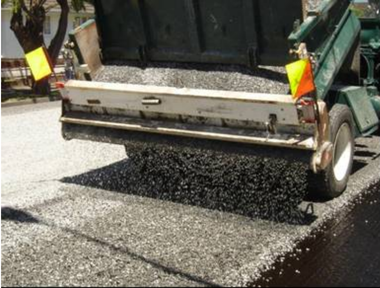
Figure 5.4 Application of the grade 5 chip
