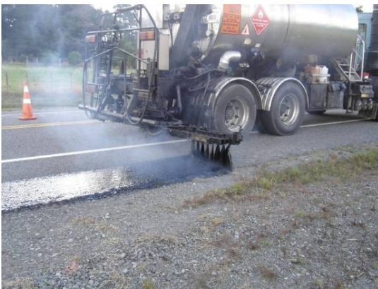
Figure 6.2 Spraying the 180/200 sealing binder
