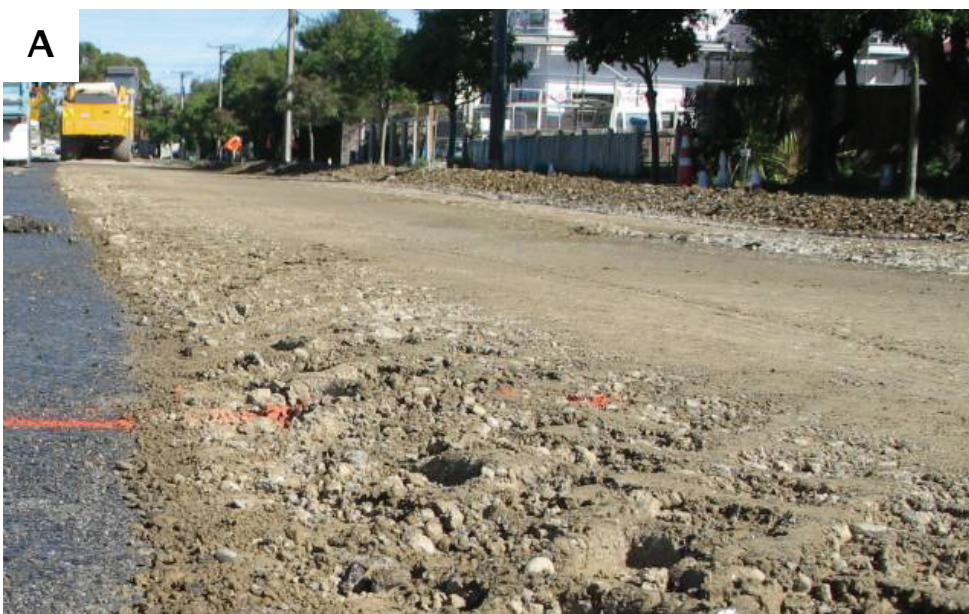
Figure 3.27 Recycled pavement layer of Burke St showing a high amount of fine clay in the surface (a). A high proportion of clay is clearly evident from the largely ‘dirt-like’ appearance of the surface of a compacted sample of 4A (b)
