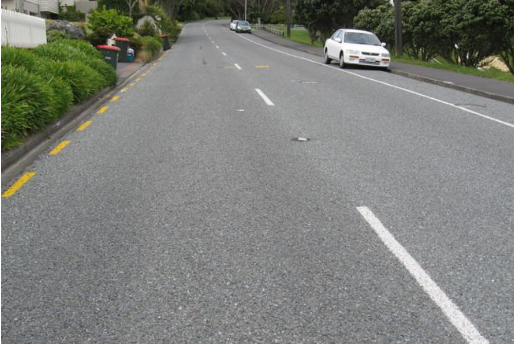
Figure F1 LOW S_1 Site 32, Wellington: A new, diffuse chipseal surface with S_1 = 0.24 ( Q_o = 0.049 )
