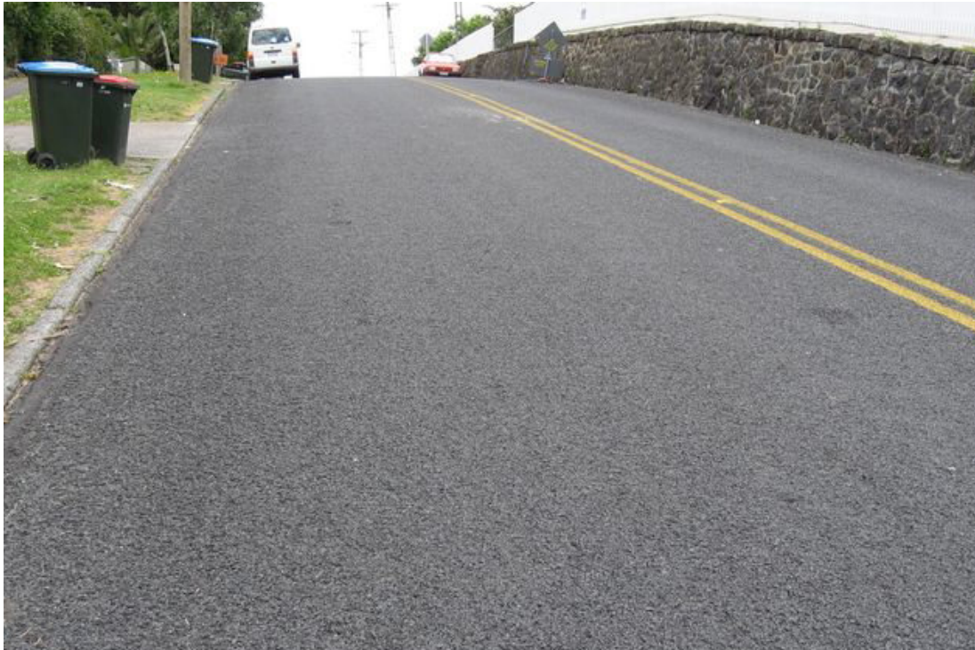
Figure F3 LOW Q_o . Site 73, Auckland: A dark, 1-year-old chipseal surface with Q_o = 0.028 , ( S1 = 0.52 )
