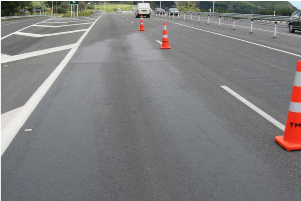
Figure F2 HIGH S_1 Site 122, SH1 Wellington: A flushed chipseal surface that is highly specular in the wheel track. S_1 = 1.19 ( Q_o = 0.065 ).
