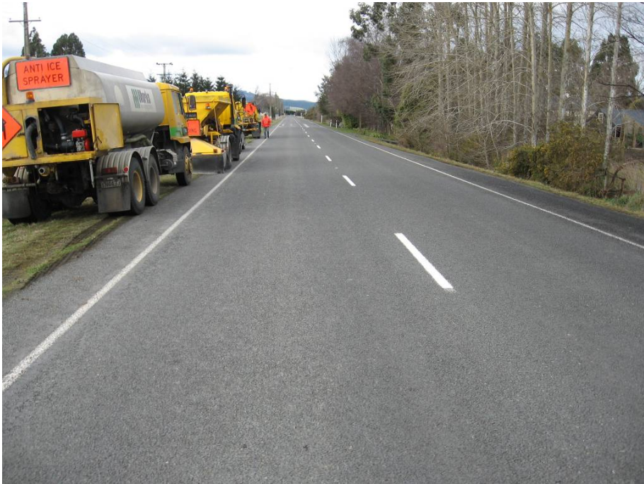
Figure A.3 View looking towards the northeast (decreasing direction)
