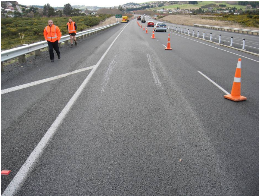
Figure A.1 View looking towards the northeast (increasing direction)
