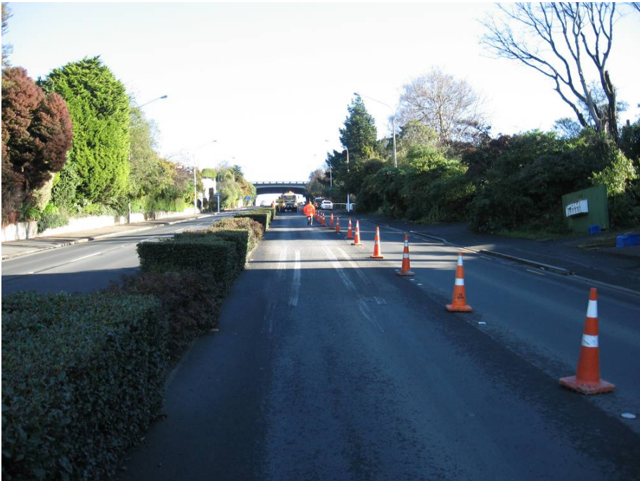
Figure A.7 View looking uphill towards the west
