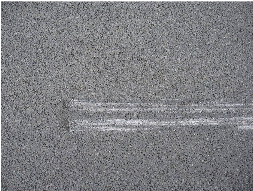
Figure A.2 View of surface (also shows tyre skid mark – mineral grit)
