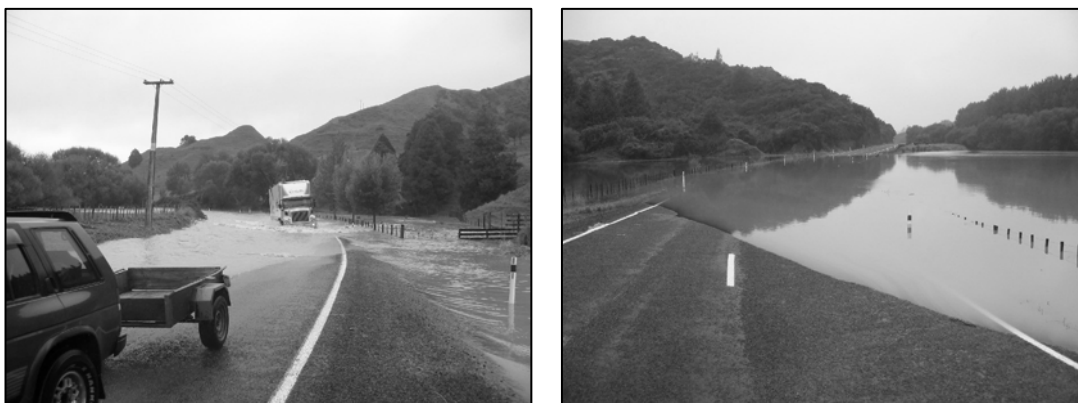
Figure 5.1 Surface flooding of the state highway network at Mapara and Honikiwi, Waikato.
