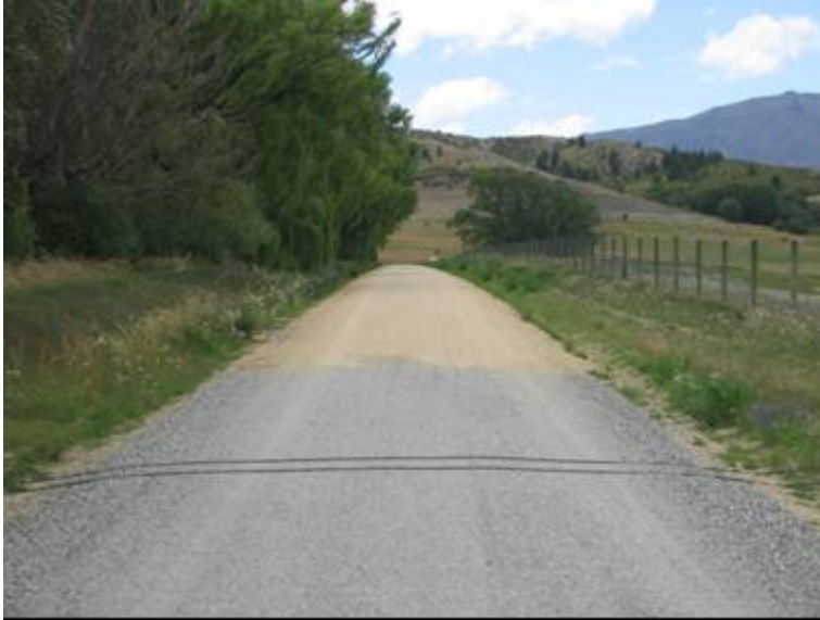
Figure 3.5 Keddell Road - Otta seal section and untreated section
