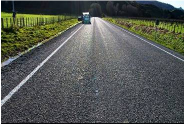
Figure A1.13 Paroa Road - a seal extension replaced the emulsion section (photo taken August 2007)
