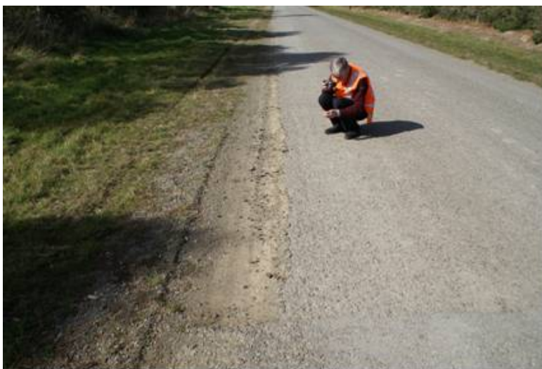
Figure 5.2 Edgebreak on Mayes Road site (August 2007)
