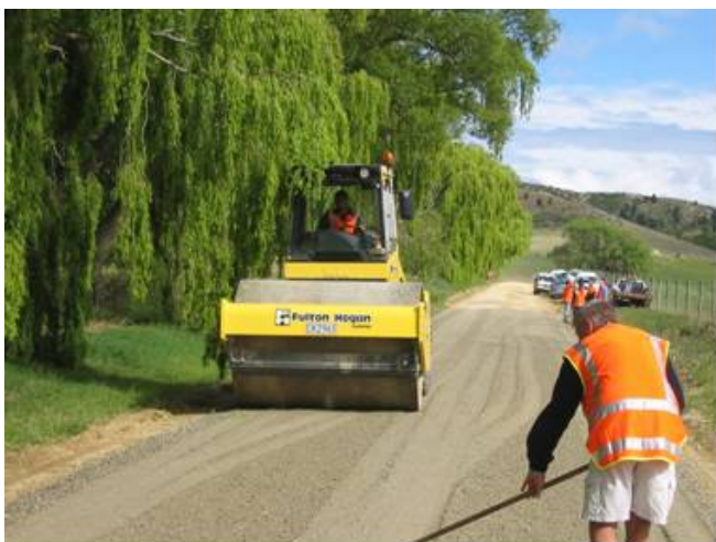
Figure 4.3 Rolling the Otta seal, Keddell Road
