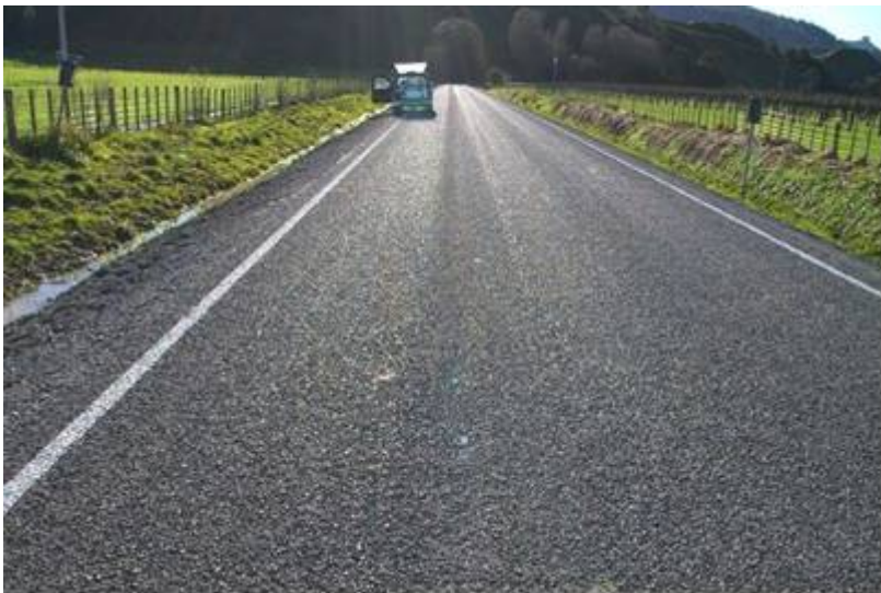
Figure 6.4 Paroa Road seal extension (December 2007)
