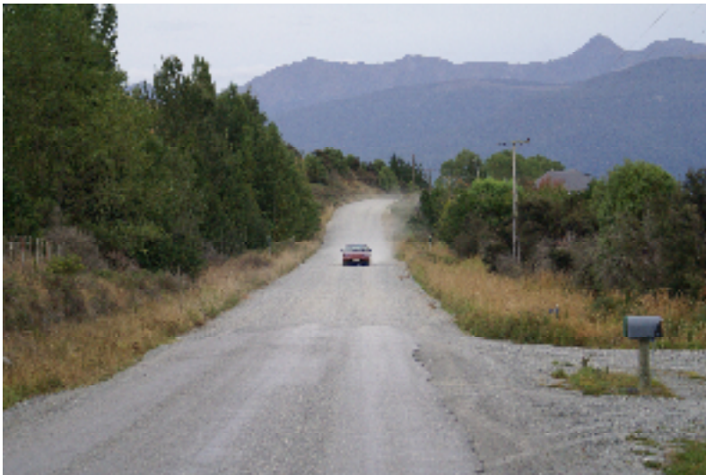
Figure 3.6 Sinclair Road, looking towards the lake from the end of the Otta seal
