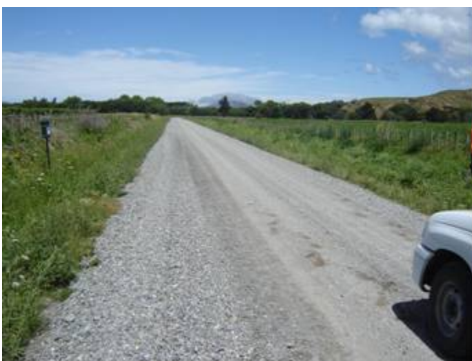
Figure A1.12 Paroa Road - emulsion section, looking south
