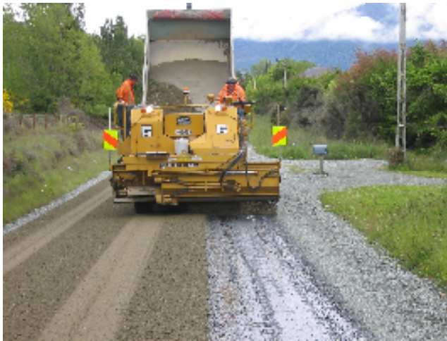
Figure 4.2 Spreading aggregate on Sinclair Road, using the chip spreader
