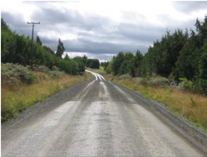
Figure A1.1 Sinclair Road - on Otta seal, looking north to oil section
