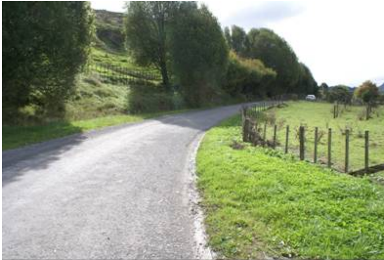
Figure 3.3 Paroa Road Otta seal
