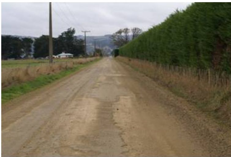
Figure 3.4 Church Road waste oil section (May 2007)
