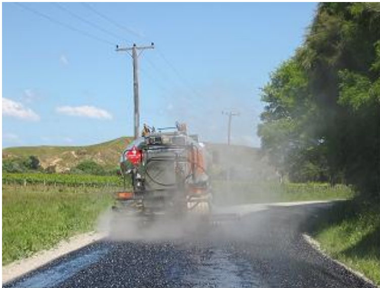
Figure 4.1 Spraying NRO on the Paroa Road site
