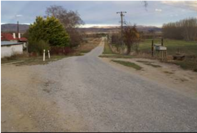
Figure A1.5 Keddell Road - from centre of Otta seal, looking south to oil section
