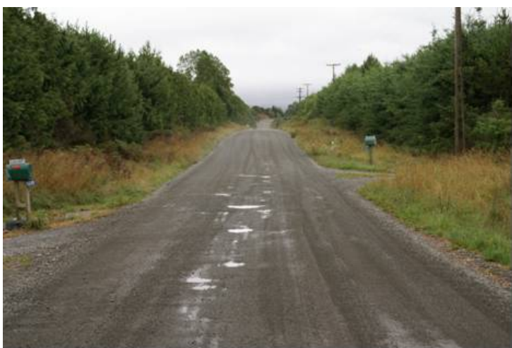
Figure 6.1 Sinclair Road waste oil section, looking south (Jan 2008)
