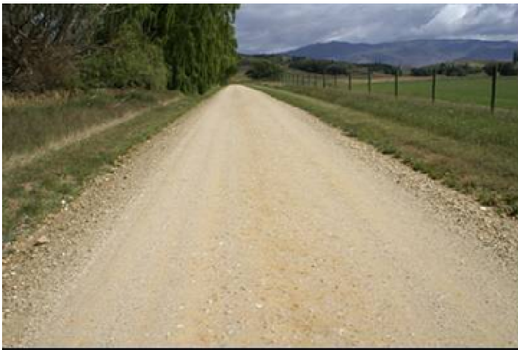
Figure 6.2 Keddell Road untreated section
