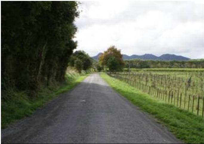
Figure A1.10 Paroa Road - Otta seal, looking north towards start of trial
