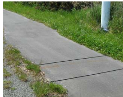
Figure AB.1 Typical off-road path counting installation.
