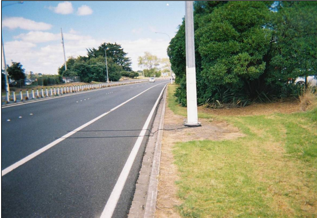
Figure AA.5.2 George Bolt Memorial Drive - typical section of George Bolt Memorial Drive.
