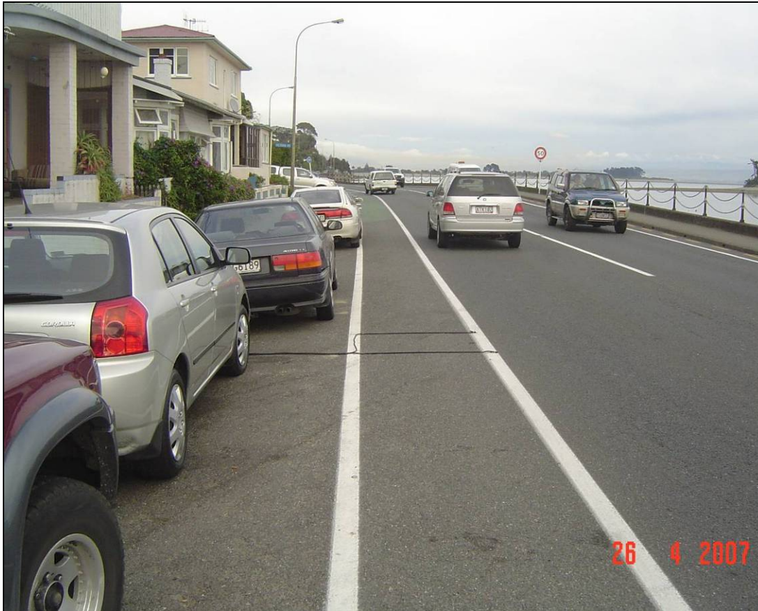
Figure AA.3.2 Typical section of Wakefield Quay showing narrow cycle lane and carriageway widths.
