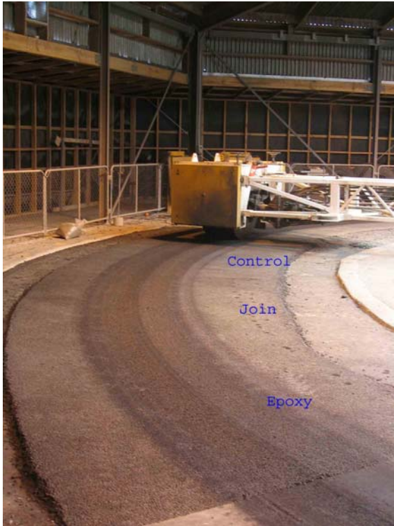
Figure 6.6 CAPTIF trial: Test sections after trafficking.
