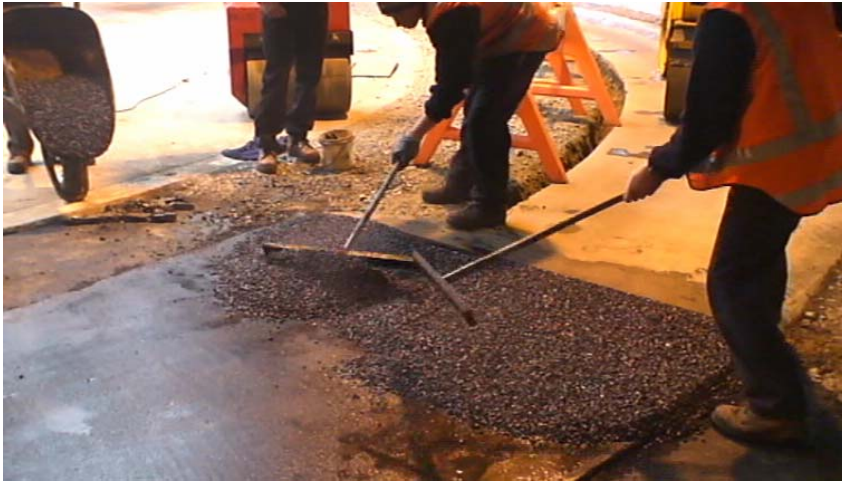
Figure 6.3 CAPTIF trial: Laying epoxy OGPA test section.
