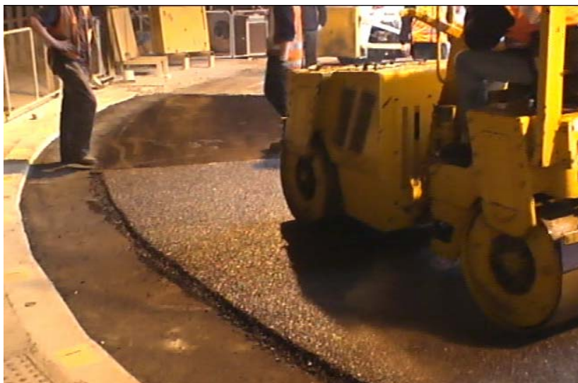
Figure 6.5 CAPTIF trial final compaction of epoxy test section.
