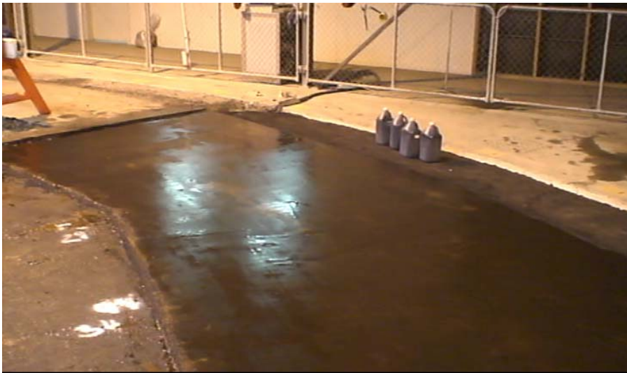
Figure 6.2 CAPTIF trial: Polymer modified bitumen emulsion tack coat.
