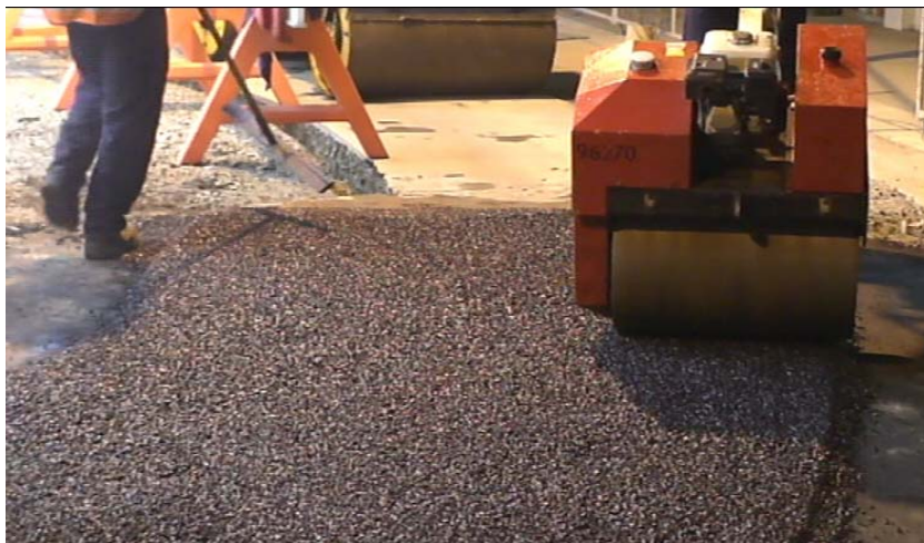
Figure 6.4 CAPTIF trial: Initial hand compaction of epoxy test section.
