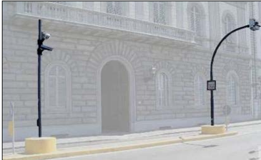
Figure 4.7 Italian Access Control Systems.
