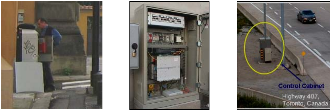
Figure 4.6 Typical roadside controllers.
