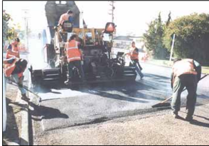
Figure 3.5 15% RAP mix being laid in 2003.
