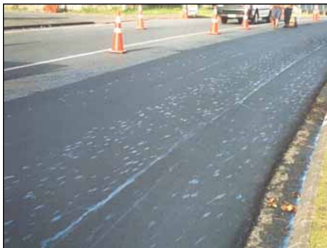
Figure 4.5 Crumb rubber mix laid in 2004.
