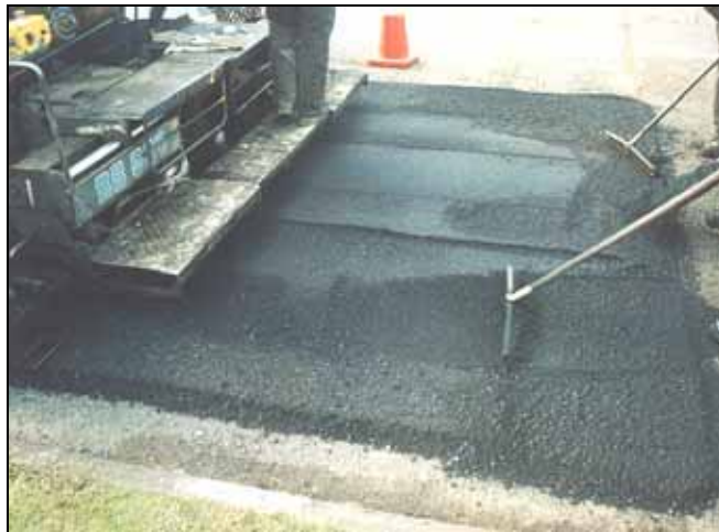
Figure 4.4 Crumb rubber mix laid 2004.
