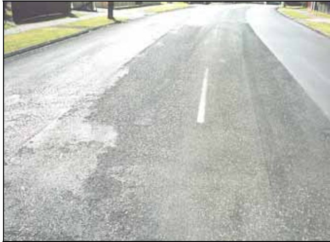
Figure 4.6 Crumb rubber mix showing one good paver run on the right and the other two runs that failed.
