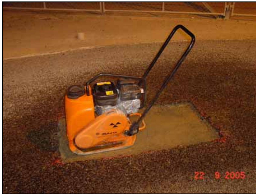
Figure 4.6 Typical surface repair of a failed area.
