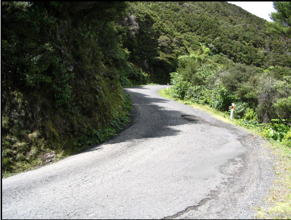
Figure 4.8 Example of edge break.
