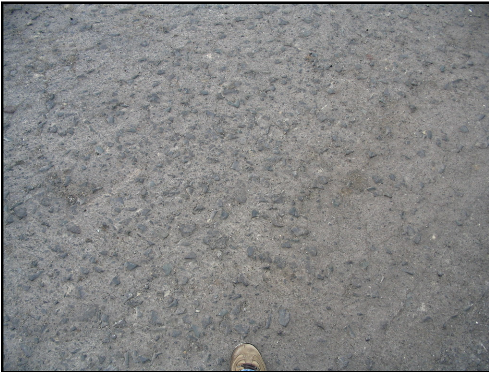
Figure 4.5 Bound surface of trial section on Aotea Road.
