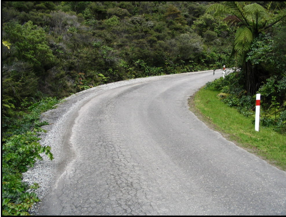
Figure 4.6 Crocodile-cracked surface.
