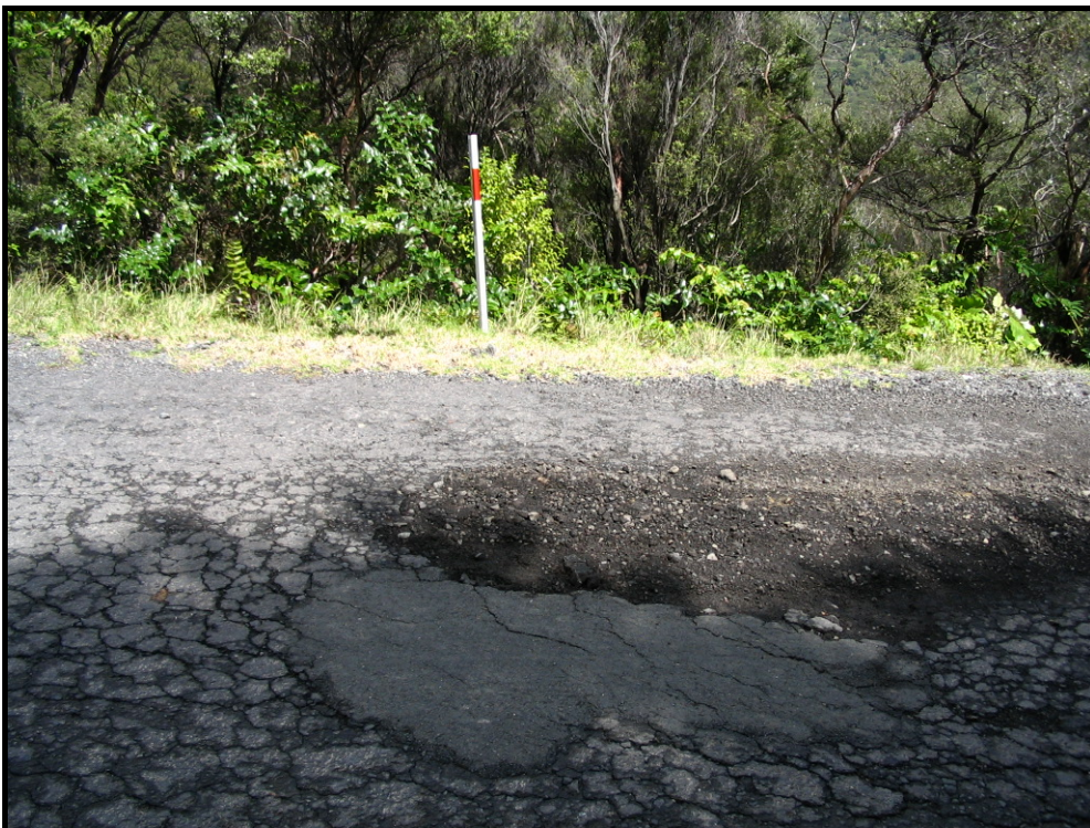
Figure 4.9 Potholing in the surface of the trial section.
