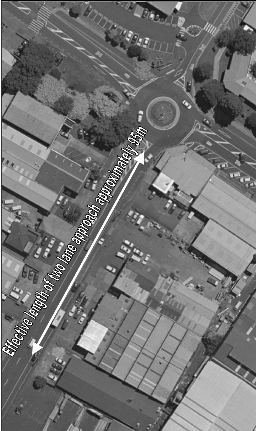
Figure D1 Frost Road/Carr Road intersection showing effective length of the two-lane approach.
