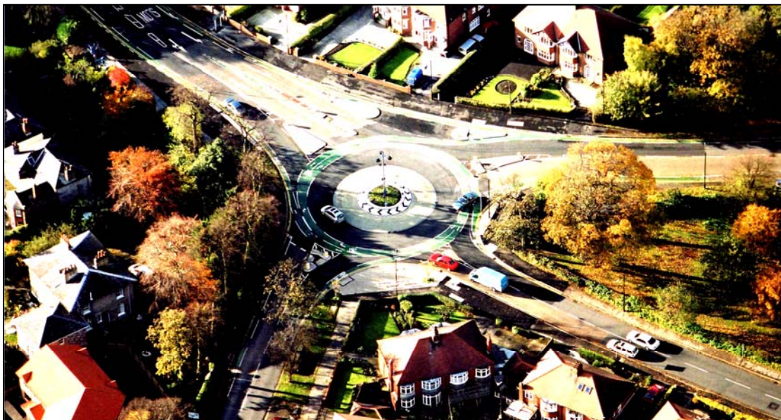
Figure 2.1 Roundabout with coloured cycle lanes on the carriageway in the City of York, United Kingdom (photo courtesy of City of York Council).
