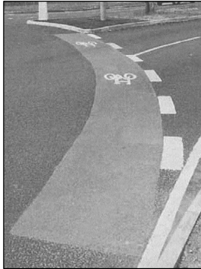
Figure 2.2 Coloured cyclist strips adjacent to limit lines in Gloucester, UK (Lawton et al. 2003).
