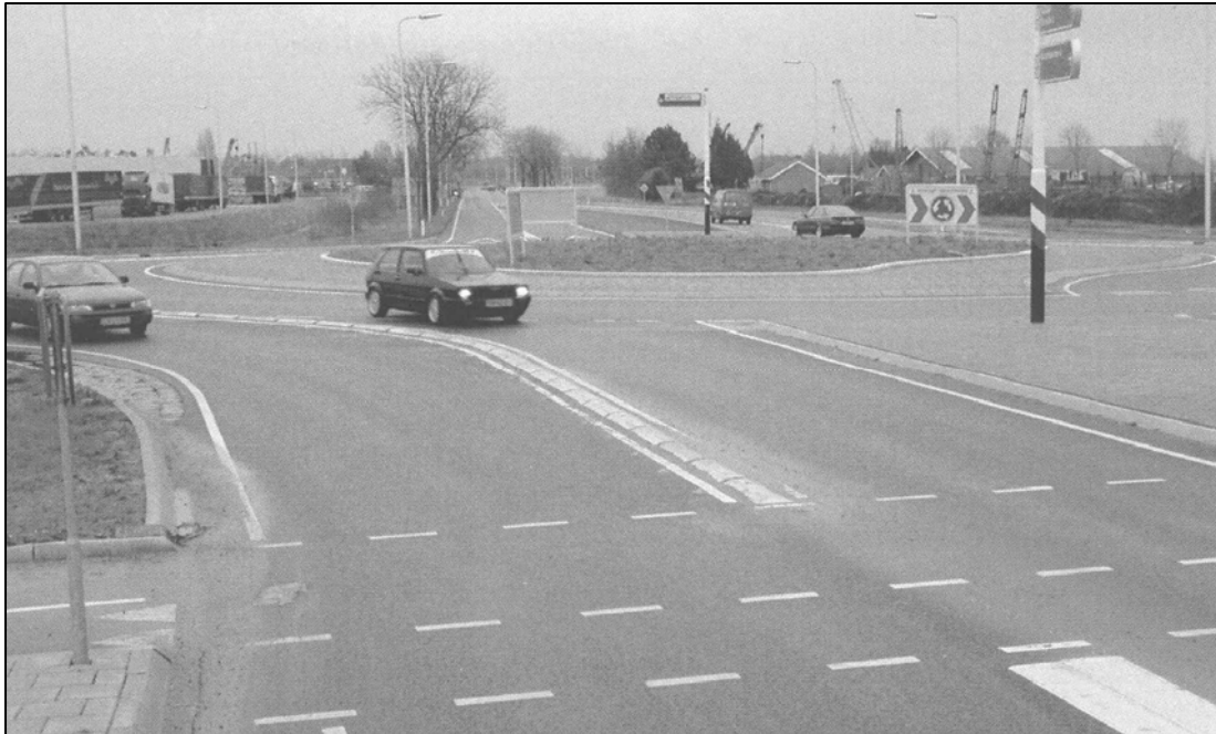
Figure 2.4 The turbo-roundabout in the Netherlands with traversable lane dividers and the off-road cyclepath visible in the foreground (Fortuijn 2003).
