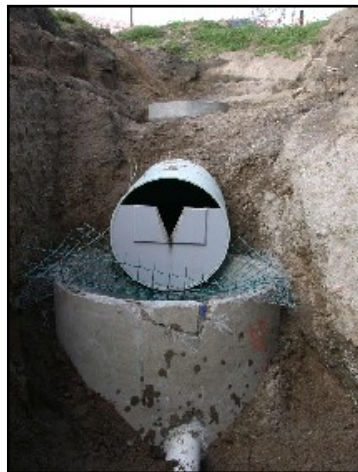
Figures 3.7 & 3.8 Runoff volume at the Cambridge site is measured in the weir before flowing into the treatment wall in the concrete riser below the weir.
