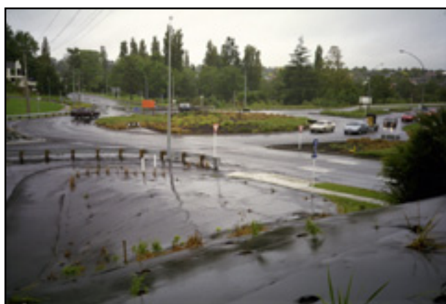
Figure 3.1 The Hamilton site. The orange hazard fence surrounds the treatment wall.
