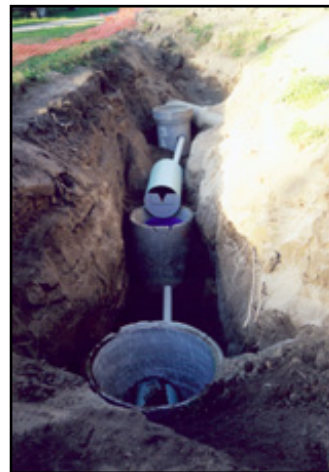
Figures 3.7 & 3.8 Runoff volume at the Cambridge site is measured in the weir before flowing into the treatment wall in the concrete riser below the weir.
