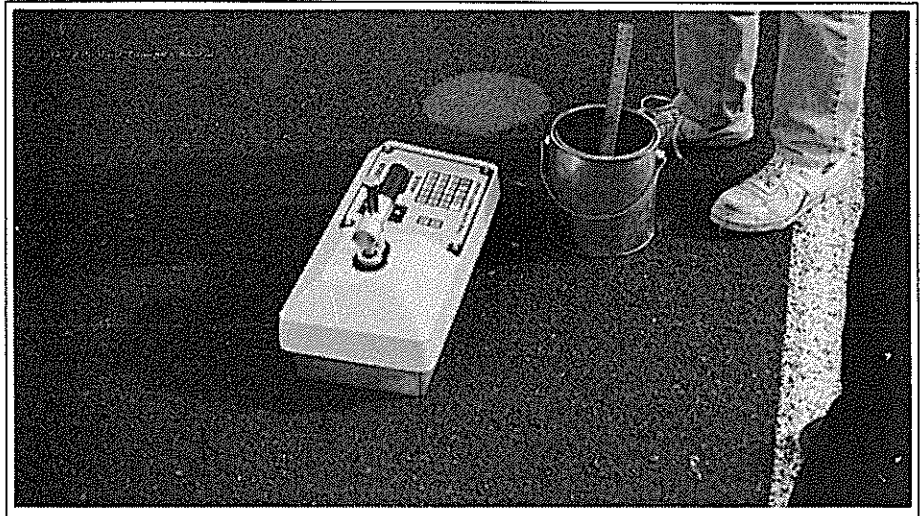
Figure 5.2 Troxler thin surfacing nuclear densometer for measuring density, and adjacent is the sand circle test for texture.
