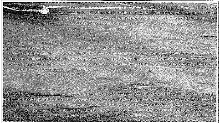
Figure 6.5 Shoving at the intersection was evident during the entire trial, and shown on 1996 and 1997 maps (Figures 6.1, 6.2).
