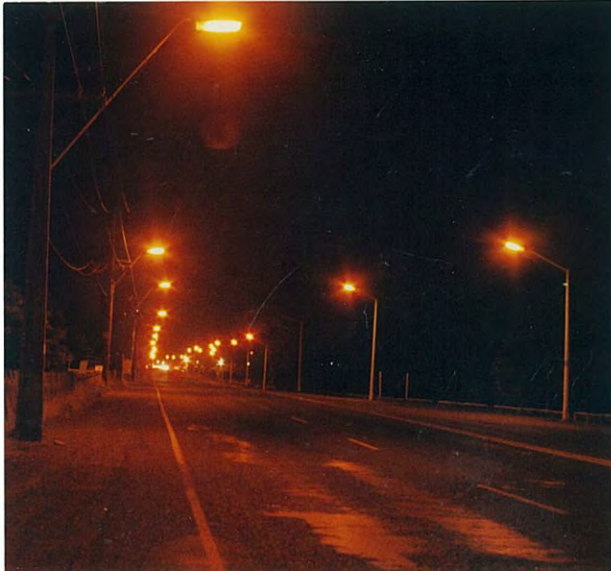
Upper Hutt, Fergusson Drive Bridge to St Patrick's \bar{L} = 0.54 \text{ cm/m}^2 , U_o = 0.48 , TI = 40\%
