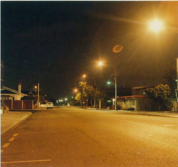
Lower Hutt Cornwall Street \bar{L} = 0.60 \text{ cm/m}^2, U_o = 0.59 Site No. 29
