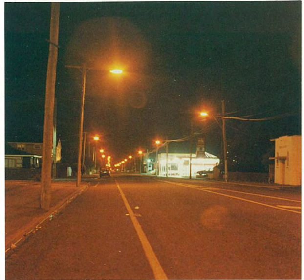
Upper Hutt, Fergusson Drive Whakatiki St to Main St L=0.55 \text{ cm/m}^2 , U_o=0.36 , TI=21\% Site No.3
