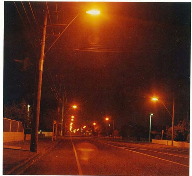
Upper Hutt, Fergusson Drive St Patrick's to Camp Street \bar{L} = 0.57 \text{ cd/m}^2 , U_o = 0.39 , TI = 16\% Site No. 1
