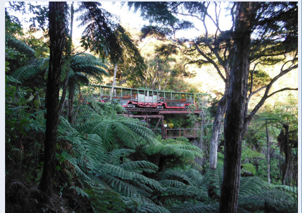
The child fell from the Snake Railcar as it travelled across the Double Decker Bridge. Photo: NZ Transport Agency
