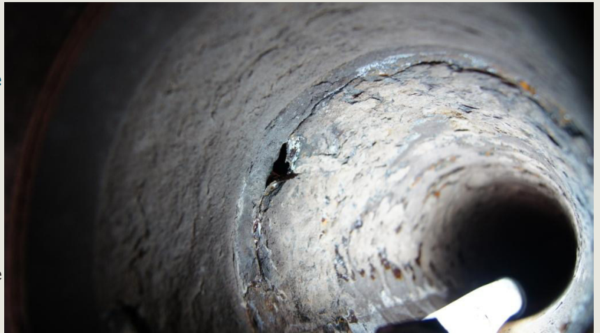
A428 dry pipe - interior view
