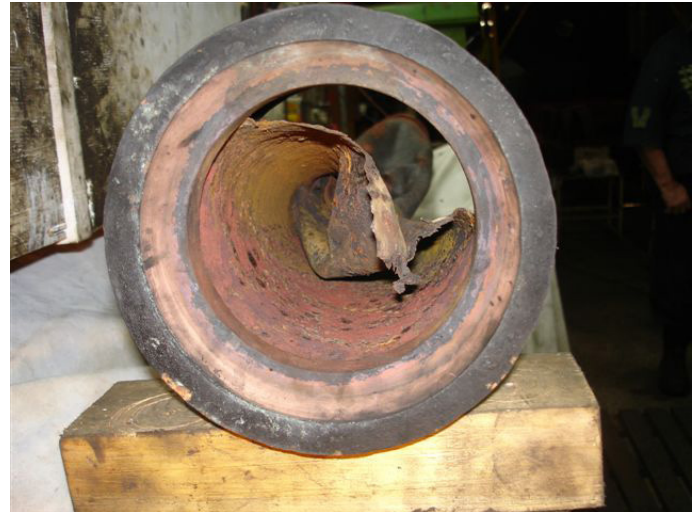
Collapsed dry pipe - end view
