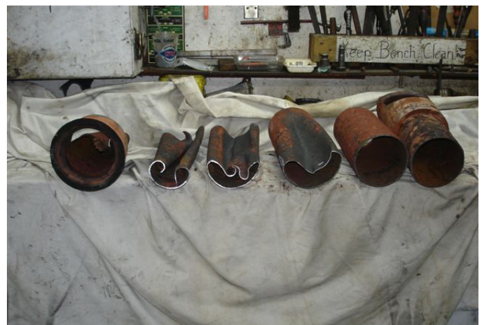
Dry pipe pieces
