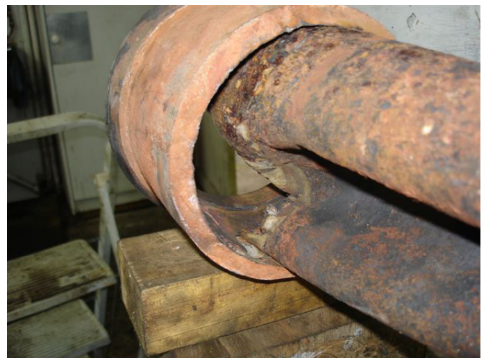
Dry pipe - joint view
