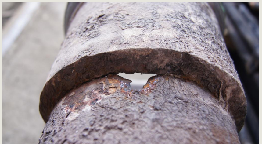
A428 dry pipe - exterior view
