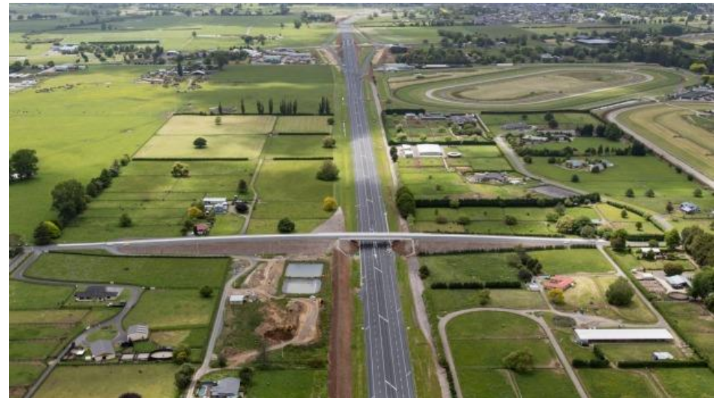
The Peake Road overbridge crosses an arrow-straight stretch of the Waikato Expressway.
