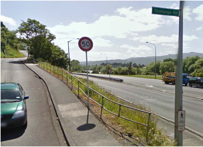
Figure 1: Typical pedestrian handrail
