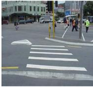
No tactile paving at the end of this pedestrian crossing. Note lack of dropped kerb in the central island.
