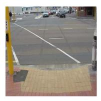
Redesigned intersection with old tactile paving unchanged - directing visually impaired pedestrians into on-coming traffic.
