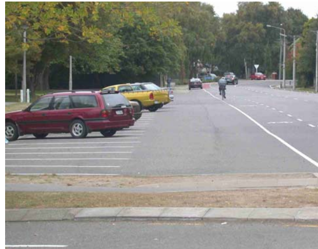
Figure 4-8: Cycle Lane next to Angle Parking (Christchurch)
