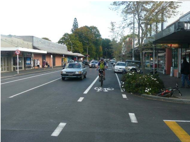
Figure 4-2: Cycle lane next to parking (Dunedin)
