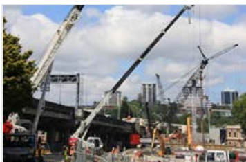
Victoria Park Tunnel. (JPG, 125KB)
