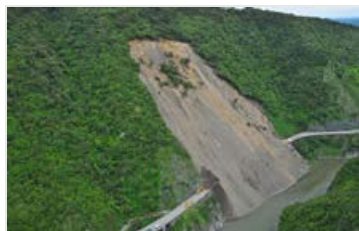
Working on the Manawatu Gorge slip, November 2011. (JPG, 119KB)
