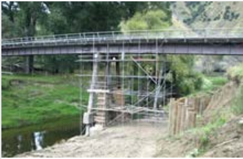
Goodwin Road Bridge. (Photo courtesy of Gisborne City Council) (JPG, 150KB)
