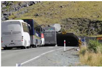
Homer Tunnel, West Coast South Island. (JPG, 145KB)
