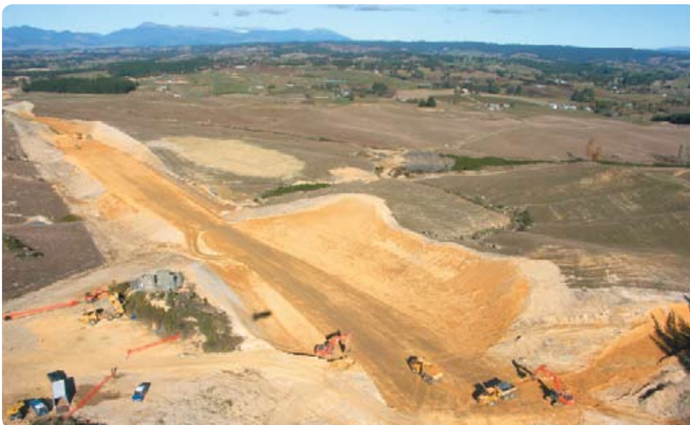
Construction of the SH6 Ruby Bay Bypass is under way.
