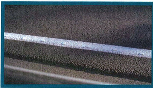
Fig 1 Audio Tactile Edge Line Marking not meeting Specification
