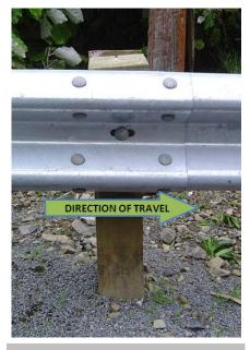
Figure 1 Standard Rail Lapping
