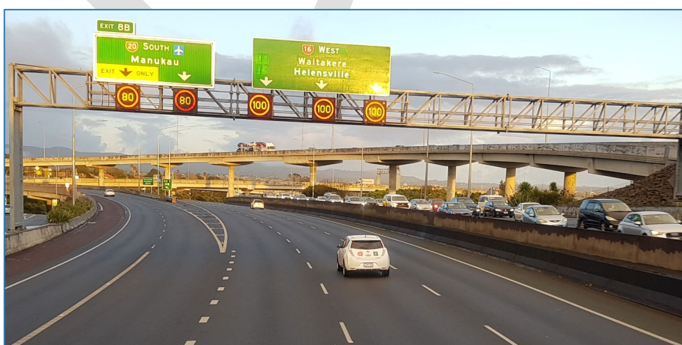
Figure 8. LCSs on a gantry spanning motorway
