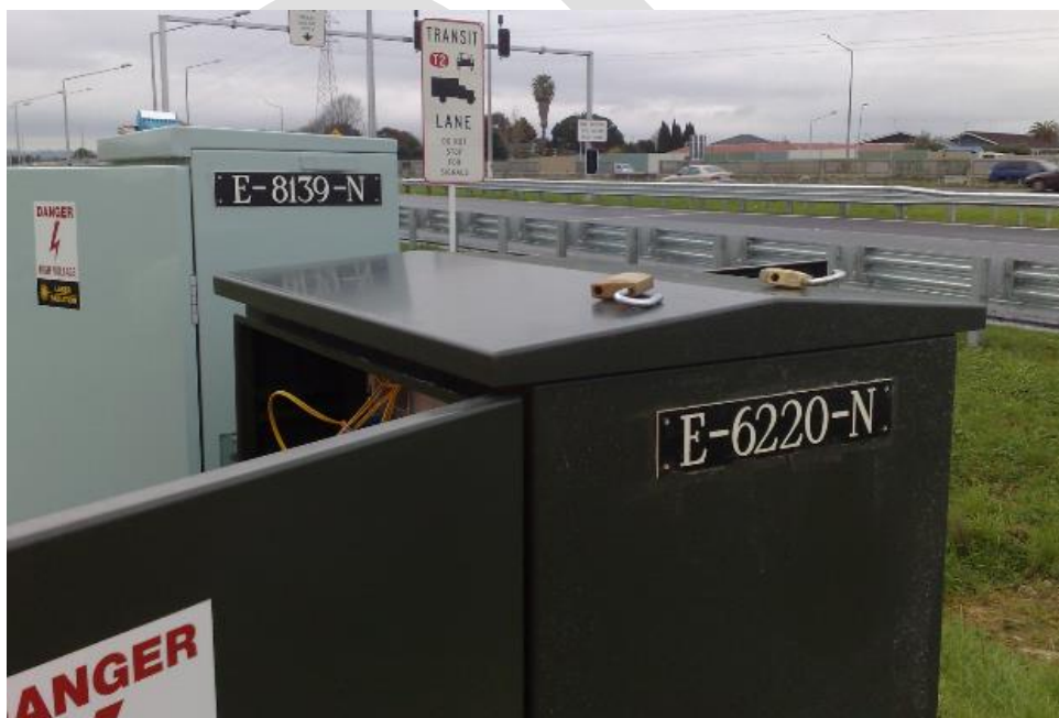
Figure 2: Communications cabinet E-6220-N and Ramp Signals Cabinet E-8139-N with their identification labels facing the approaching traffic
