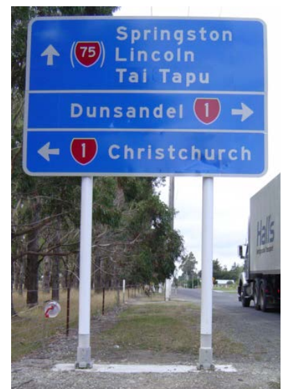
Figure 1 Correctly installed slip base sign supports
