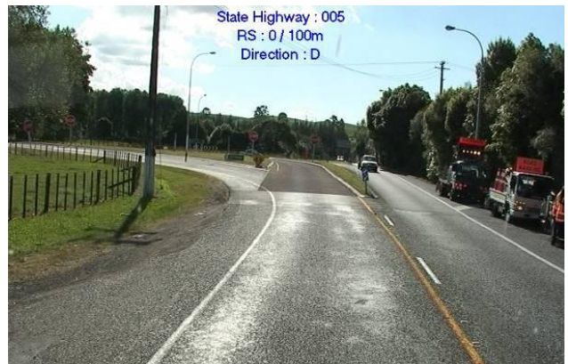
Looking northwest towards the head of the intersection on minor road
