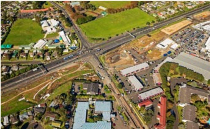
SH20A Kirkbride Road intersection, May 2015
