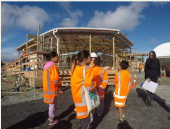
H&S manager welcoming our team to the site
