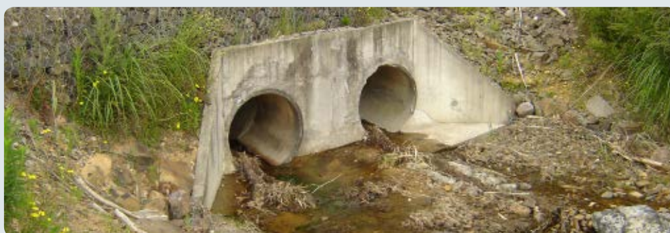
FIGURE 20 Double culvert with the installation of rope
