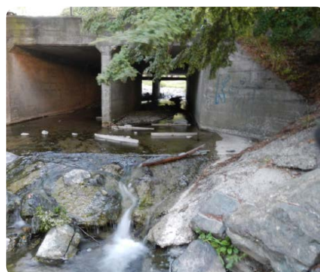
FIGURE 12 Double box culverts
