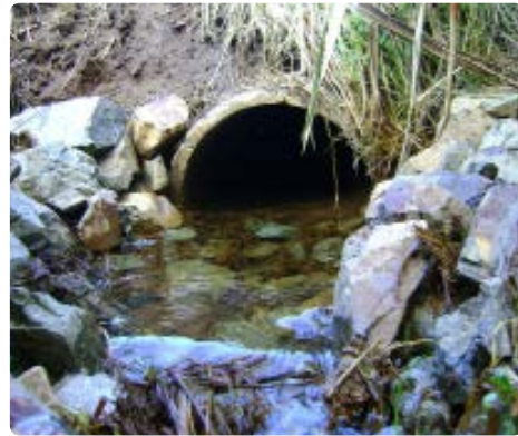
FIGURE 17 The effective use of rock armouring at a culvert outlet
