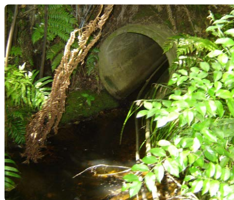
FIGURE 11 An arch culvert that maintains stream bed and has also a low flow channel
