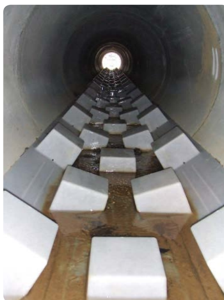
FIGURE 15 Baffles inside a culvert
