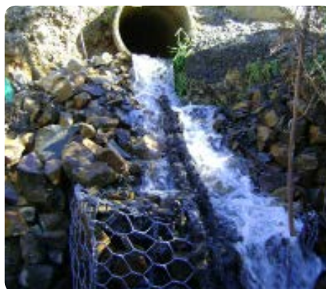
FIGURE 16 Rope has been installed in this culvert to aid fish passage
