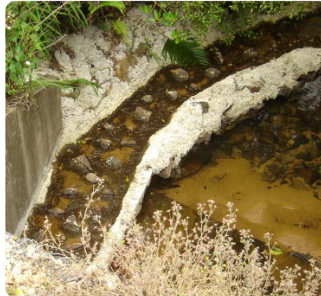
FIGURE 19 A concrete ramp which has been embedded with cobbles to air fish passage
