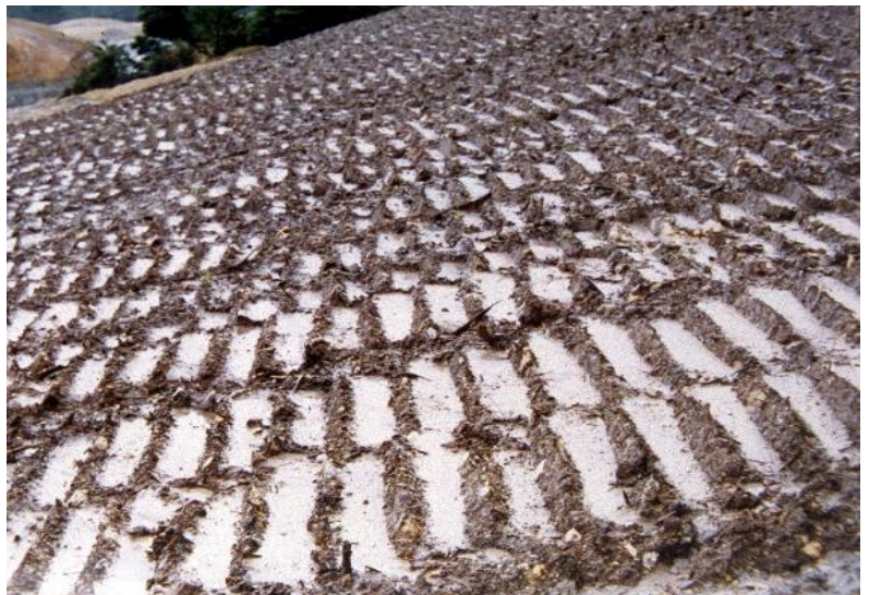
Surface roughening of a slope. Note the hollows acting as “micro” sediment traps
