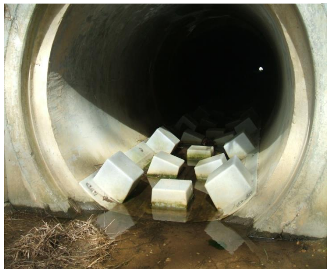
Culvert with Fish Passage Provided Through Energy Dissipation
