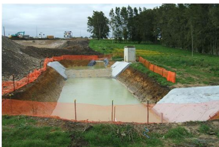
Sediment Retention Pond
