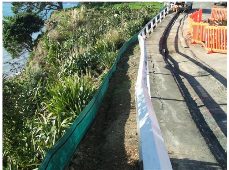
Silt Fence installed on edge of works
