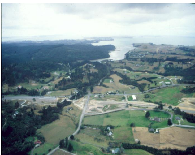
Highway Construction Immediately Upstream from the Okura Estuary
