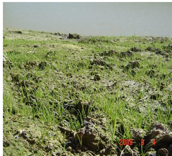
Recently applied hydroseed showing emergent grass growth
