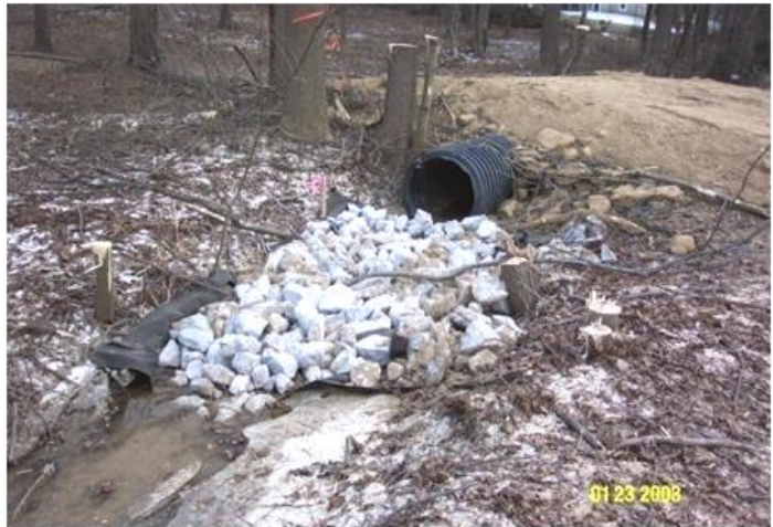
Culvert with Fish Passage Provided Through Energy Dissipation
