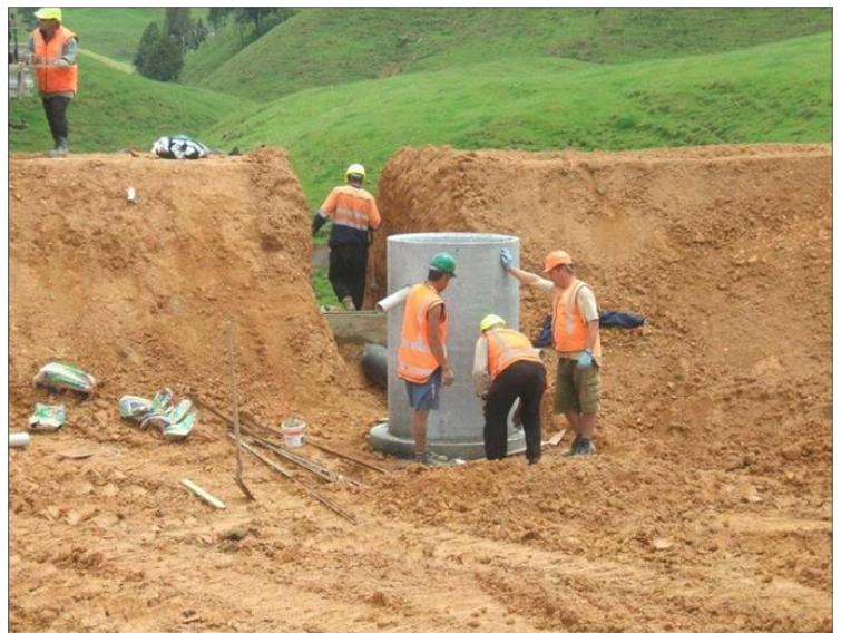
Construction of a Sediment Retention Pond
