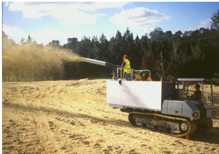
Mulching being applied in preparation for winter shutdown of the site
