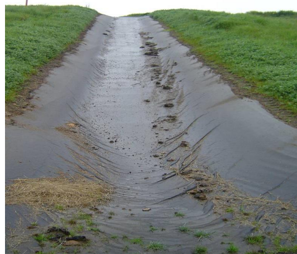
Geotextile lined flume
