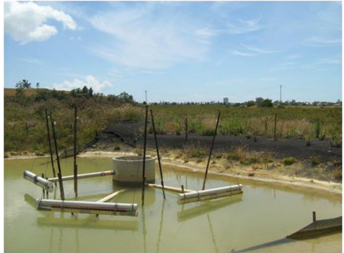
Decants on Rope and Pulley System
