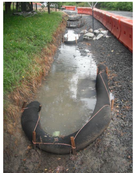
Filter sock check dams (image provided by Erosion Control Co. Ltd.)
