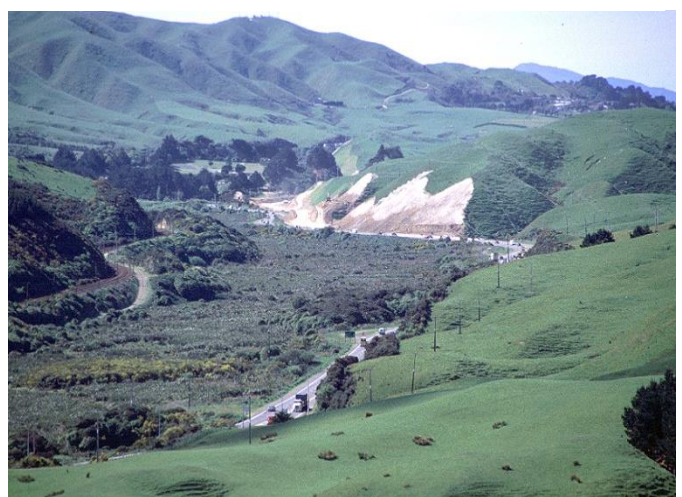
Highway Construction Adjacent to the Pauatahanui Estuary near Porirua
