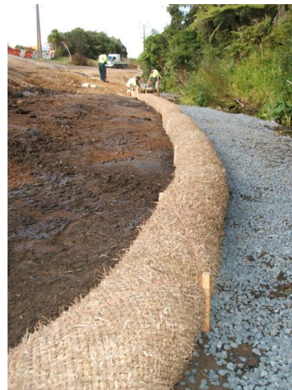
Straw filled filter sock (Image provided by Erosion Control Co. Ltd.)
