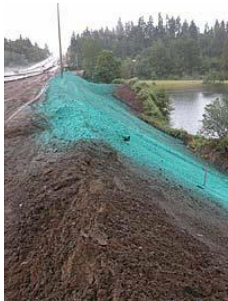
Mulch Cover – approximately 20 – 40% density = inadequate cover for stabilisation
