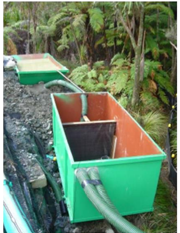
Dewatering Skip Bin
