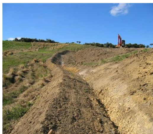
Diversion separating the clean water from the dirty water
