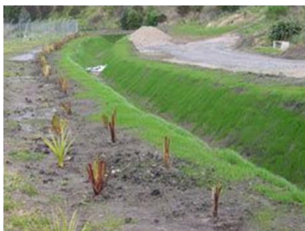
Enkamat used as erosion protection and medium for revegetation. Source: Maccaferri NZ Ltd
