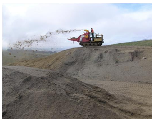
Erosion Control – Mulching
