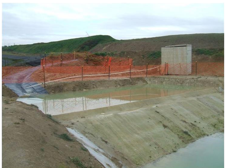
Level Spreader and Forebay
