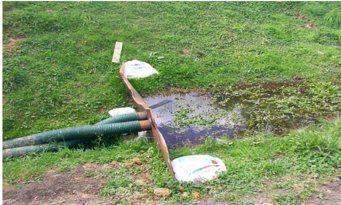
Water Being Diverted Past a Construction Site
