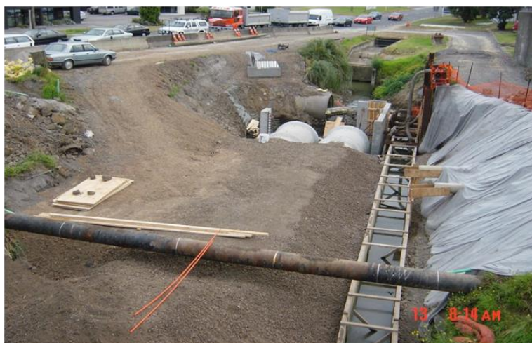
Use of Marine Ply as a Stream Diversion Approach
