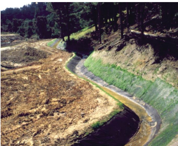
Waterway Diversion on a Highway Project
