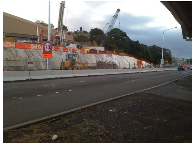
Geotextile used as a temporary stabilising agent on cut embankment.
