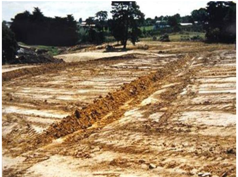
Contour drain. (Source: Environment Canterbury)
