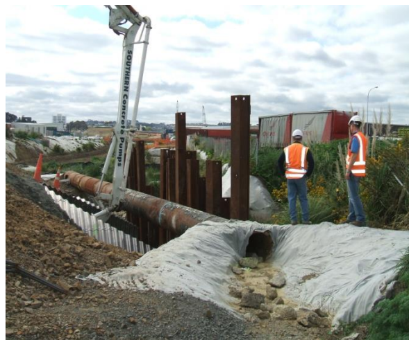
Temporary Culvert Stream Diversion
