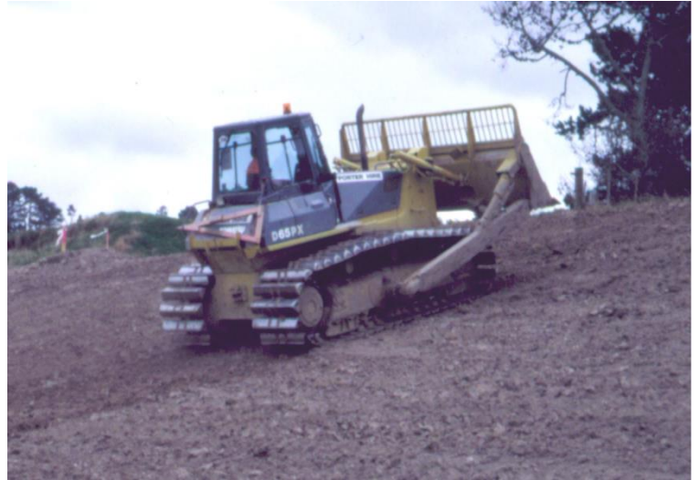
Surface roughening with bulldozer
