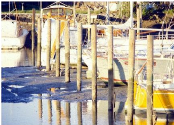
Marina Infilling by Sediment from Upstream Earthwork Activities
