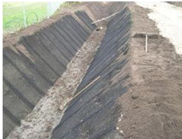
Enkamat used as erosion protection and medium for revegetation. Source: Maccaferri NZ Ltd
