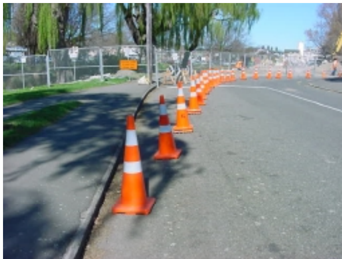
Figure C12.1: Showing Delineation Taper in Advance of Safety Fence.
