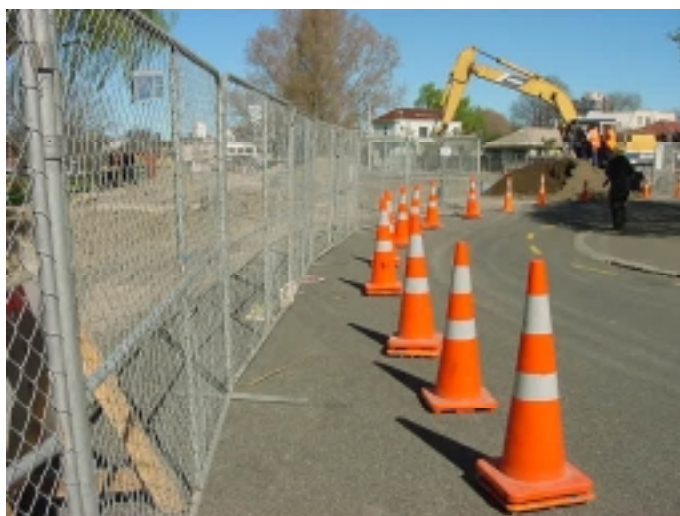
Figure C12.2: Excavation and Site Protected by a Safety Fence. Note the Lateral Safety Zone and Delineation
