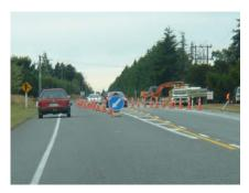
of the road, signs are only required on the left-hand side of the road. The RCA, engineer or contractor can request signs on both sides of a road, when this is considered desirable for safety or traffic management reasons.
