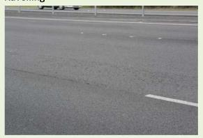
Loss of chip from an asphaltic concrete or a slurry surface. It occurs where the binder has oxidised and is losing its grip on the surfacing aggregate.
