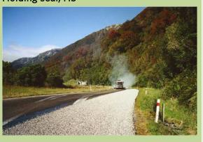
A chipseal constructed in an attempt to extend the life of a failed pavement for a short period.
