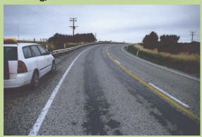
Scabbing as a failure mechanism in an old chipseal (typically aged > 10 years old) where the binder fails and chip is lost due to the increased hardness and brittleness of the bitumen.
