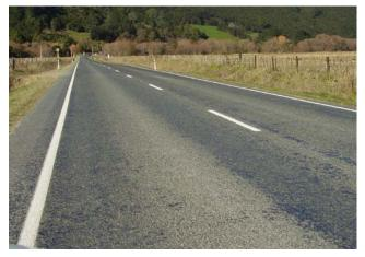
Densification occurs in both the layers of chipseal and also the underlying pavement layer causing depressions in the wheel paths.
