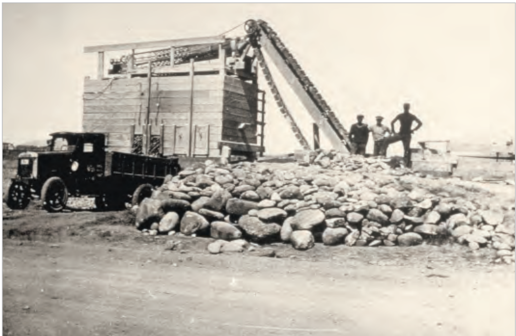
Figure 8-20 Screening aggregate for road use from a beach near Opunake, Taranaki, in the 1920s.
