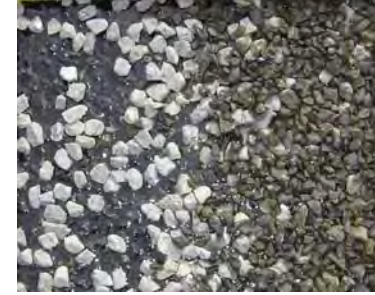
Application of the second chip
