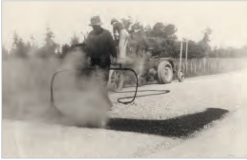
Figure 3-6 Constructing a first coat chipseal near Gisborne in the 1920s was not highly mechanised, compared to the line of construction machines used in the 2000s shown in Figure 3-7. Left: Hand spraying the basecourse, from the tractor-drawn bitumen distributor. Right: Spreading the chip by shovel as the tip truck was not yet in use. Photos courtesy of John Matthews, Technix Group Ltd
