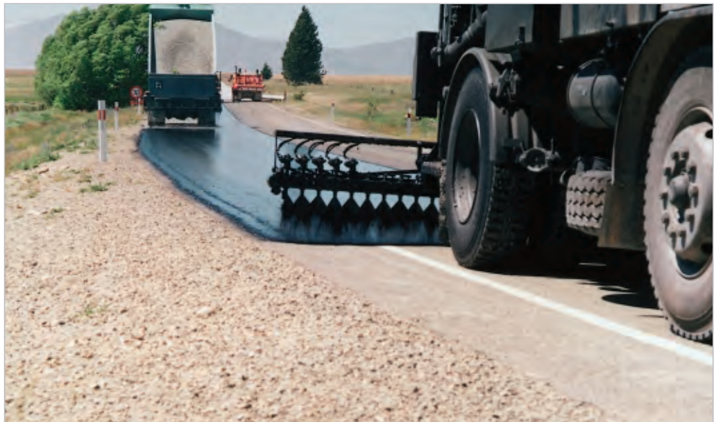
Figure 10-1 A sprayer in operation showing the spray fans. Note the different shape of the fan coming from the end nozzle.
