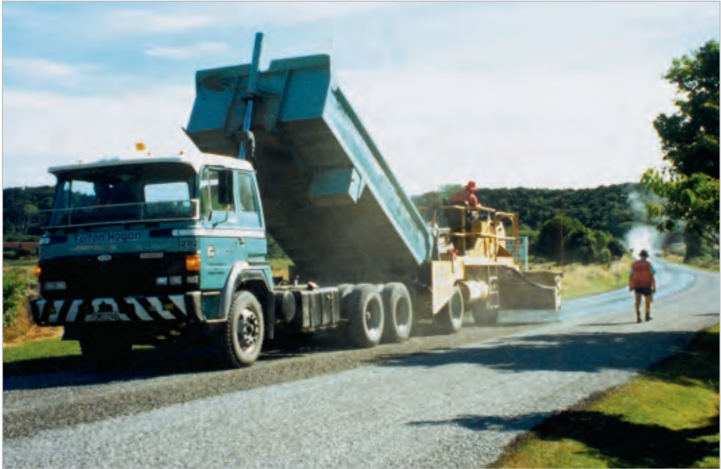
Figure 10-18 A truck supplying chip to a self-propelled chipsealer during a chipsealing operation. Photo courtesy of Les McKenzie, Opus
