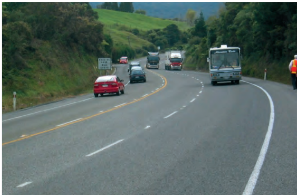
Figure 6-6 A chipseal on climbing lanes where high speed traffic passes heavy vehicles.
