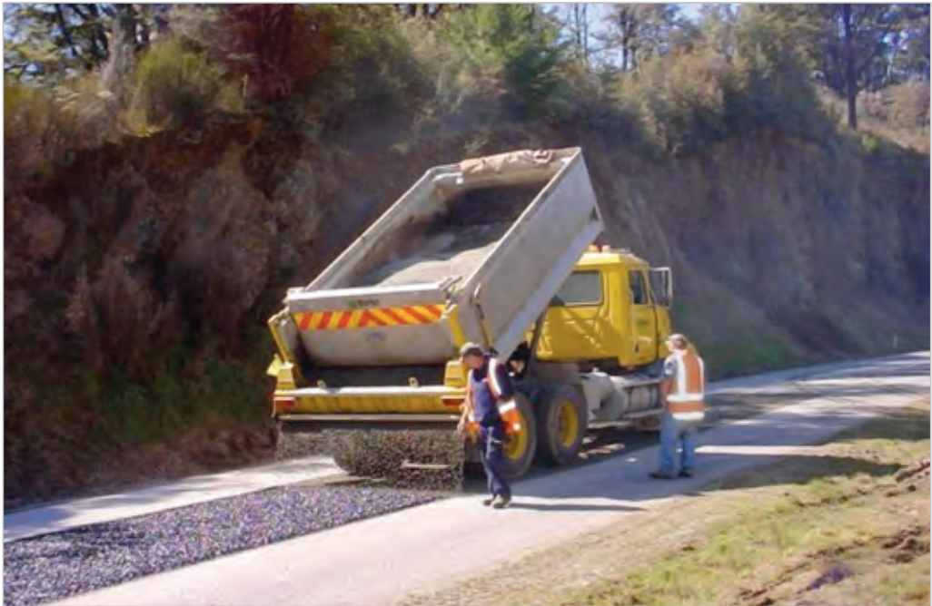
Figure 10-19 Tailgate roller spreader. Photo courtesy of Philip Muir, Works Infrastructure Ltd
