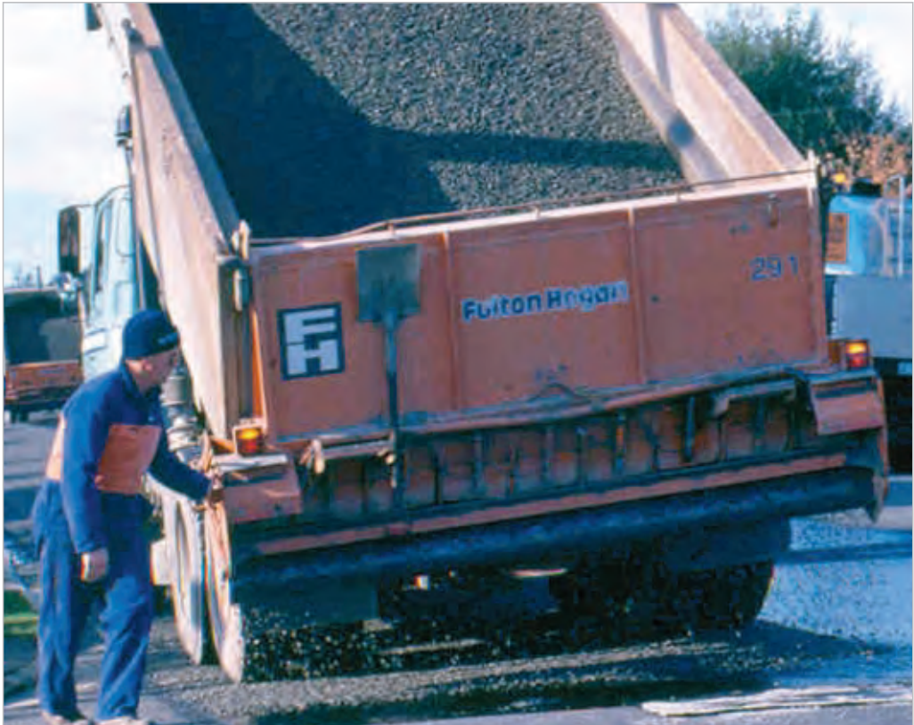
Figure 10-21 Procedure for calibrating chip spreading on paper.
