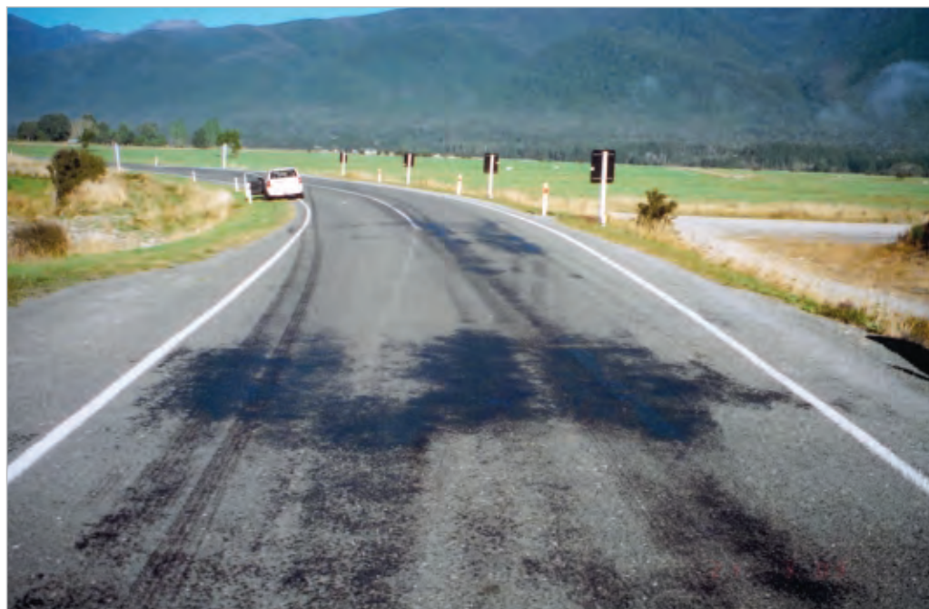
Figure 12-3 A surface showing both bleeding and tracking on a hot summer day, possibly caused by an old repair patch. This has caused the current chipseal to flush and bleed.
