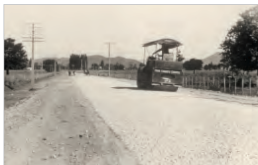
Figure 7-2 Preparation of basecourse for chipsealing has changed a great deal in the last 80 years. Left: A steam roller compacts a new basecourse on State Highway 2 near Manutuke, Cook County, Gisborne, in the 1920s.
