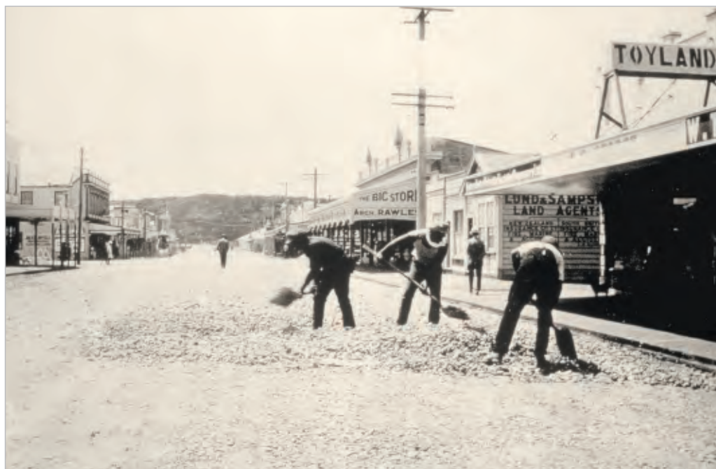
Figure 7-4 Even when chipsealing was less common, failures soon after pavement construction occurred, as they may do today. Here this road works team repairs a non-compliant section of freshly compacted pavement in the main street of a small New Zealand town in the 1920s.
