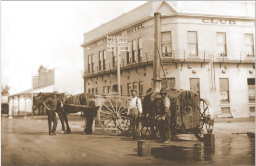
Figure I-4 Draughthorse-drawn bitumen hand sprayer ready for sealing the main street of Opunake, Taranaki, in the 1920s. Photo courtesy of Feaver Collection, Puke Ariki Museum Archives, New Plymouth
