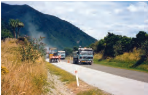
Figure 3-7 Constructing a chipseal. Clockwise from top left: Spraying binder and spreading chips in one operation. Top right: Spraying the binder. Bottom right: Spreading the chips. Bottom left: Rolling the surface. Photos courtesy of Les McKenzie, Opus
