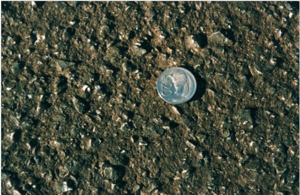
Figure 3-22 Detail of a cape seal surface. (The coin is about 3 cm diameter.)
