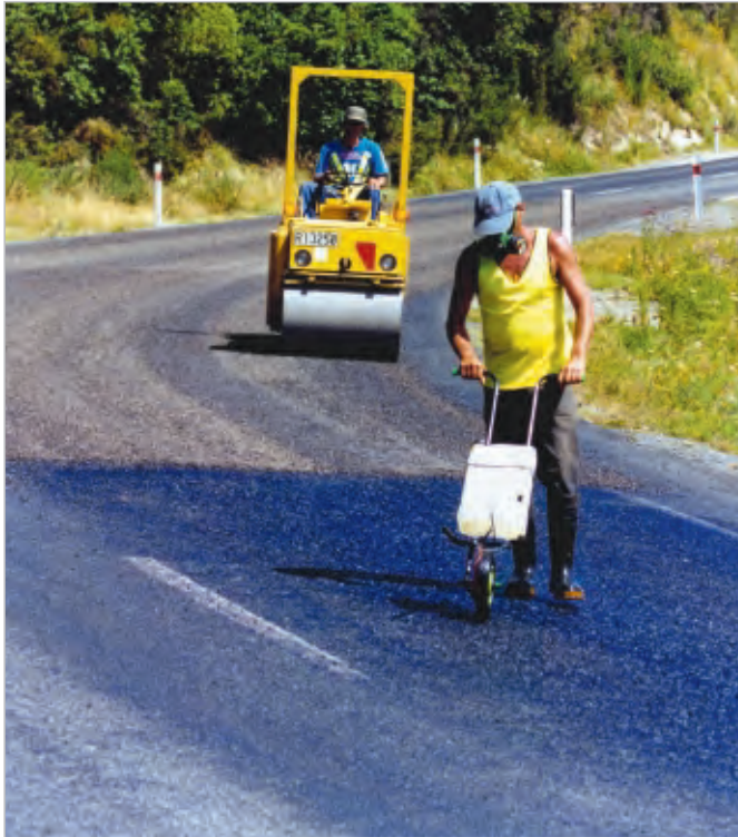
Figure 12-6 Solvent (e.g. kerosene) being applied before it is covered with chip.
