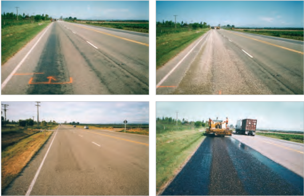
Figure 7-9 Dry chipping a flushed area before chipsealing the entire surface. Clockwise from top left in order of construction: Original surface marked out to show area to be dry chipped. Top right: Dry chip laid in wheelpaths. Bottom right: Binder is laid lane by lane over the dry chip. The next step is to lay the chip over the binder as for a conventional reseal. Bottom left: The completed surface.
