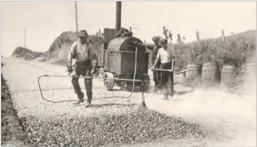
Figure 1-5 Most early chipsealing was carried out to keep down dust in the summer and mud in winter. In the 1920s this spray operator in Opunake County was using a hand sprayer with a swinging boom that kept the hose clear of the hot bitumen tank. Photo courtesy of John Matthews, Technix Group Ltd
