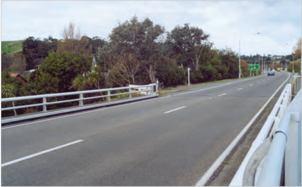
Figure 6-8 An approach road that is consistent with the bridge deck surfacing.
