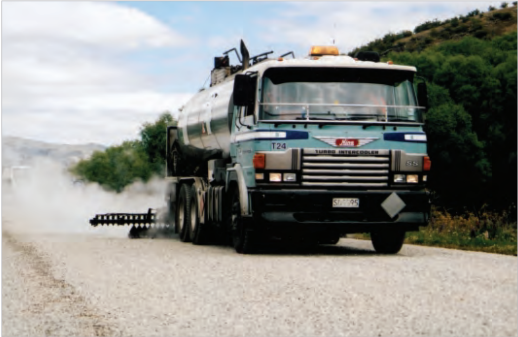
Figure 10-17 A bitumen distributor in action.
