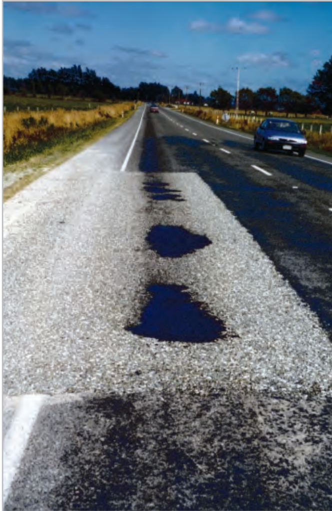
Figure 4-18 A flushed and tracked repair patch.
