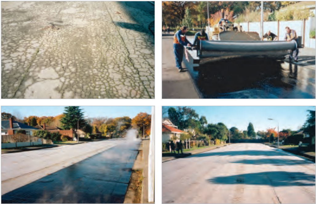
Figure 3-26 Laying a geotextile on a cracked surface.
