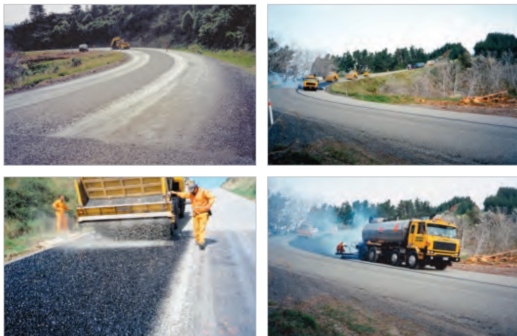
Figure 3-16 A sandwich seal under construction in Hawke's Bay. Clockwise from top left: Applying the first layer of large chip to the flushed surface without binder. Top right: Applying the binder over the large chip. Bottom right: Applying the binder over the large chip. Bottom left: Small chip being spread over binder over large chip.
