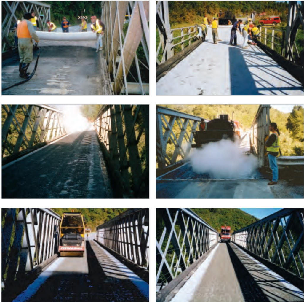
Figure 6-9 A geotextile two coat seal being applied to a single-lane timber bridge (on State Highway 6, West Coast of South Island) to protect joints and metal parts from the effects of water. Clockwise from top left: Laying the geotextile over hand-sprayed tack coat. Top right: Smoothing down the geotextile. Middle right: Spraying the geotextile with the binder. Bottom right: Spreading the chip over the geotextile. Bottom left: Rolling the chip onto the geotextile. Middle left: Spraying the second application of binder over the geotextile and first chip layer. The next step is to apply a second layer of chip.
