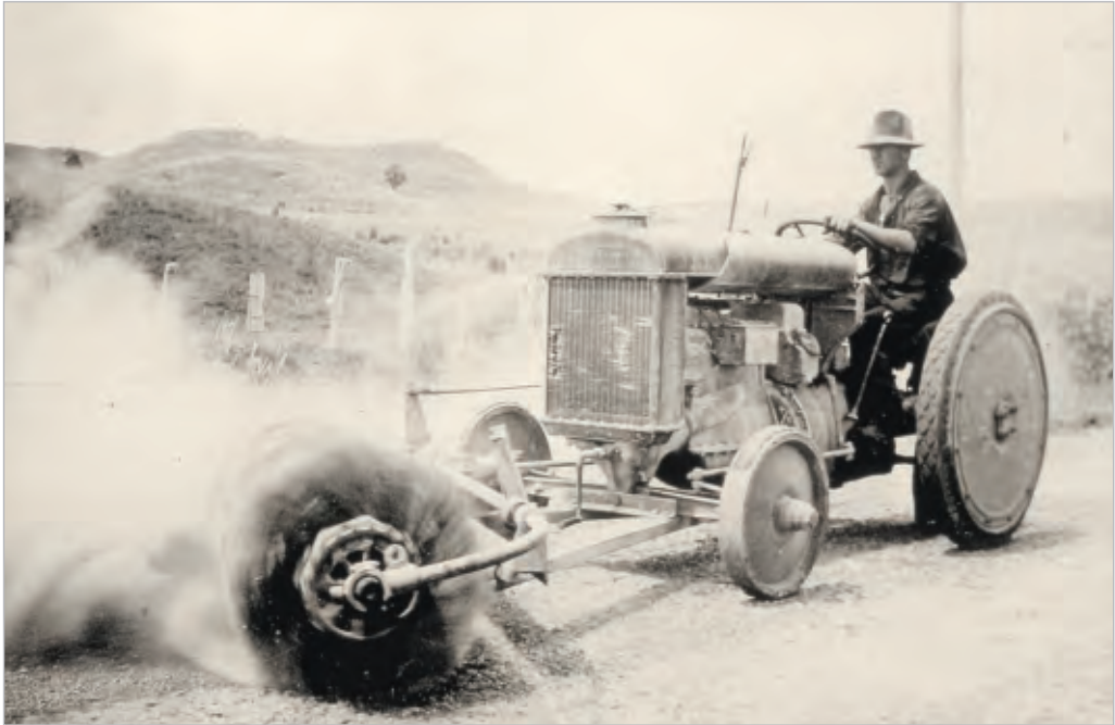
Figure 7-1 The basecourse for State Highway 2 in Cook County, Gisborne, was swept clear of loose aggregate and other detritus by this rotary broom mounted in front of a tractor (with solid wheels and tyres), in the 1920s. Photo courtesy of John Matthews, Technix Group Ltd
