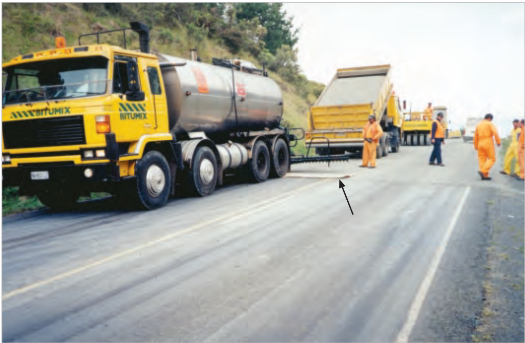
Figure 11-6 A spray run about to start. Note the paper spread in place so that an accurate start line can be achieved.
