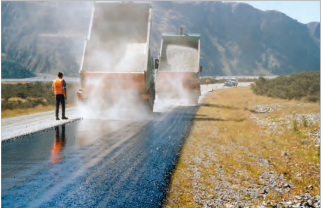
Figure 8-26 Clouds of dust when applying chips may indicate that they have low cleanness value.
