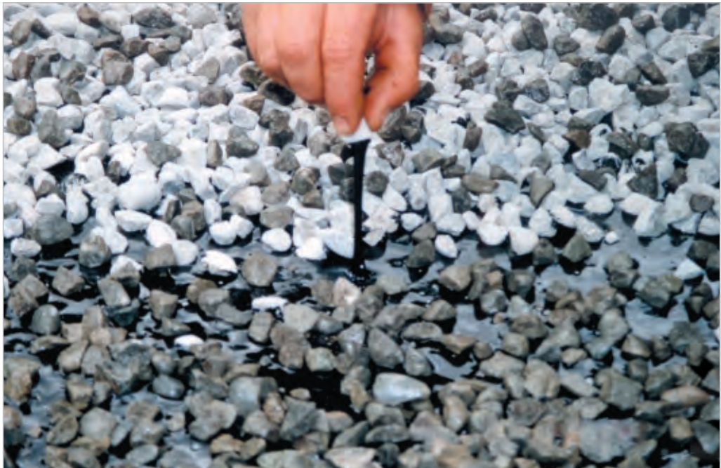
Figure 8-19 Removing a chip from a PMB chipseal reveals a long string of binder with enhanced elasticity. Photo courtesy of Les McKenzie, Opus
