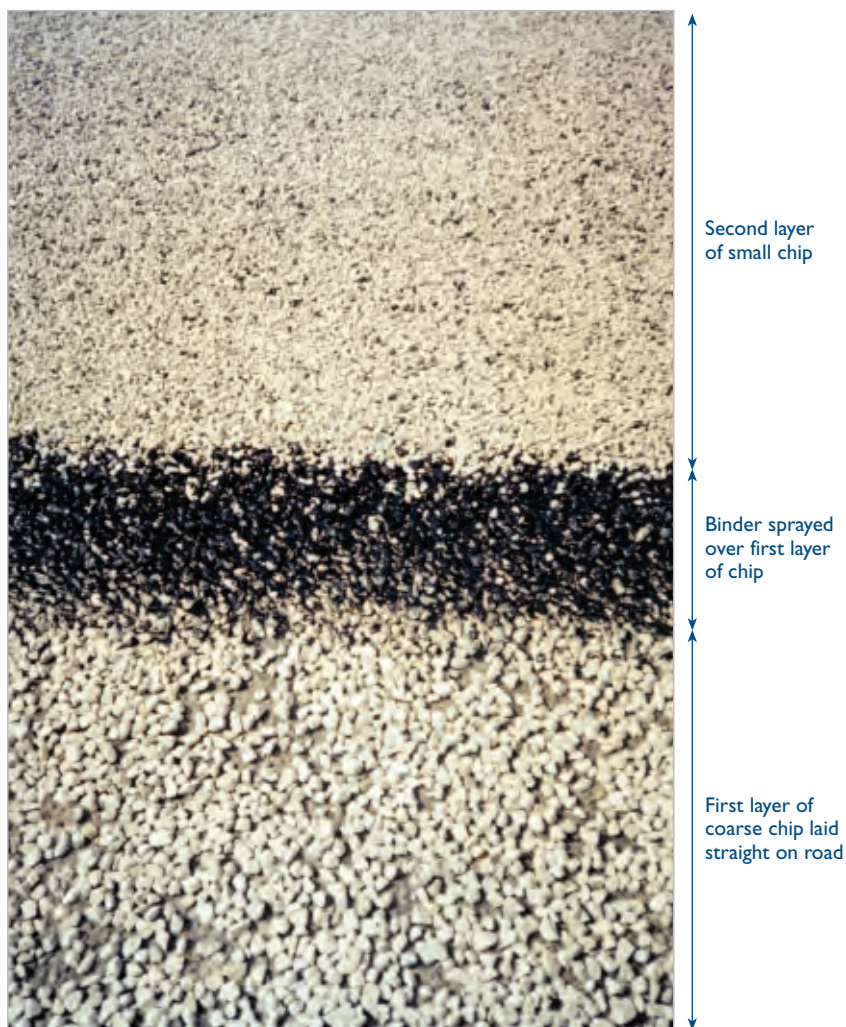
Figure 12-8 The three layers of a sandwich seal are shown part way through construction.
