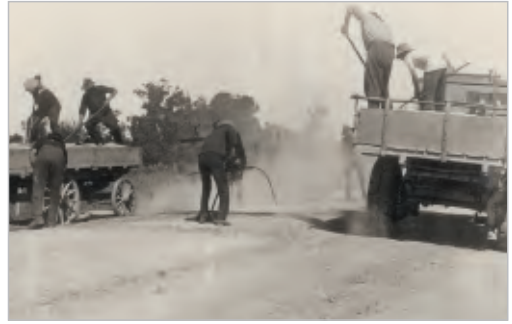
Figure 3-6 Constructing a first coat chipseal near Gisborne in the 1920s was not highly mechanised, compared to the line of construction machines used in the 2000s shown in Figure 3-7. Left: Hand spraying the basecourse, from the tractor-drawn bitumen distributor. Right: Spreading the chip by shovel as the tip truck was not yet in use. Photos courtesy of John Matthews, Technix Group Ltd
