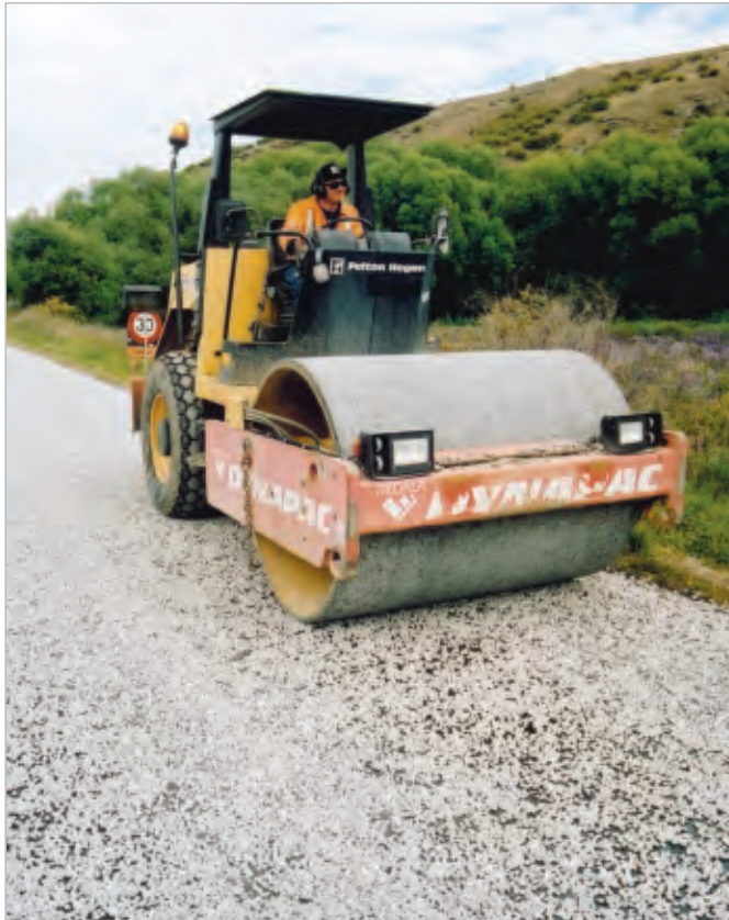
Figure 10-24 The two axles of a combination roller showing the different rollers.
