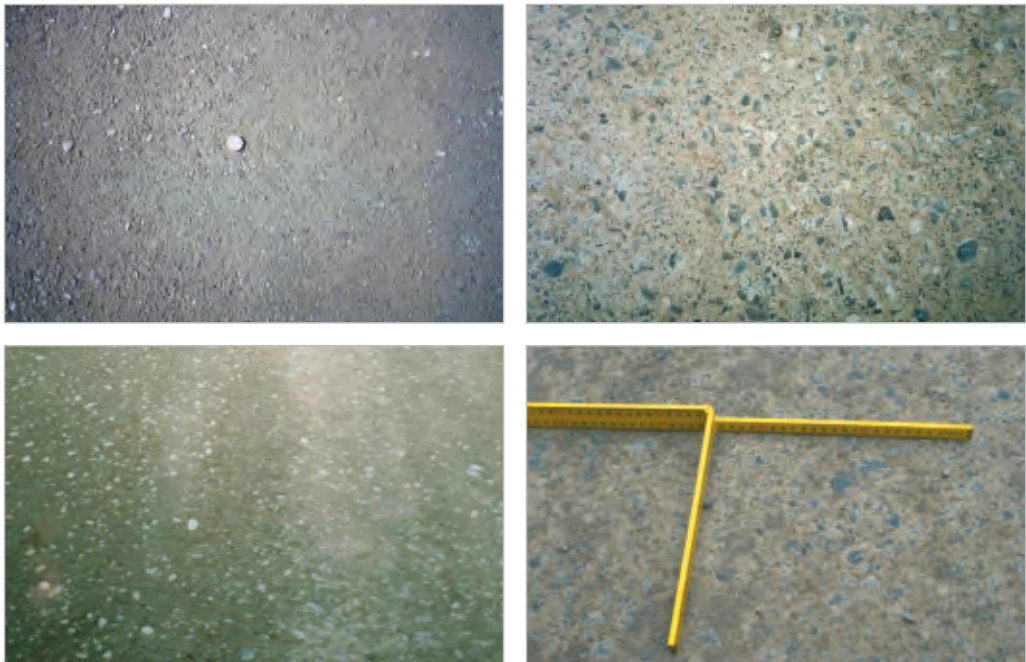
Figure 7-3 Basecourses prepared for first coat sealing from aggregates that are characteristic of different parts of New Zealand, after they have been prepared by sweeping.
