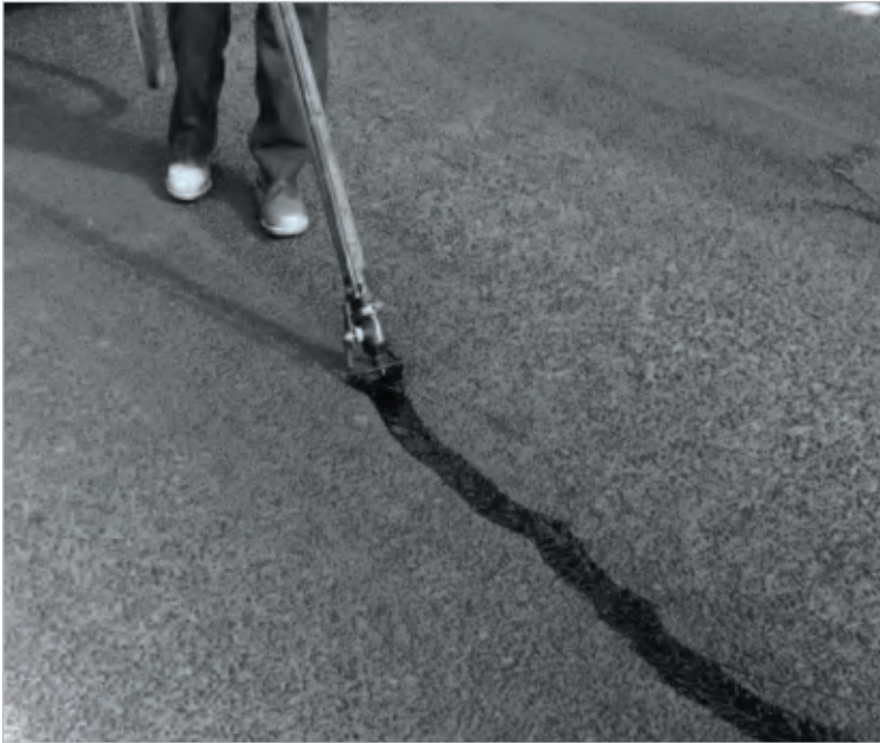
Figure 7-5 Filling a large joint crack using the bandage technique.
