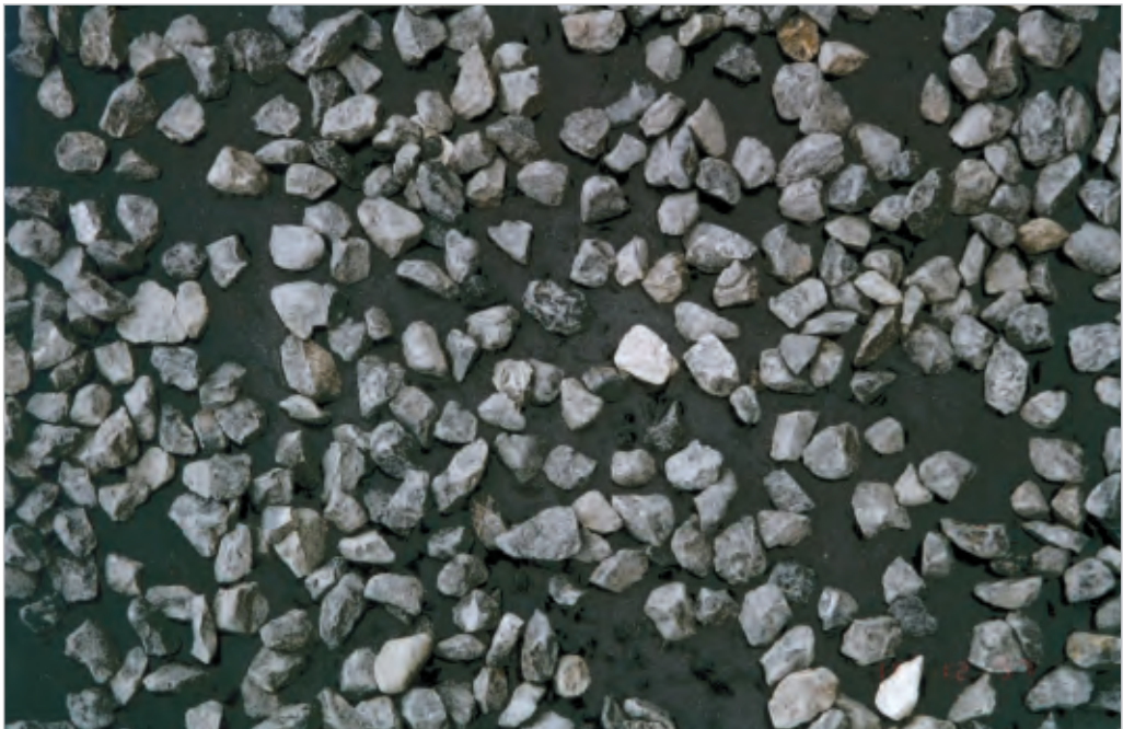
Figure 11-4 Now advice is to aim for a chip spread-target rate as shown at the top of this page. This was previously considered as under-chipped. The image at the bottom of this page shows a chip spread rate suitable for use in the first layer of a racked-in chipseal. Note the large 'windows' where smaller chip in the second layer can adhere to the binder. Photos courtesy of Shirley Potter and Les McKenzie, Opus
