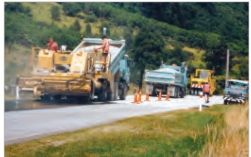
Figure 3-7 Constructing a chipseal. Clockwise from top left: Spraying binder and spreading chips in one operation. Top right: Spraying the binder. Bottom right: Spreading the chips. Bottom left: Rolling the surface. Photos courtesy of Les McKenzie, Opus
