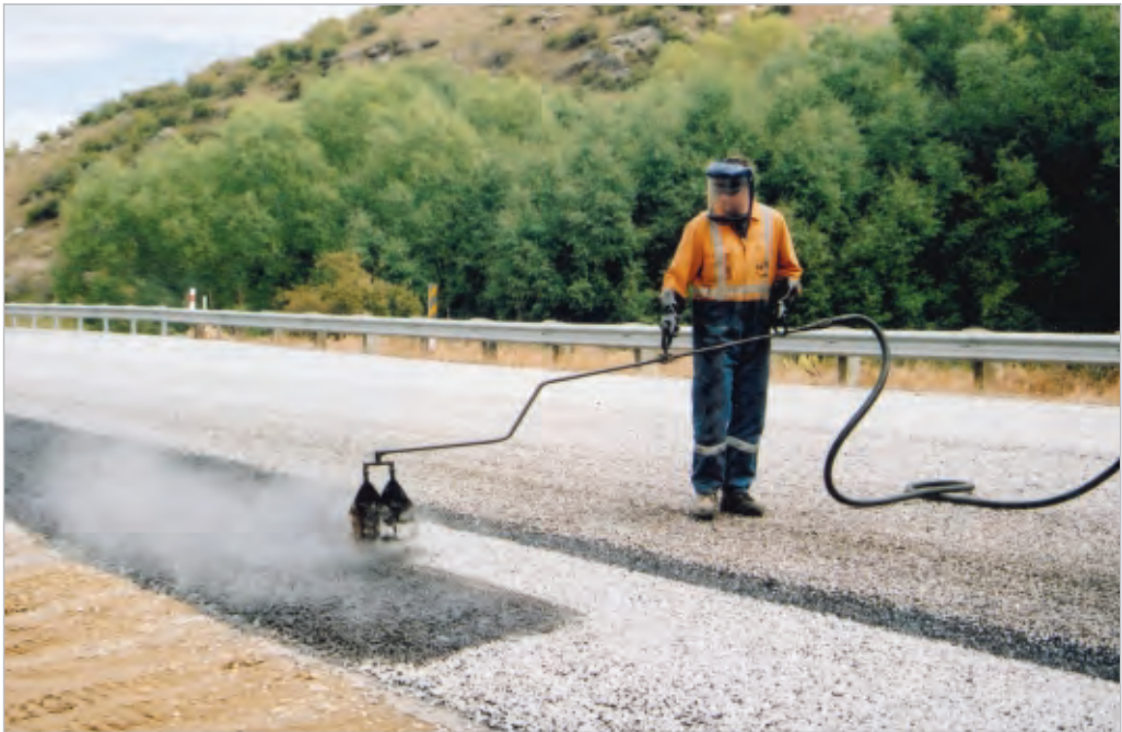
Figure 10-11 Hand spraying an extra width near a side road.
