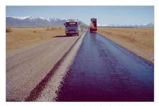
To cope with the extreme climate experienced in the Mackenzie Basin, South Island, a two coat seal is used on State Highway 80 (with Aoraki/Mount Cook and the Southern Alps in the far distance). Each step of the process is visible: in the centre of the road is a narrow strip of the first layer of bitumen, to its right are the first layer of chips, and then the second layer of bitumen. The second layer of chips is in the process of being spread.
