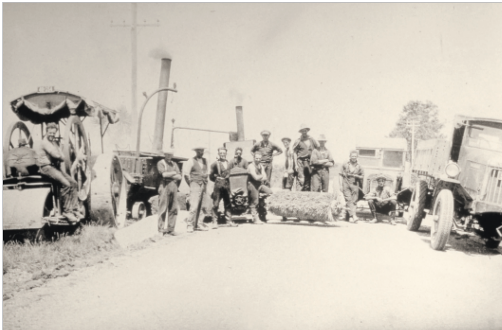
Figure 11-1 A 1920s road sealing team ready for work, with their steam roller, the tar kettle stoked up with the distributor nearby, rotary broom, and chip spreading trucks, in Cook County, Gisborne.
