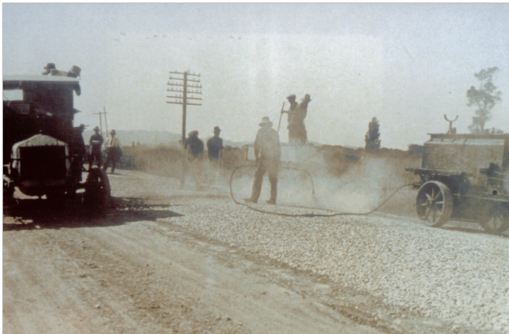
Figure 11-7 In the 1920s, hand spraying was the only way to get the binder onto the road. It required highly developed skills to apply the binder evenly over the surface.
