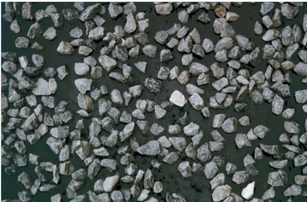
Figure 11-4 Now advice is to aim for a chip spread-target rate as shown at the top of this page. This was previously considered as under-chipped. The image at the bottom of this page shows a chip spread rate suitable for use in the first layer of a racked-in chipseal. Note the large 'windows' where smaller chip in the second layer can adhere to the binder. Photos courtesy of Shirley Potter and Les McKenzie, Opus
